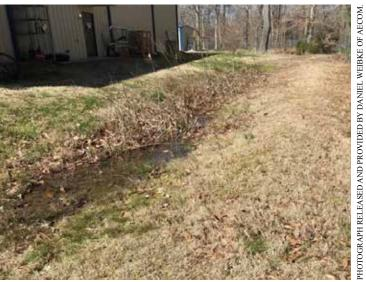
Operational issues, like the clogged media caused by prolonged ponding shown here, can be prevented or resolved through routine maintenance and inspection.
