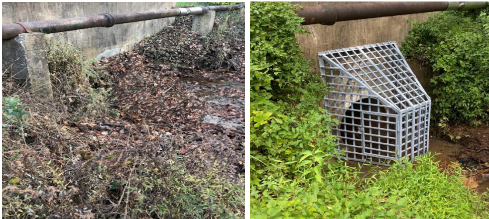
(Left) Excessive debris covers the trash screen and impedes water flow causing flooding during heavy rain events. (Right) The same location after removal of excessive debris and sediment and replacement of trash screen with a larger model.
