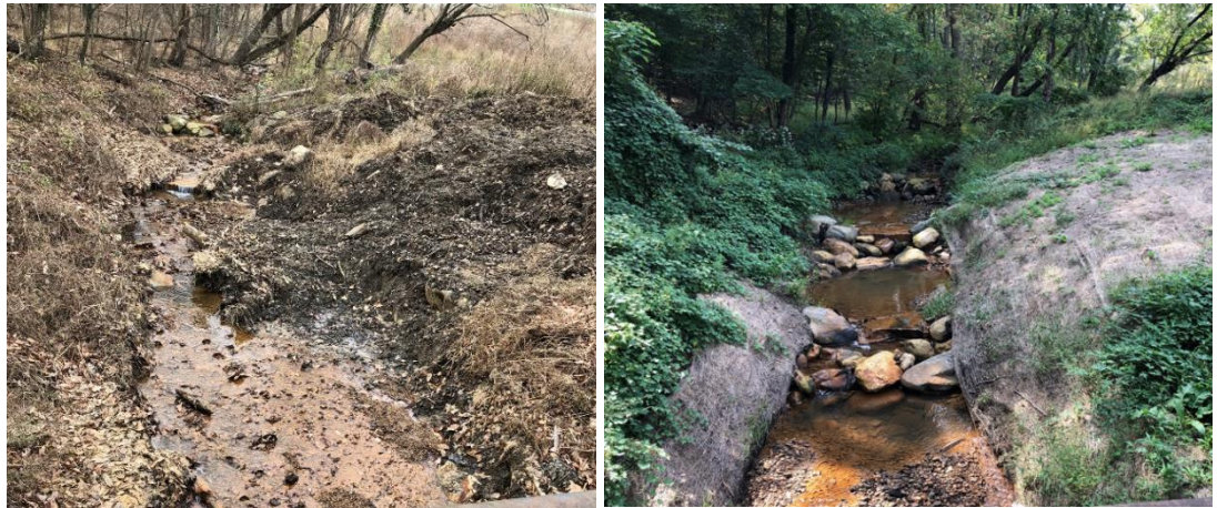
(Left) Excess sediment and debris inhibited stream flow, and lack of bank stabilization allowed for erosion upstream of the trash screen at Ord & Weitzel Drive. (Right) Removed sediment and debris, reconstructed stream plunge pools, and stabilized stream banks allow improved flow of water.
