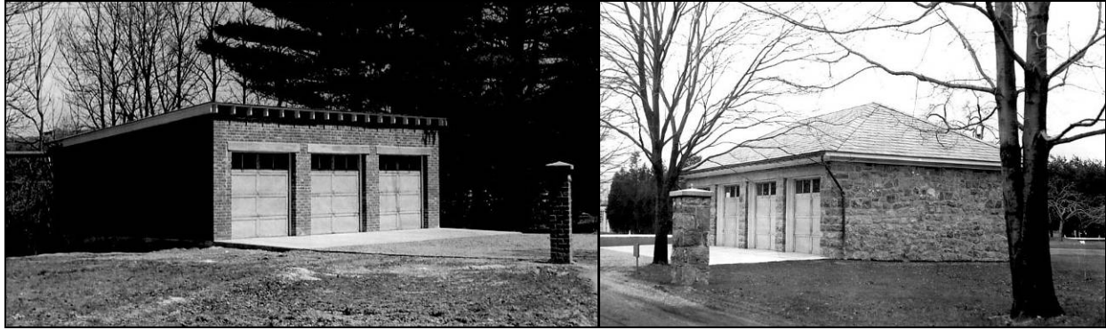
Figure 4-23. Small Garages Constructed at Picatinny Arsenal, New Jersey
