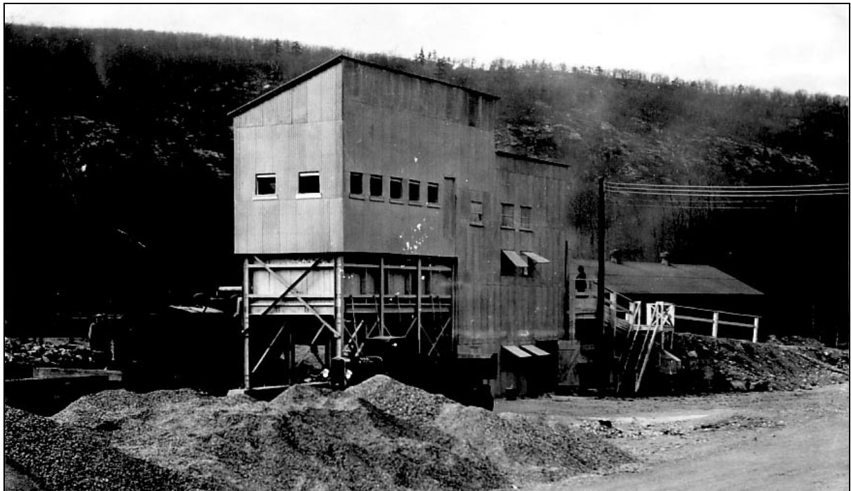
Figure 4-26. Rock Crushing Plant, Picatinny Arsenal, New Jersey.
