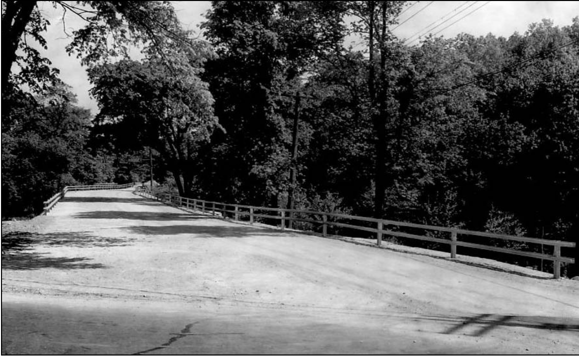
Figure 4-27. New Entrance, Picatinny Arsenal, New Jersey.
