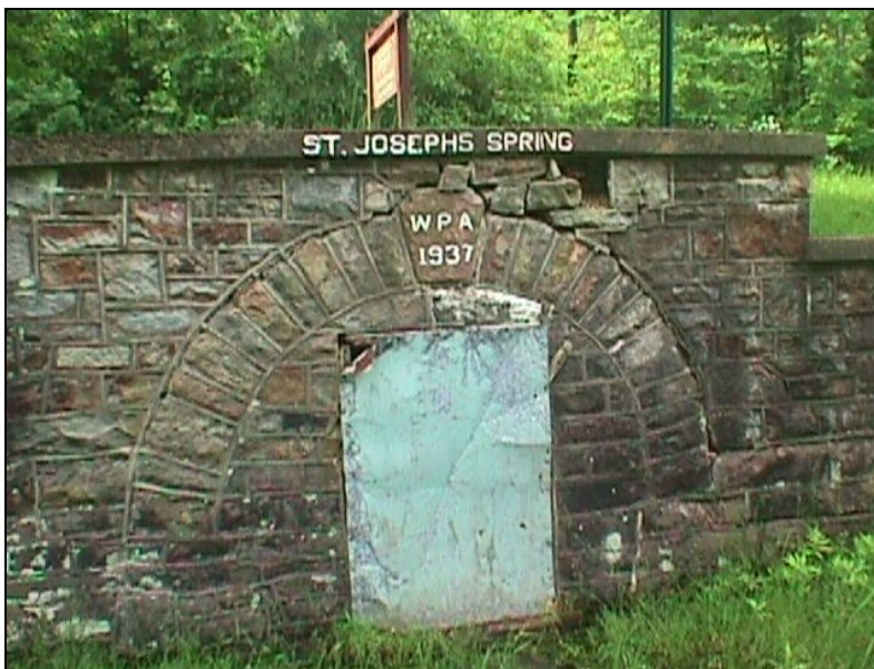
Figure 4-33. Stone Wall Along St. Joseph's Spring, Fort Indiantown Gap, Pennsylvania.
