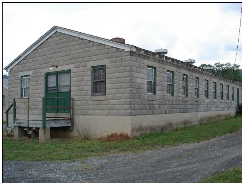
Figure 4-30. Concrete Block Mess Hall, Area 13, Fort Indiantown Gap, Pennsylvania.
