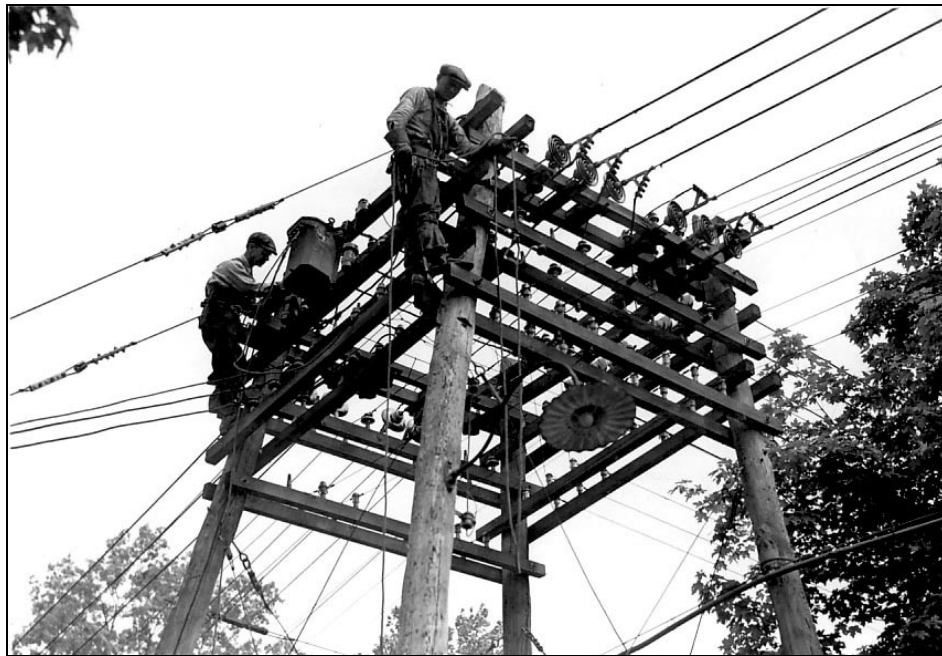
Figure 4-28. Installation of Electric Lines, Picatinny Arsenal, New Jersey.
