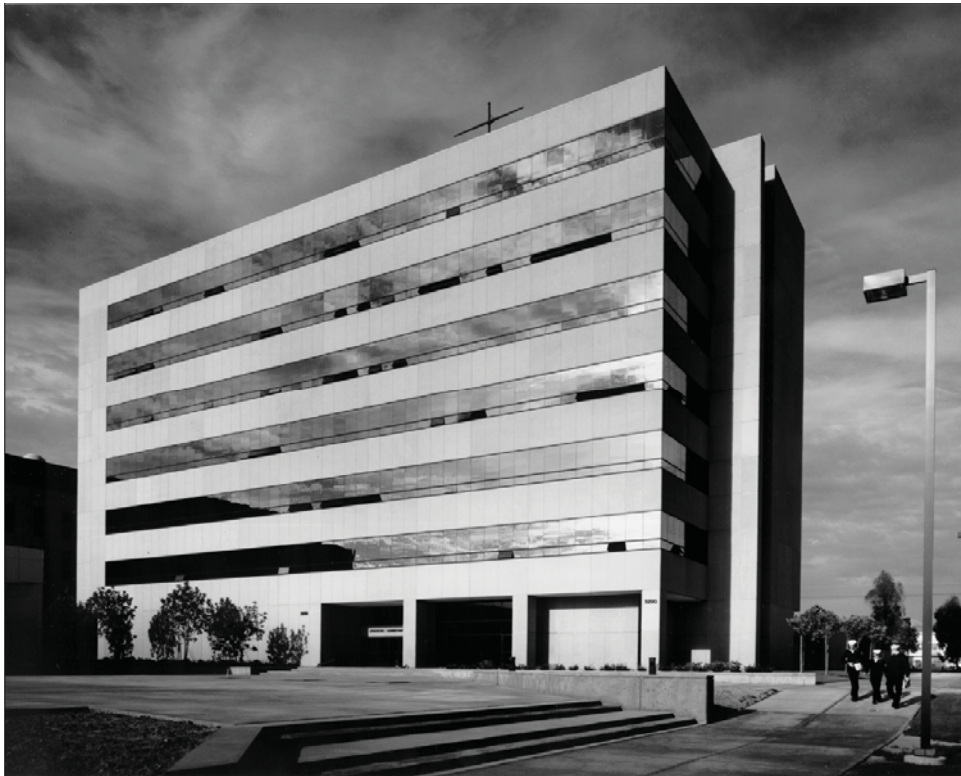
Operations/Administration Complex, Fleet Training Center, NS San Diego, CA, ca. 1985 (courtesy of Kelly Michajlenko, MDWF).
