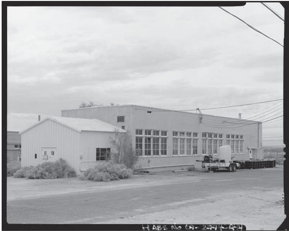
Maintenance Shop, NAWS China Lake, CA (HABS No. CA-2274-A-4).
