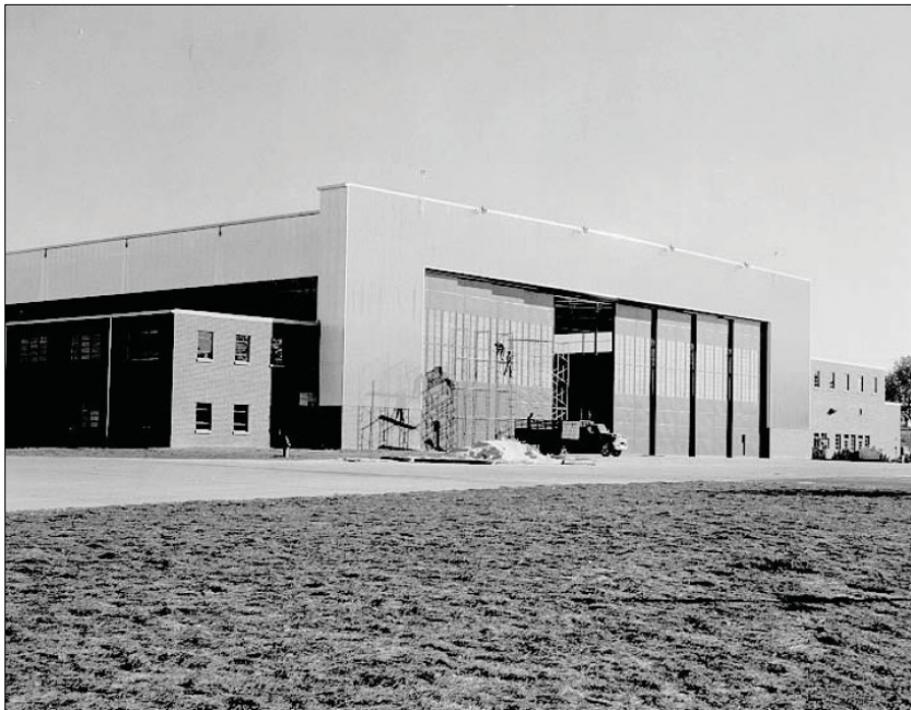
Facility No. 0001, Hangar, NAS Atlanta, GA, 1957 (Hardy, Heck, Moore & Myers, 2000).
