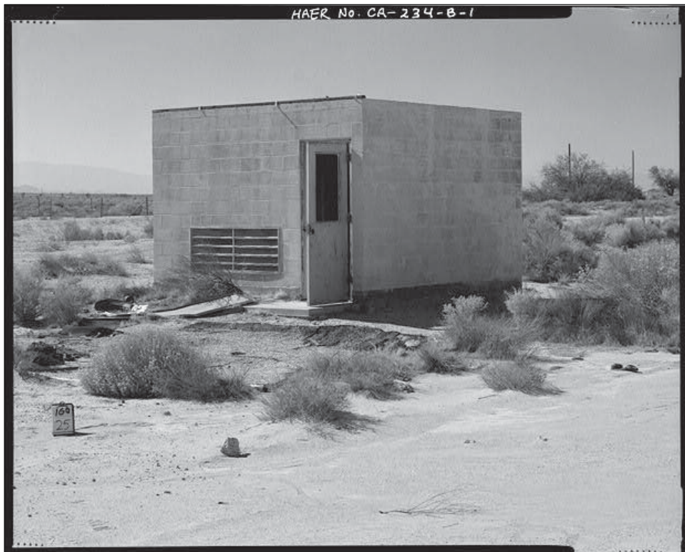
Air Supply Bldg. for Bldg. 545, Edwards AFB, CA (HAER No. CA-234-B-1).
