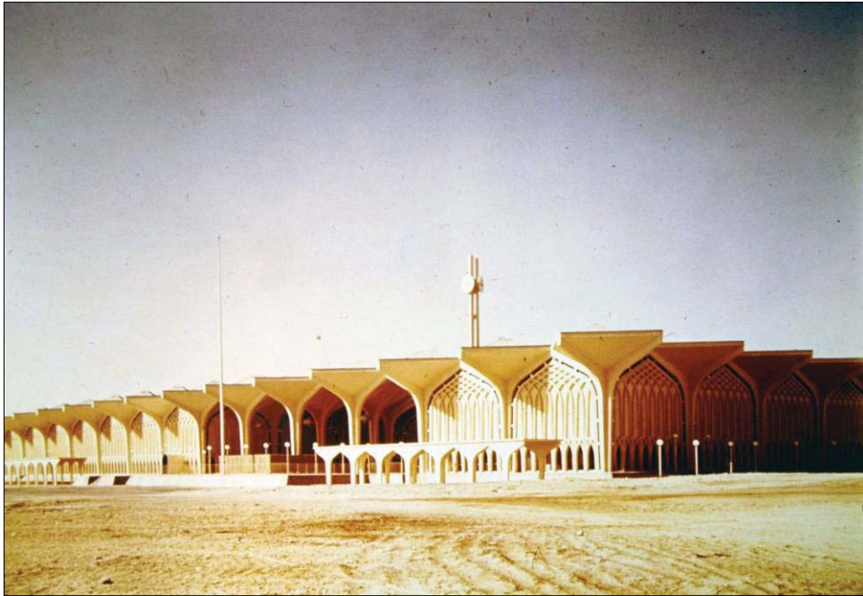
Dhahran Civilian Airport Terminal, Saudi Arabia (U.S. Army Corps of Engineers Archives, Ft. Belvoir, VA, Box 87).
