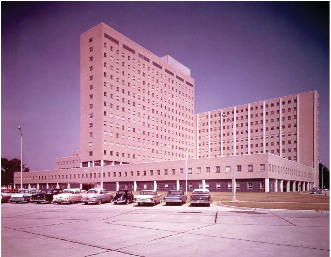
Naval Hospital Portsmouth, VA, ca. 1954 (courtesy of Amanda Walter, AECOM).
