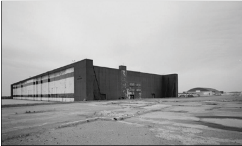
Building No. 8289, Hangar, Loring (Limestone) Air Force Base, ME (Library of Congress, HAER No. ME-64-C).
