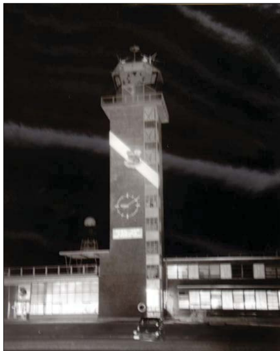
Photo, Control Tower, Loring (Limestone) Air Force Base, Limestone, ME, 1963 (National Archives II, College Park, MD).
