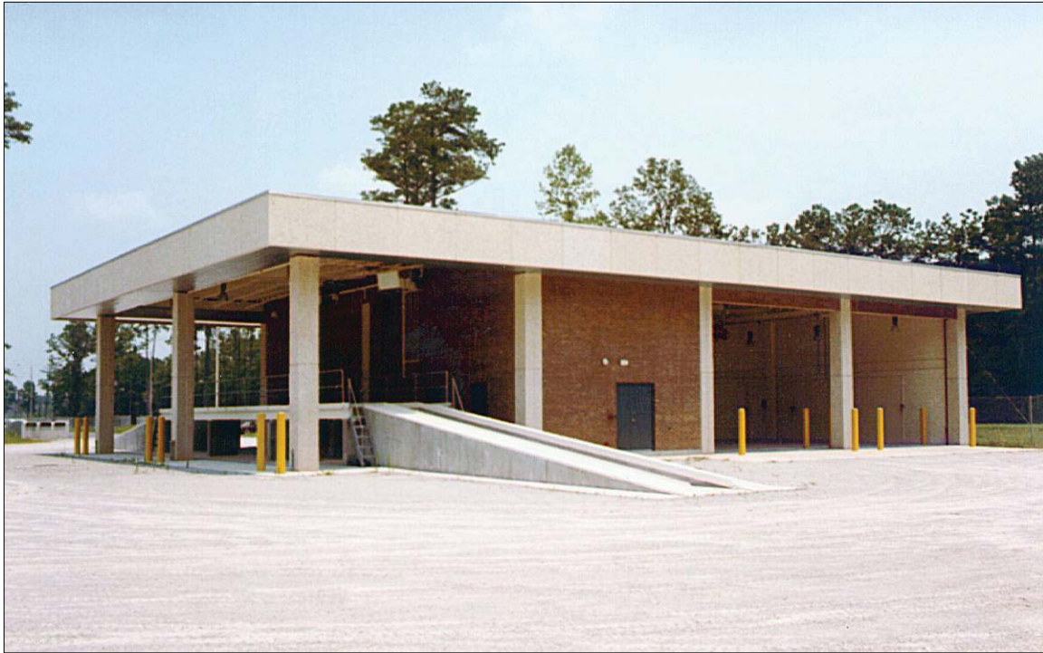
Operation & Maintenance Facility, Camp Lejeune, NC, ca. 1982 (photo by J. N. Pease Associates, courtesy of Angela Mellow, Pease Associates).
