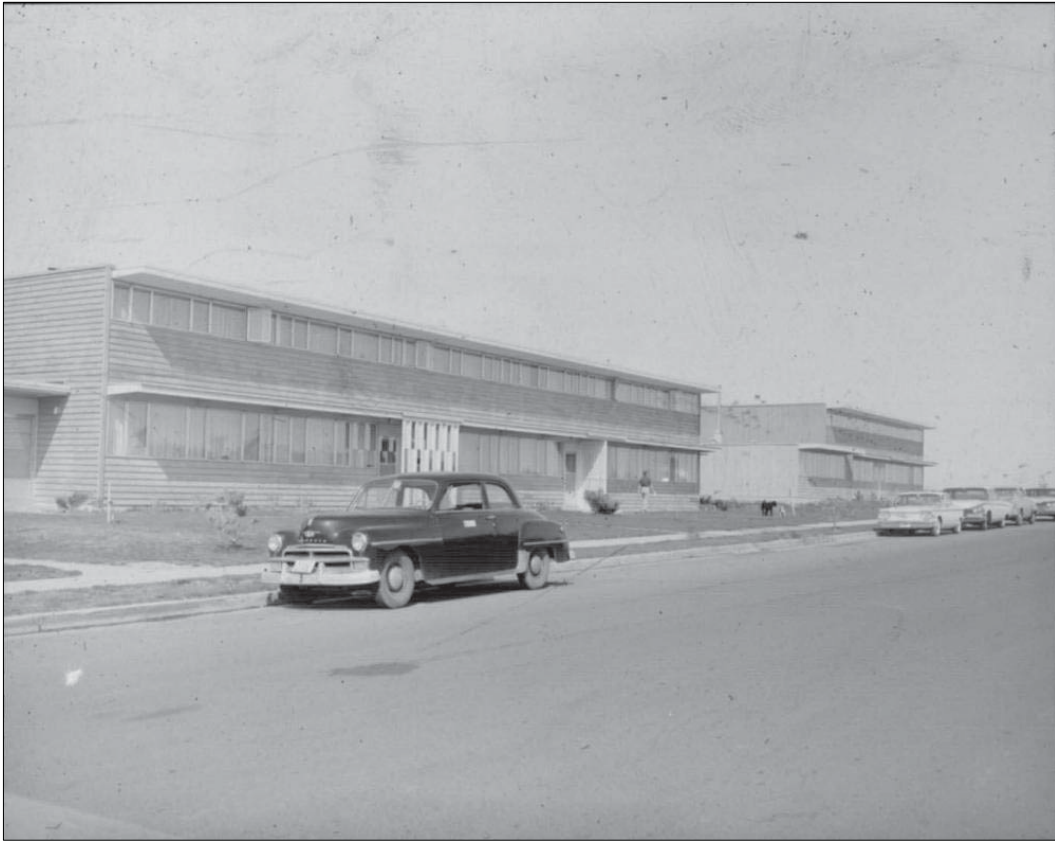
Wherry Housing, Mountain Home AFB, ID, ca. 1958 (courtesy of Mountain Home AFB).
