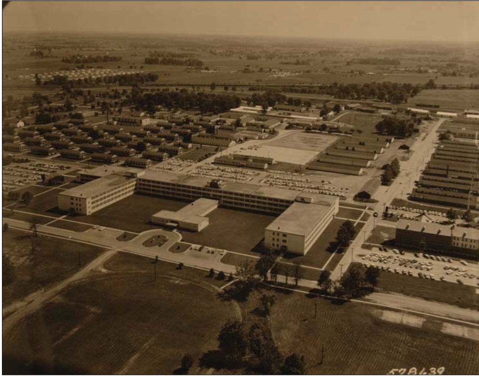
Army Finance Center, Fort Benjamin Harrison, Indianapolis, IN, 1960 (National Archives II, College Park, MD).
