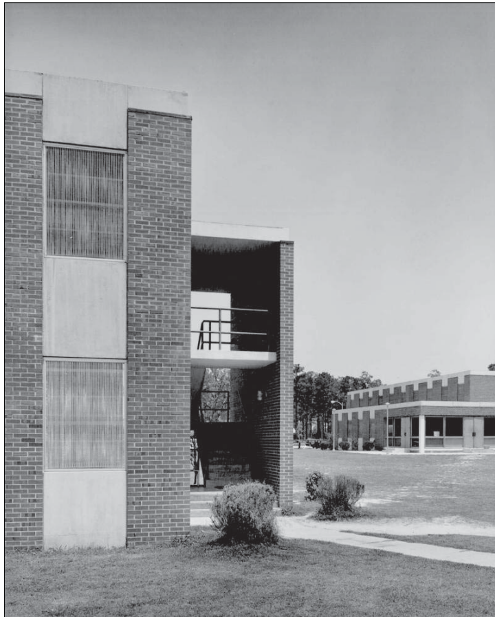
Barracks, Force Troops Complex, Camp Lejeune, NC, ca. 1970 (photo by Gordon H. Schenck, Jr., courtesy of Angela Mellow, Pease Associates).
