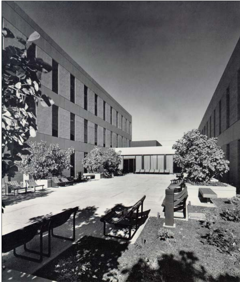
Propulsion Engineering & Applied Instruction Building, P-005/P-008, Fleet Training Center, NS San Diego, CA, ca. 1980 (courtesy of Kelly Michajlenko, MDWF).
