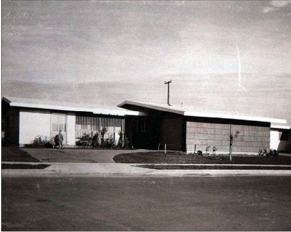
Capehart Housing, Vandenberg AFB, CA, ca. 1956 (National Archives II, College Park, MD).
