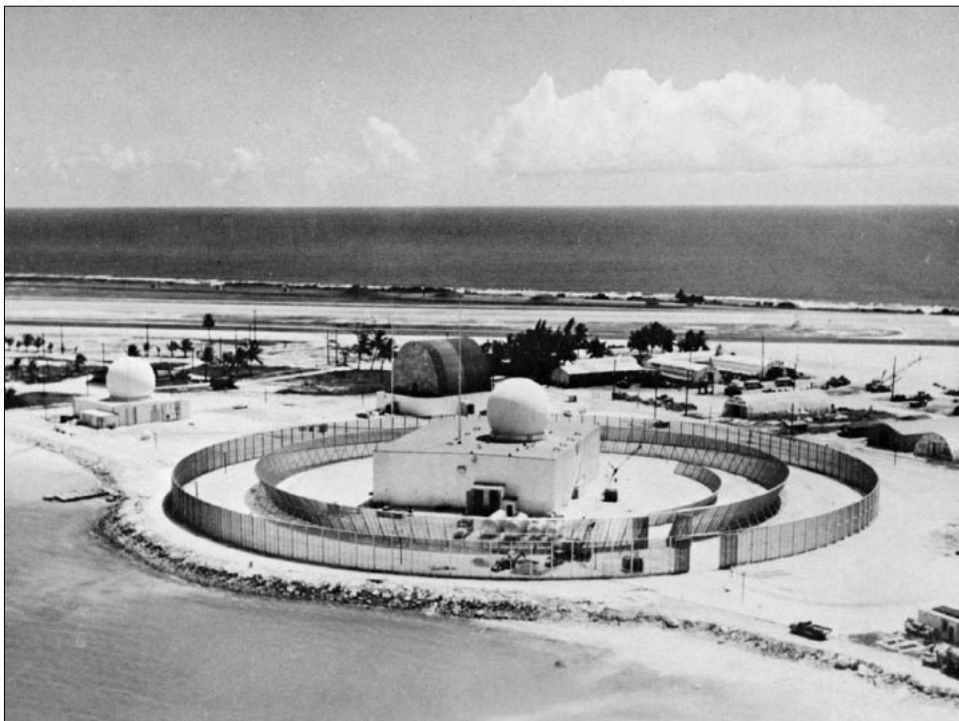
Prototype "Hard" Nike-Zeus Anti-missile System Facilities, Kwajalein Atoll (Breuer, Against All Odds).
