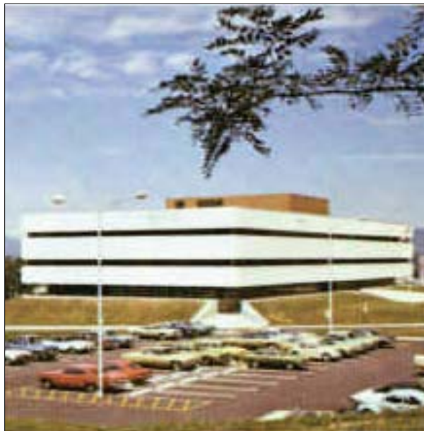
Consolidated Administration Building, Radford Army Ammunition Plant, Radford, VA (U.S. Army Corps of Engineers Distinguished Design Awards, 1976).
