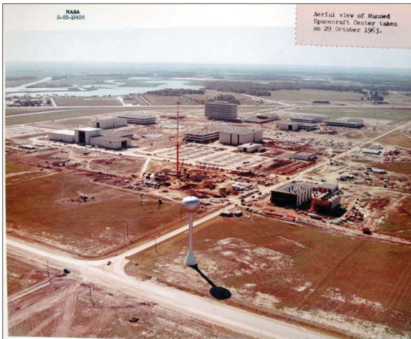
Manned Spacecraft Center, Houston, TX (U.S. Army Corps of Engineers Archives, Ft. Belvoir, VA, Box 97, Folder 7).
