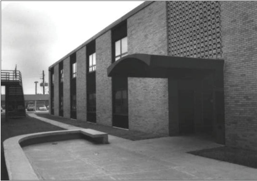
Naval and Marine Corps Reserve Readiness Center, Houston, TX, 1995 (Turner Collie & Braden Inc., 1998).
