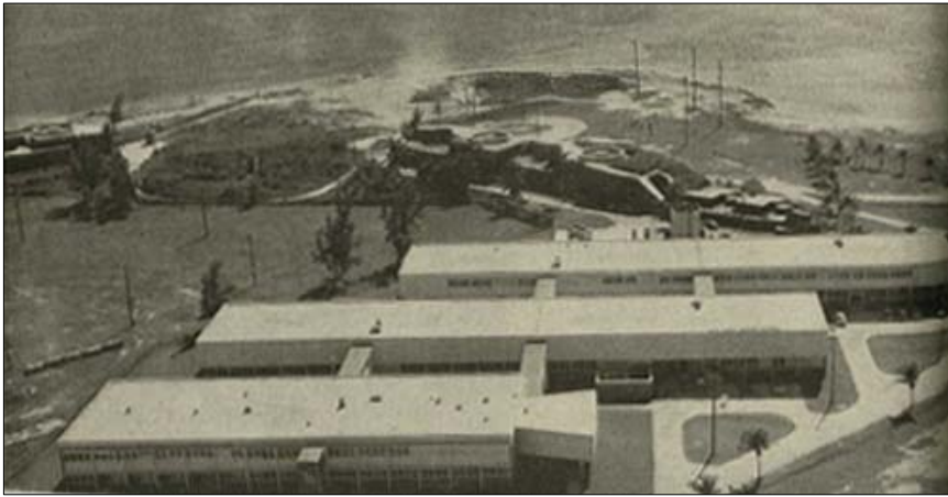
Aerial view of the Fleet Sonar School, Key West, FL (Photo from Architectural Forum, July 1955).
