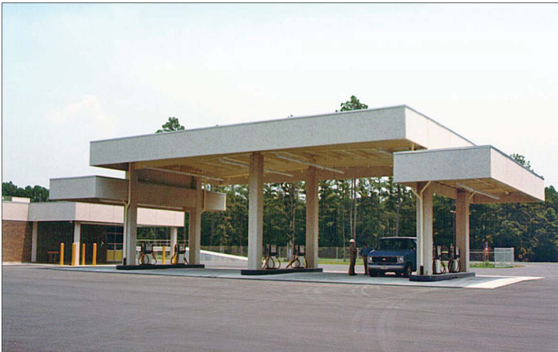
Operation & Maintenance Facility, Camp Lejeune, NC, ca. 1982 (photo by J. N. Pease Associates, courtesy of Angela Mellow, Pease Associates).
