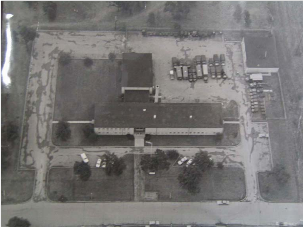
Army Reserve Center, Tonawanda, NY, ca. 1952 (HHM, Inc., 2008).
