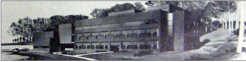
Night Vision Systems Laboratory, Ft. Belvoir, VA (Progressive Architecture, Aug. 1975).
