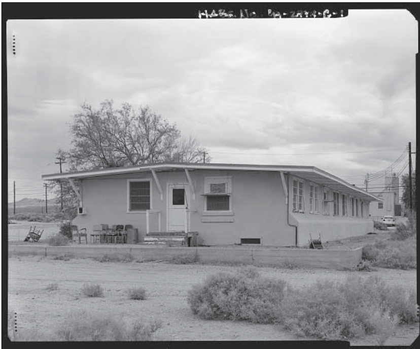
Office, NAWS China Lake, CA (HABS No. CA-2274-C-1).
