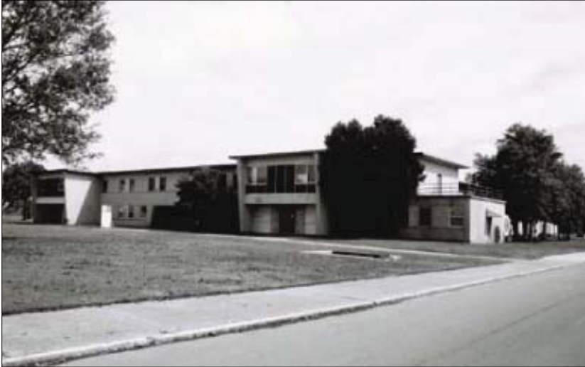
Facility S-328, Barracks for Enlisted Men, NAS Memphis (Integrated Cultural Resource Management Plan and Historical Resource Survey Update, Naval Support Activity Mid-South, 2004).
