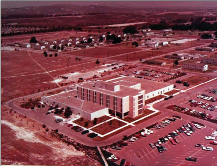
Hospital, Building No. 201, Vandenberg Air Force Base, CA (National Archives II, College Park, MD).
