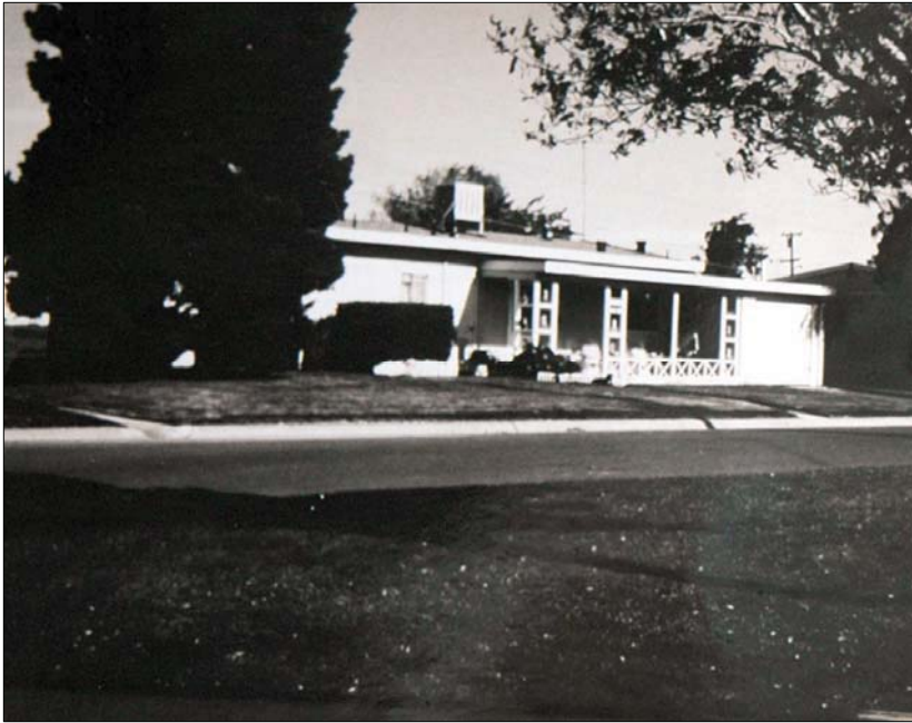
Capehart Housing, Travis AFB, CA, ca. 1960 (National Archives II, College Park, MD).
