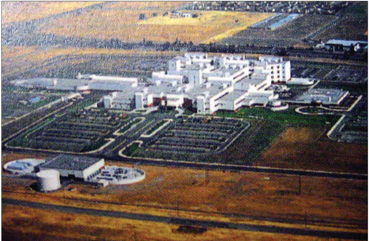
Rendering, David Grant Medical Center, Travis AFB, Fairfield, CA (NBBJ: Selected and Current Works, 1997).
