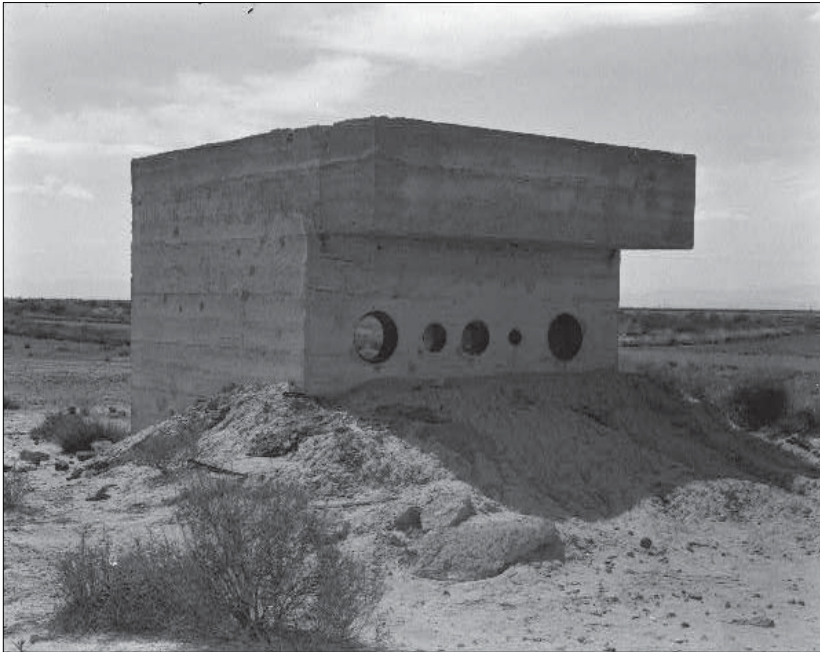
Instrumentation Structure, White Sands Missile Range, NM (HAER No. NM-1A-70).
