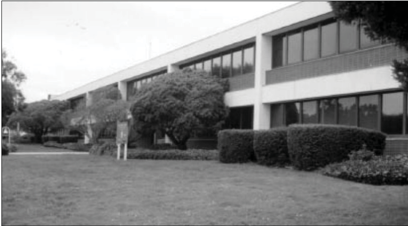
Naval & Marine Corps Readiness Center, San Bruno, CA, 1997 (photo by HHM Inc., courtesy of Turner Collie & Braden Inc., 1998).
