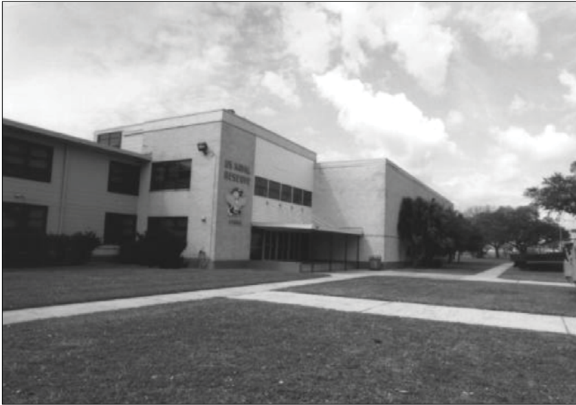
Naval & Marine Corps Reserve Readiness Center, New Orleans, LA, 1995 (Turner Collie & Braden Inc., 1998).
