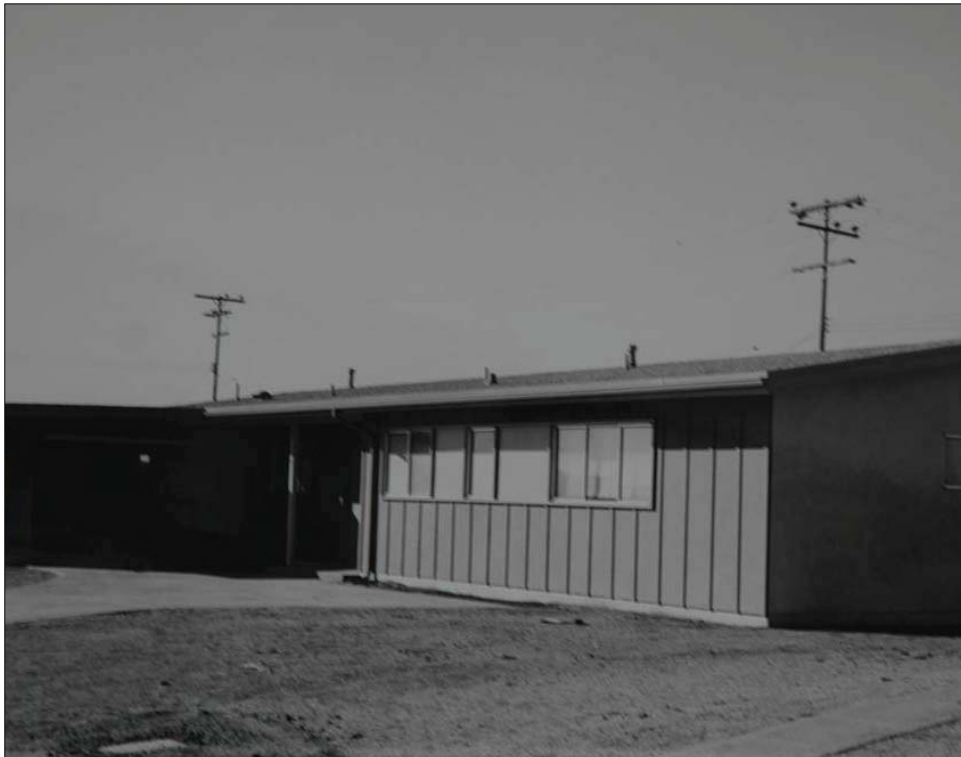
200-man BOQ, Capehart Housing, Mather AFB, Sacramento, CA, 1959 (National Archives II, College Park, MD).
