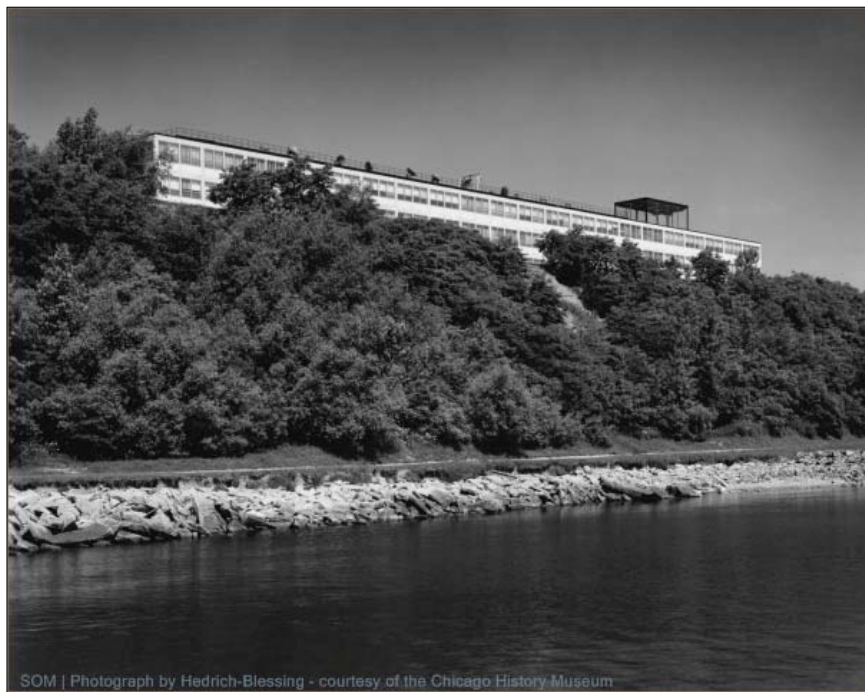
Fire Control, Technicians, Opticalmen, and Instrument School, Naval Station Great Lakes, Chicago, Illinois. Photo from www.som.com (accessed 28 Dec. 2009).
