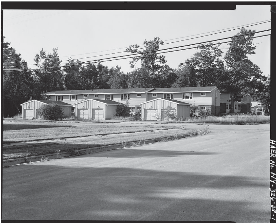
Capehart Four Family Home, Plattsburgh AFB (HAER No. NY-326-DB-1).
