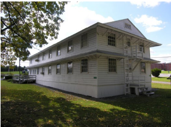
FIGURE 6-56. FORT INDIANTOWN GAP, PENNSYLVANIA ANG. FORMER WORLD WAR II BARRACKS.
