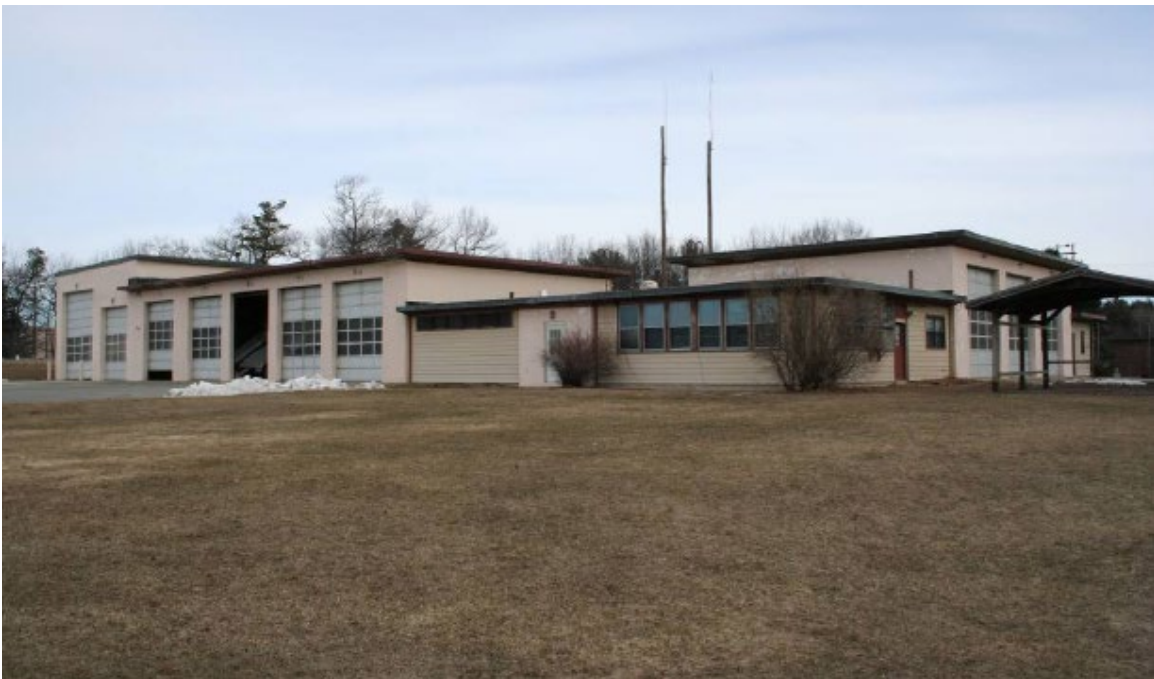
FIGURE 6-36. PEASE INTERNATIONAL TRADEPORT, NEW HAMPSHIRE ANG. COMBINED CRASH AND STRUCTURAL FIRE STATION.
