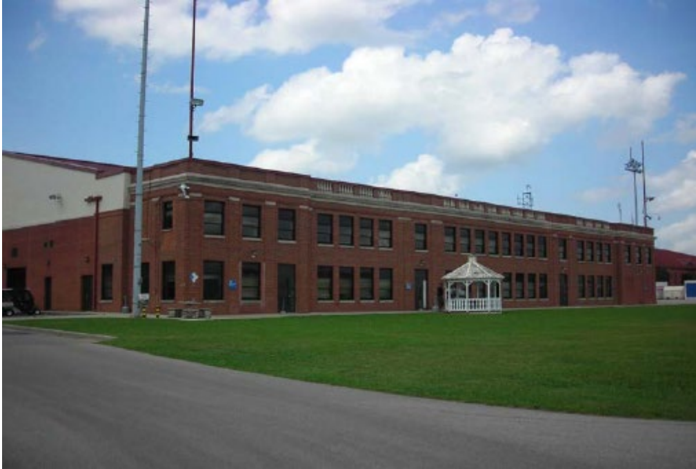
FIGURE 6-2. BIRMINGHAM ANG, ALABAMA ANG, 1937. FORMER HANGAR, DOORS ON BOTH SIDES HAVE BEEN INFILLED.
