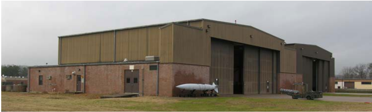
FIGURE 6-11. BRADLEY FIELD, CONNECITCUT ANGB. DOUBLE UNIT HANGAR, 1983.
