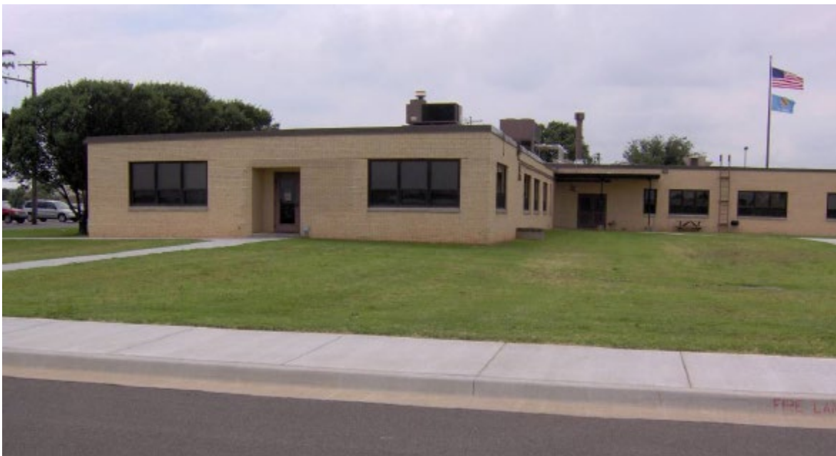
FIGURE 6-47. WILL ROGERS ANGB, OKLAHOMA ANG. WING ADMINISTRATION BUILDING. 1981.
