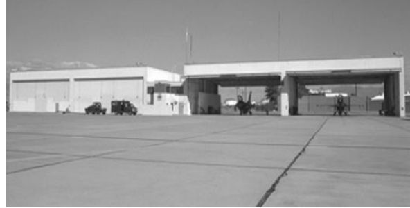
B. SECOND GENERATION ADC ALERT HANGAR, STROBEL & SALZMAN, DAVIS-MONTHAN AFB (FROM USAF 1999A: PLATE 39)
