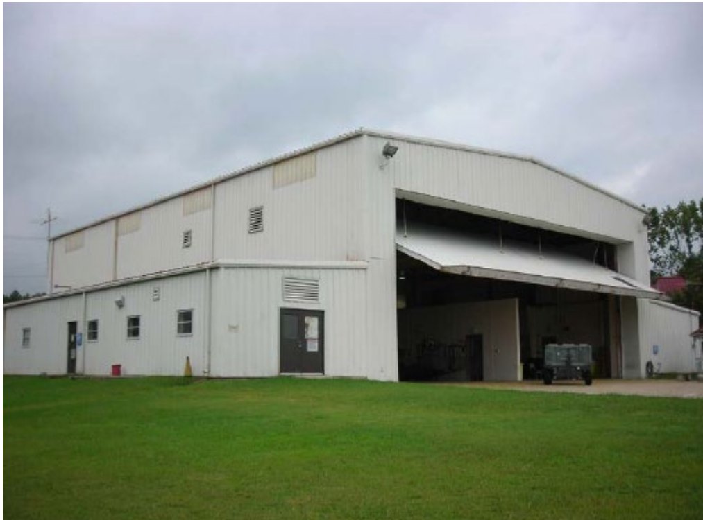
FIGURE 6-20. BIRMINGHAM ANGS, ALABAMA ANG. FORMER FUEL SYSTEMS MAINTENANCE DOCK AND CORROSION CONTROL HANGAR, CURRENTLY ENGINE SHOP.
