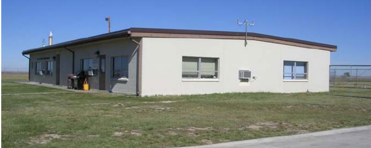
FIGURE 6-35. ALERT CREW QUARTERS, GREAT FALLS INTERNATIONAL AIRPORT ANGB, 1968. BUILDING 44.
