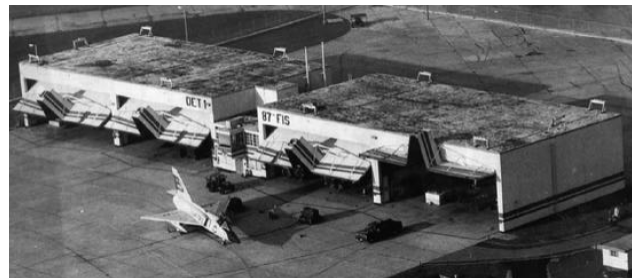
D. FIRST GENERATION ADC ALERT HANGAR, STROBEL & SALZMAN, CHARLESTON AFB (FROM USAF 1999A: PLATE 12).
