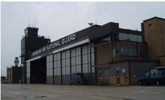
FIGURE 6-3. LAMBERT IAP, MISSOURI ANG. FORMER NAVAL AIR STATION HANGAR, 1942.
