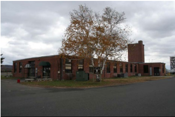
FIGURE 6-59. WESTFIELD-BARNES AIRPORT, MASSACHUSETTS ANG. FORMER DINING HALL, 1950.
