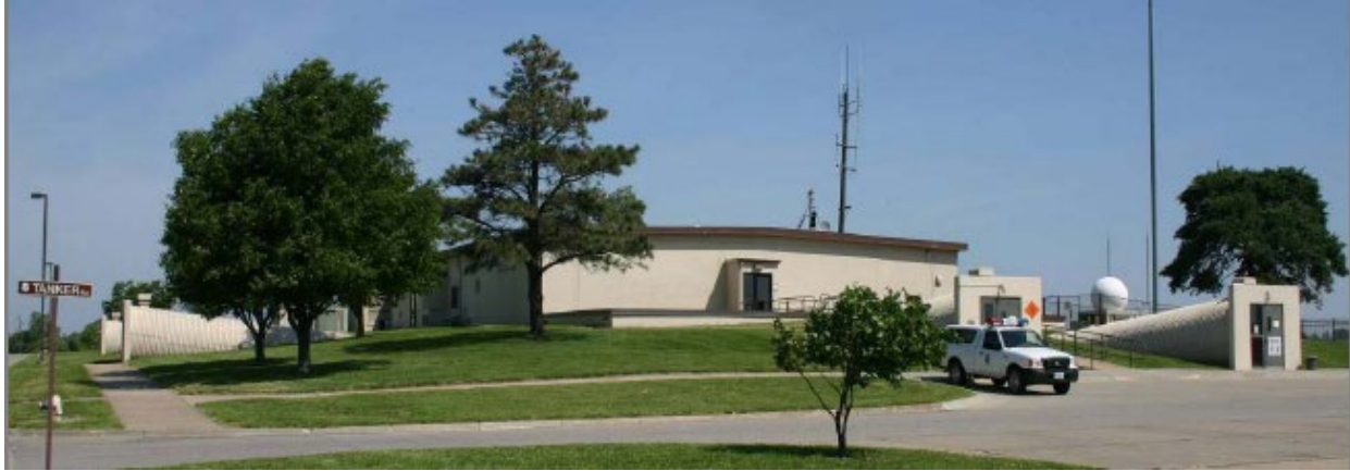
FIGURE 6-33. SAC ALERT READINESS QUARTERS, 150-MAN "MOLEHOLE," FORBES FIELD ANGB, KANSAS, COMPLETED 1960.
