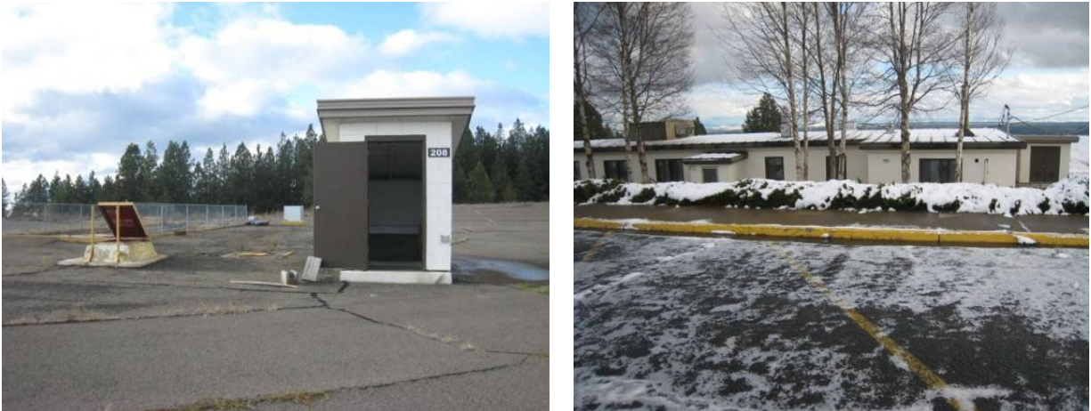
FIGURES 5-8. FOUR LAKES ANG COMMUNICATIONS STATION, WASHINGTON, DECOMMISSIONED LAUNCH AREA (LEFT); ADMINISTRATION AREA (RIGHT)
