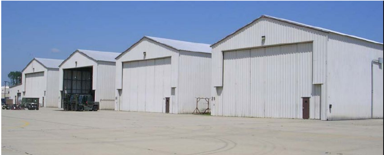
FIGURE 6-31. ALERT SHELTERS, TERRE HAUTE AIRPORT ANGB (HULMAN FIELD), 1966.
