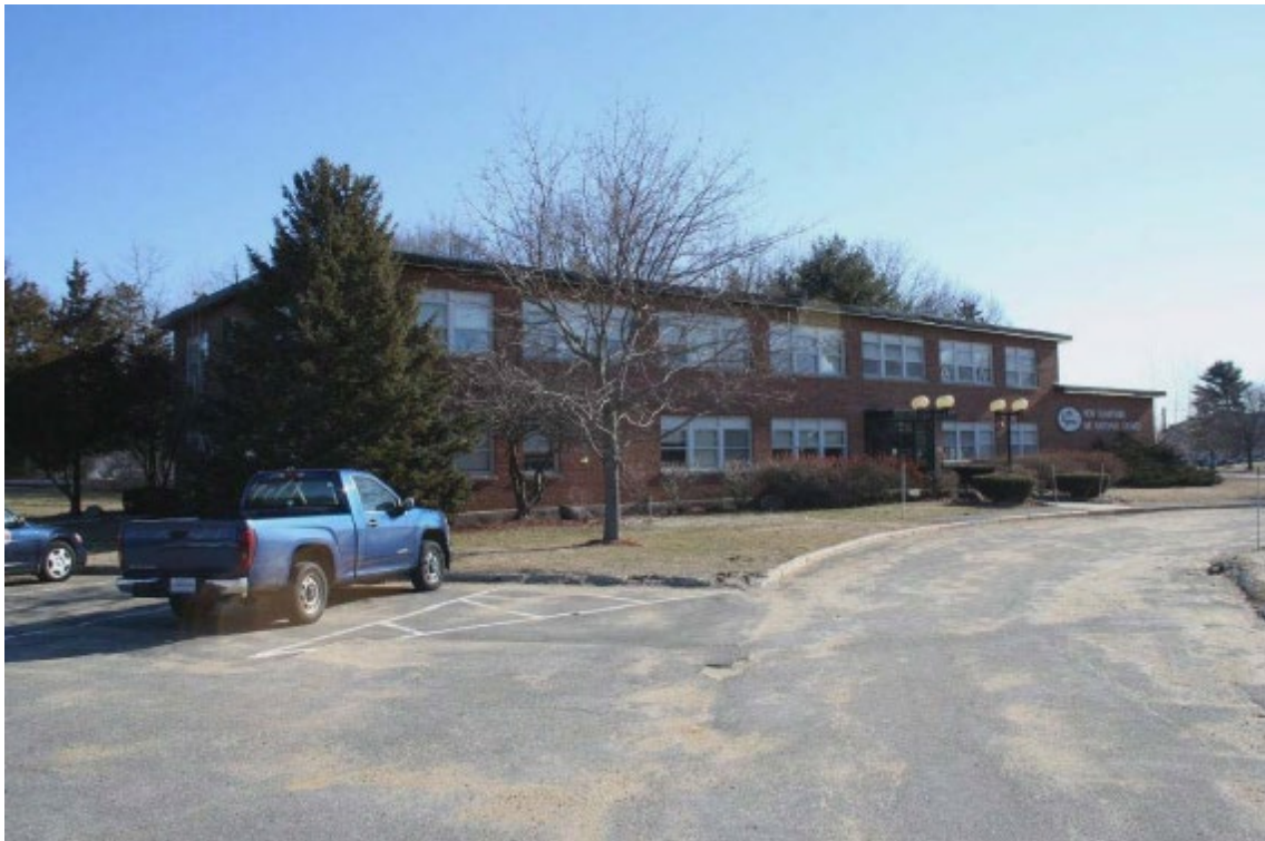
FIGURE 6-45. PEASE INTERNATIONAL TRADEPORT, NEW HAMPSHIRE ANG. ADMINISTRATION BUILDING. 1954.
