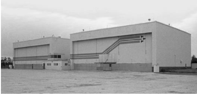
A. SECOND GENERATION ADC ALERT HANGAR, STROBEL & SALZMAN, FORMER LORING AFB (FROM USAF 1999A: PLATE 38).
