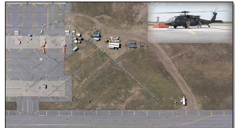
Remedial infrastructure at Airfield's Oasis Fuel Point
