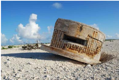
Super typhoon Ioke drove high surf onto Wake Island, tipping a historic pillbox from World War II. Photo by Mark Rauzon
