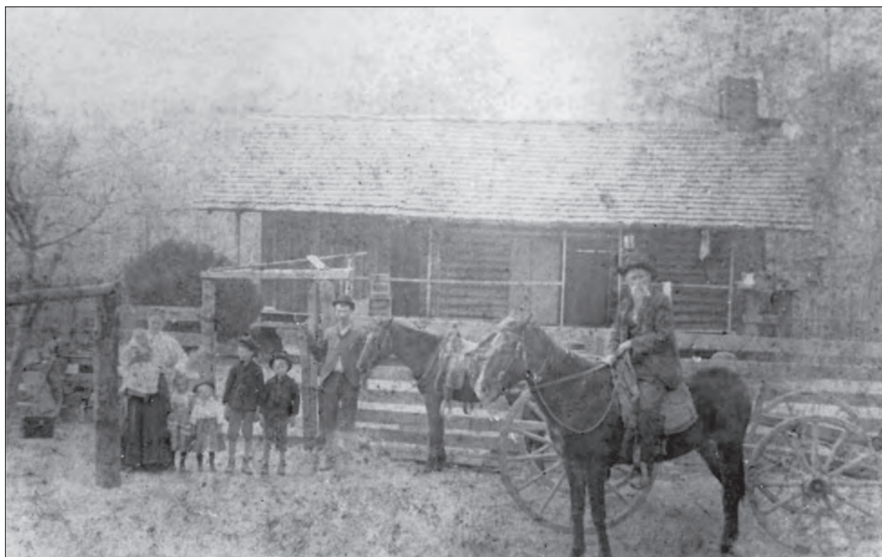
Figure 16 — The first settlers built homes of logs with stick and mud chimneys, like this extended dogtrot cabin (courtesy Museum of West Louisiana).
