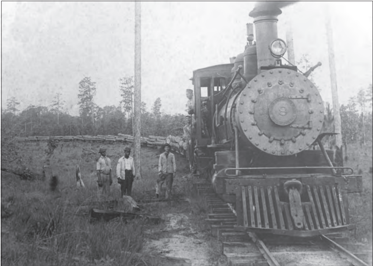
Figure 48— Logging train hauling logs to the mill (courtesy Museum of West Louisiana).
