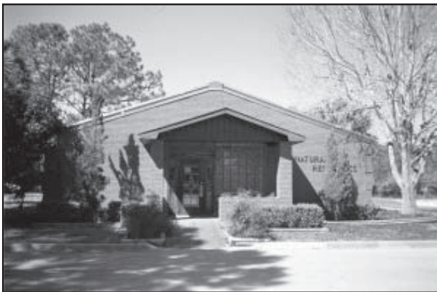
Figure 30. Front entrance of the Natural Resources building.
