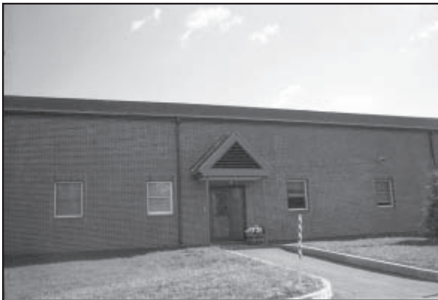
Figure 47. The exterior of Building 12 where the archaeological collection storage area is located.
