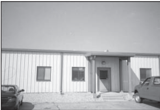
Figure 4. View of Building 1453 showing roof and facade.
