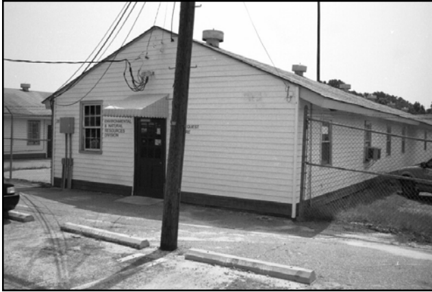
Figure 74. Exterior of the Environmental and Natural Resources Division building.
