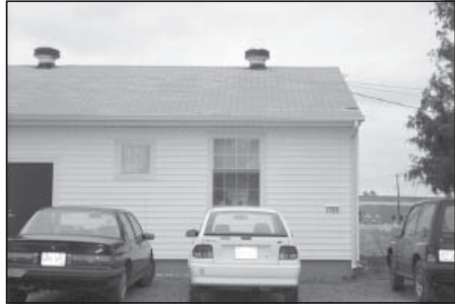
Figure 38. Building 2159 contains all post archaeological collections.
