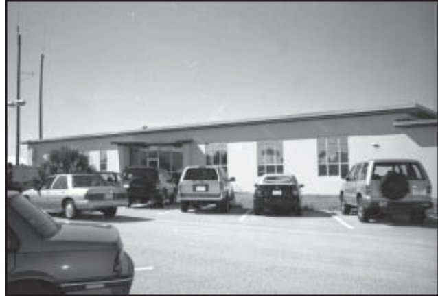
Figure 15. Exterior of Building 1638.
