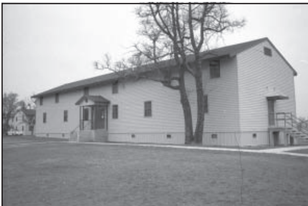
Figure 10. The front of Building 1313.
