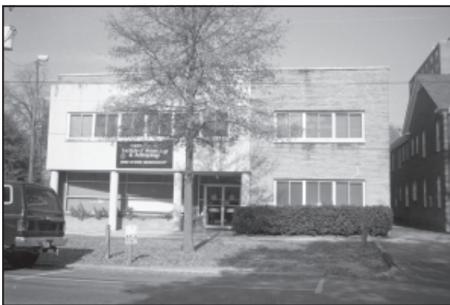
Figure 268. Exterior of the building on Pendleton Street that contains archaeological collections.
