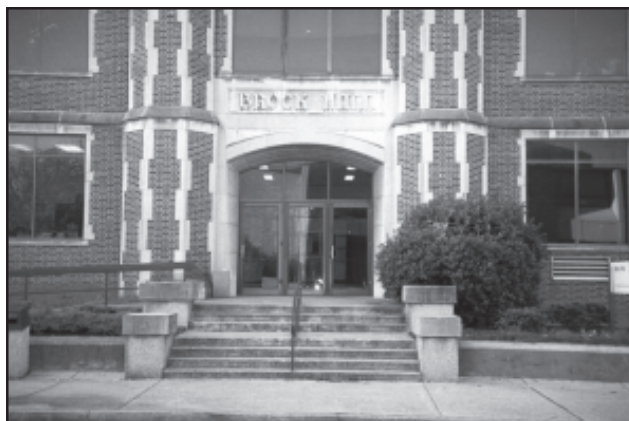
Figure 281. Exterior of Brock Hall where Department of Defense records are stored by the institute.
