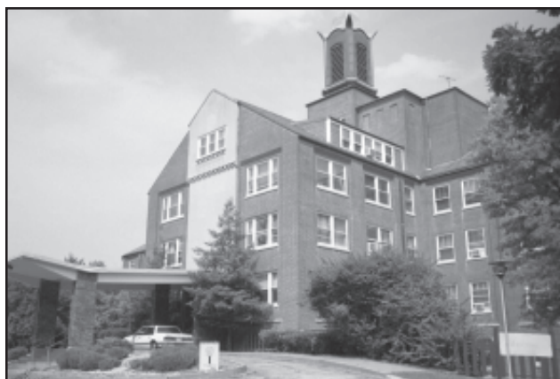
Figure 223. The exterior of the Mt. Providence Building where the archaeological laboratory and storage rooms are located.
