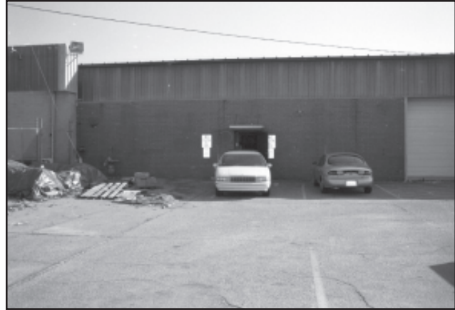
Figure 269. Exterior of the building on College Street.
