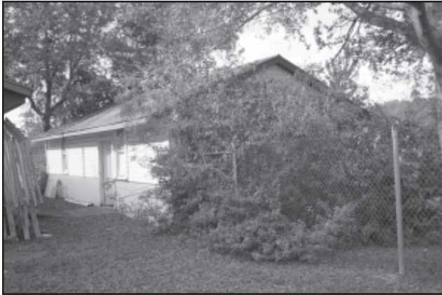
Figure 146. Exterior of the “Pole Barn”.
