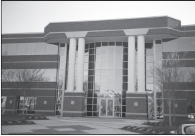
Figure 249. Exterior of the office building that contains the TRC Garrow and Associates offices.
