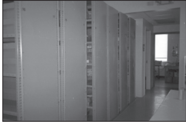
Figure 219. The long-term, movable, metal storage units.
