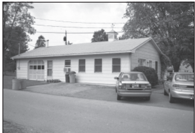
Figure 256. Exterior of the laboratory.
