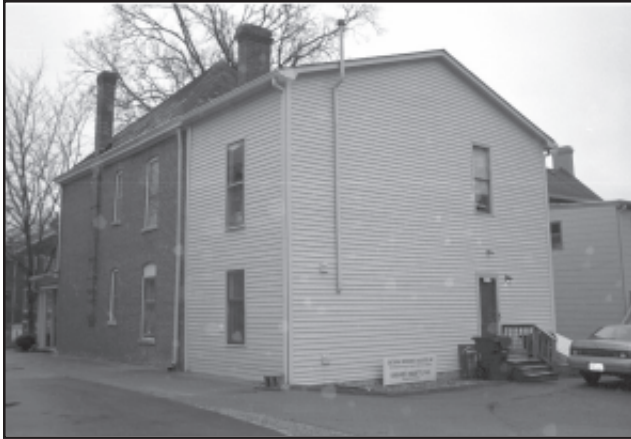
Figure 191. The addition that serves as the laboratory and collections storage area.
