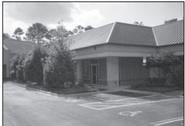
Figure 119. The building with Environmental Services offices.
