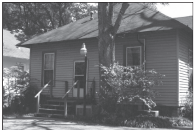
Figure 158. The back entrance exterior.
