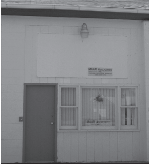
Figure 116. Exterior of warehouse with door and window leading into MAAR Associates office.
