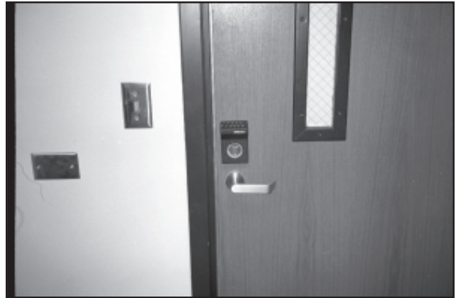
Figure 97. Omni lock system for the storage room at the Laboratory of Human Osteology.
