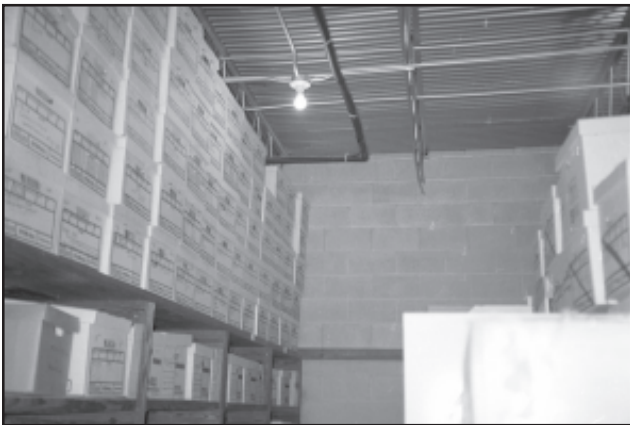
Figure 95. Interior walls of the collections storage area.
