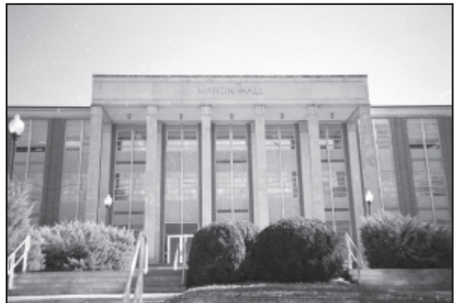
Figure 87. Front view of Martin Hall, where Fort McClellan collections are stored in the Archaeological Resource Laboratory.
