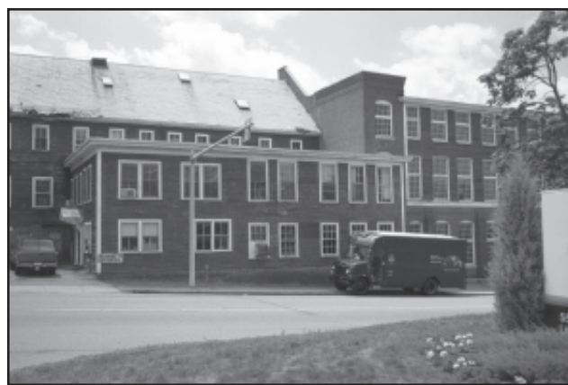
Figure 207. Turn-of-the century mill that now houses the Timelines offices.
