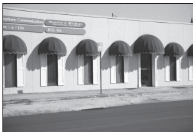
Figure 84. Exterior of building that contains ECG's offices.
