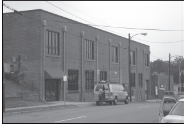
Figure 247. Front of the newly renovated West Lane Street Warehouse, where the new laboratory and storage repository are located.
