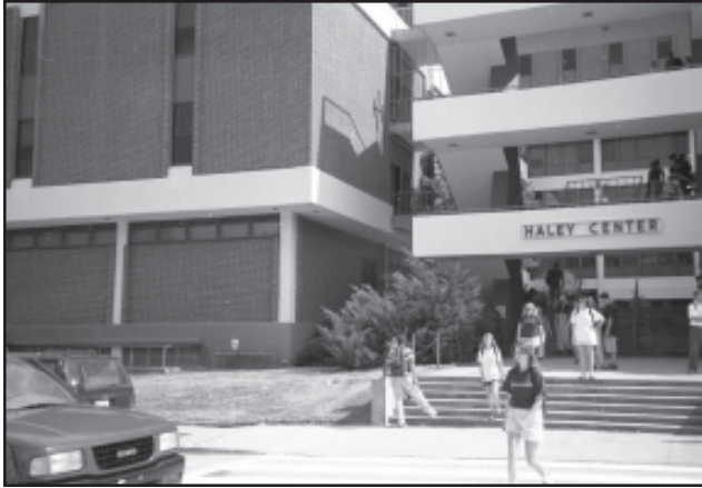
Figure 81. The foundation of the Haley Center.
