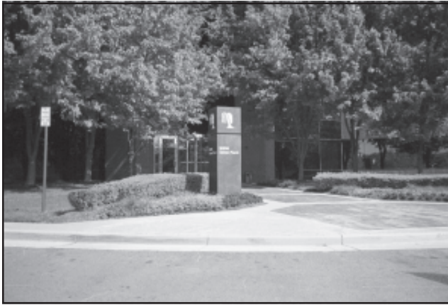
Figure 290. Exterior of Building 10306. Building 10300 looks the same.
