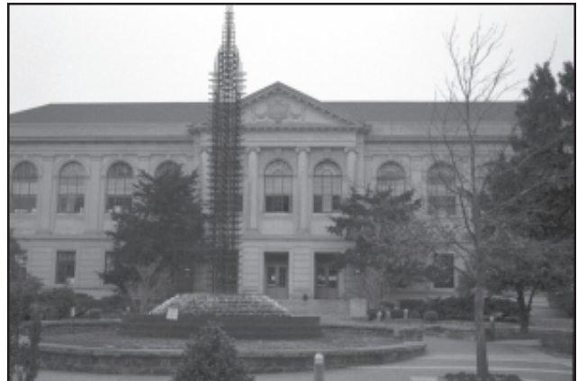
Figure 108. The front of Vol Walker Hall.
