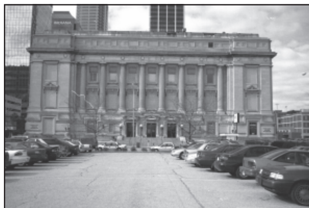
Figure 175. Exterior of the Indiana State Museum.
