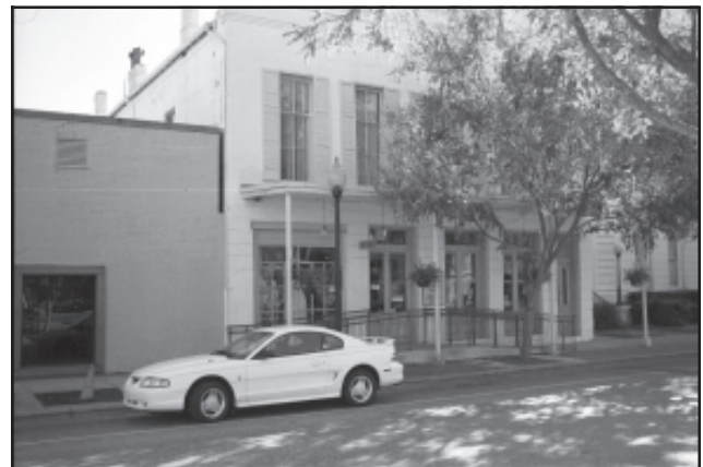
Figure 136. Exterior view of the entrance to the Pensacola Historical Society.
