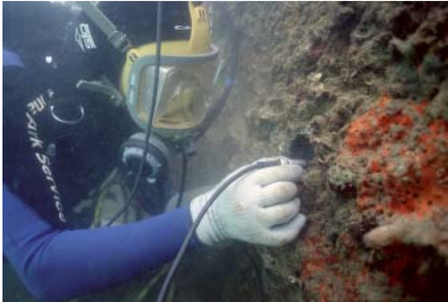
Figure 5. Deploying the ultrasonic thickness probe on Arizona 's hull.
