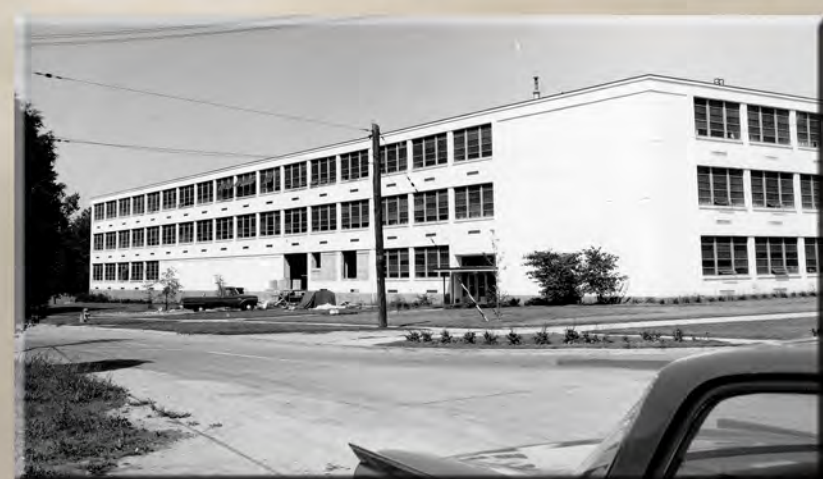
Gates-Lord Hall, Defense Information School, Fort Benjamin Harrison, under construction in 1965.
