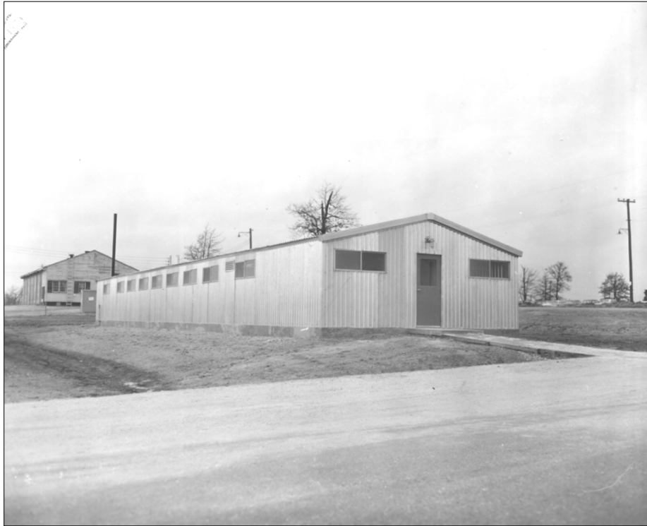
Figure 35. Exterior of prefabricated metal troop housing at Fort Leonard Wood, Missouri, November 1966 (NARA SC635542).
