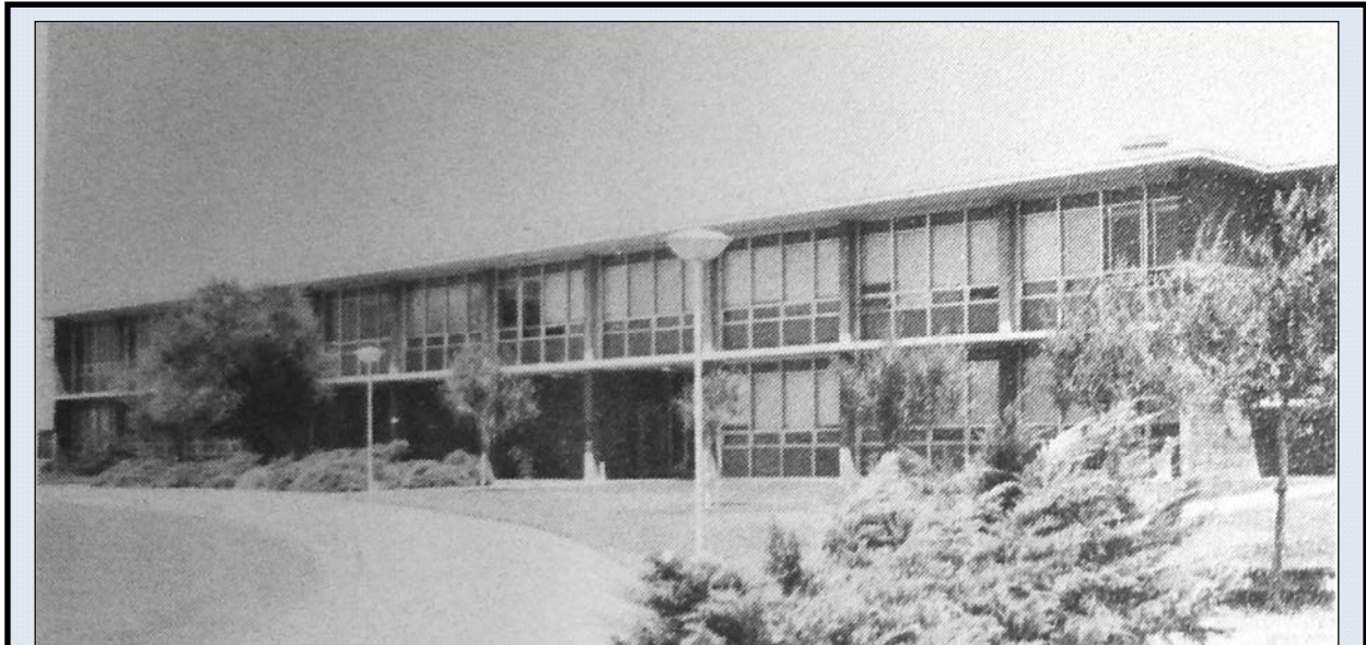
Figure 37: NAS Lemoore Administration Building (Facility 700) ca. 1965 features multi-light vertically aligned windows with solid panels above and below. The windows are grouped between concrete structural posts, and sheltered under a wide roof eave (photo: Golden Eagle circa 1965).
