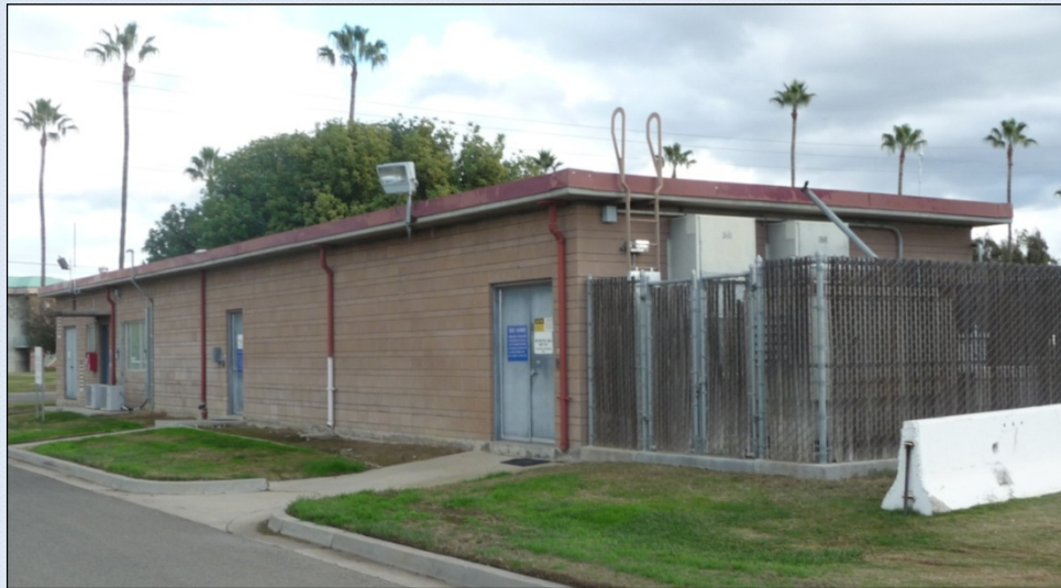
Figure 34: NAS Lemoore Facility 740, Telephone Exchange Building (photo: JRP).
