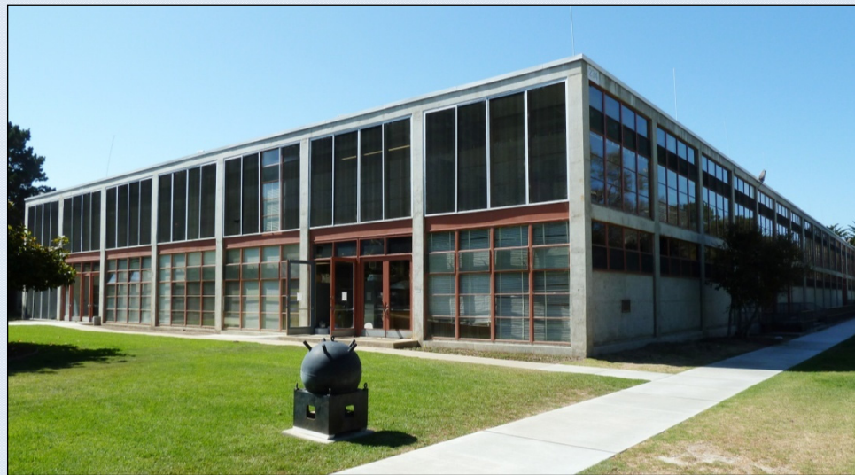
Figure 43: Halligan Hall (Facility 234) is defined by its grid-style design with flush window walls separated by structural concrete columns (photo: JRP).
