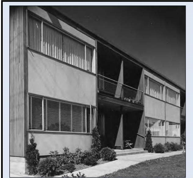
Figure 70: Bassetti & Morse-designed Gamma Rho Apartment building is a Seattle Historical Site (photo: Dearborn-Massar).
