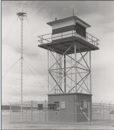
Figure 77: Spotting Tower at Range B-16 at NAS Fallon (photo: JRP 2012).
