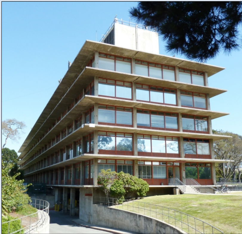
Figure 42: Five-story tall Spanagel Hall (Facility 232) features distinctive cantilevered canopies sheltering grouped windows filling most of the space between concrete structural columns (photo: JRP).
