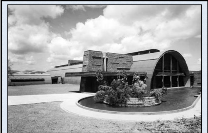
Figure 13: The Camp Parks Chapel and Library in Dublin, CA was constructed in 1945 by Bruce Goff from three standard dimension Quonset huts (photo: Decker and Chiei).
