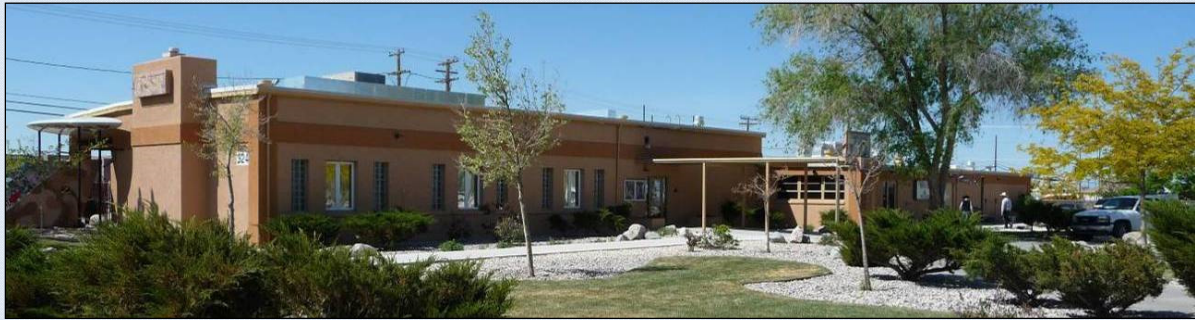
Figure 84: The Commissioned Officers' Club, Building 324, was among several buildings designed by the firm Lockard and Casazza. Featuring collaboration between Lockard and Mathews, it was built in 1959, but received additions and alterations in 1987 and 1997 (photo: JRP).
