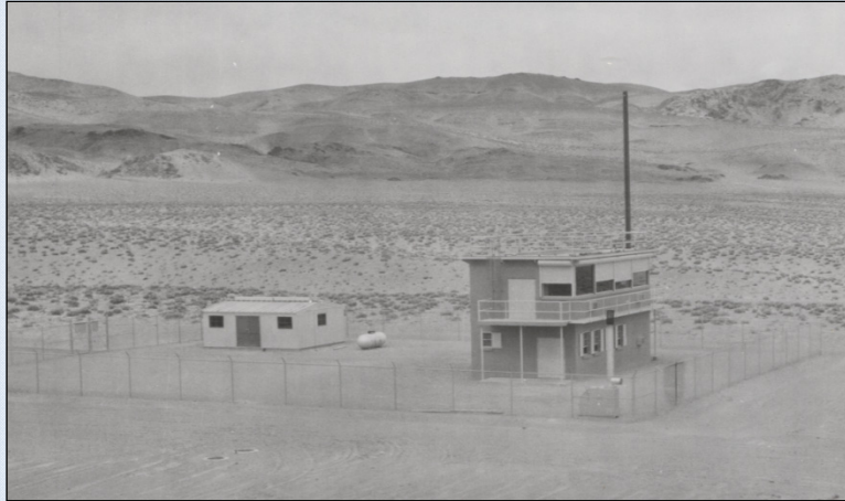
Figure 78: Building 612, Control Tower Building (right) and Building 613, Electrical Production Building at Range B-16 at NAS Fallon (photo: JRP 2012).
