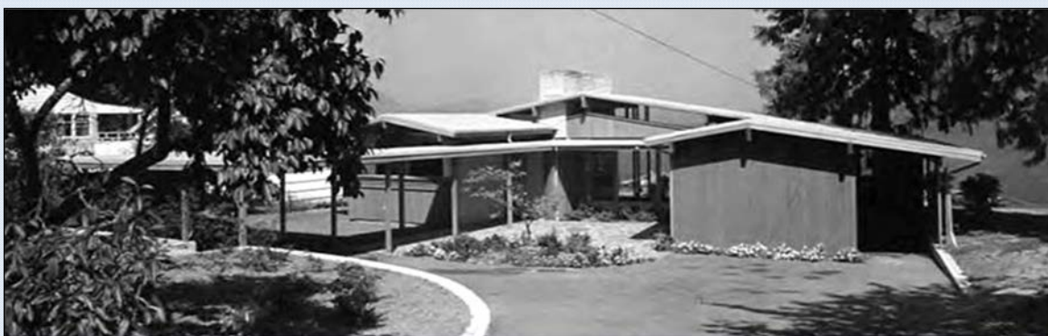
Figure 69: Ambruster Residence built in 1951 with parallel low-pitch gable roofs, clerestory windows, and exposed natural materials (photo: Dearborn-Massar).
