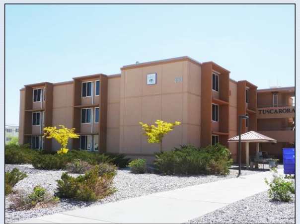
Figure 21: Despite modifications, Building 358 at NAS Fallon retains original form (photo: JRP).
