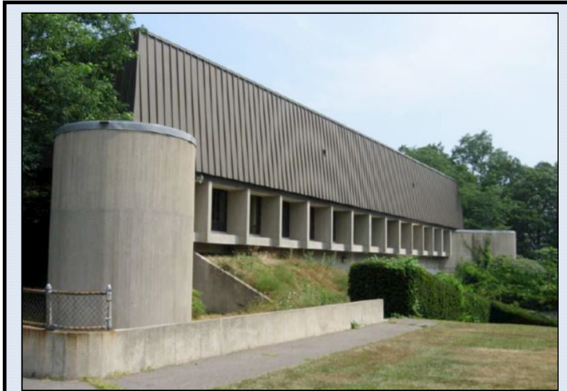
Figure 29: The left photograph shows the front (north) elevation of Connecticut Hall (1970) shortly after its completion. The front corner tower elements are today largely obscured by vegetation. On right is the rear of the building as seen in 2009 (photo: Karmazinas 2009).
