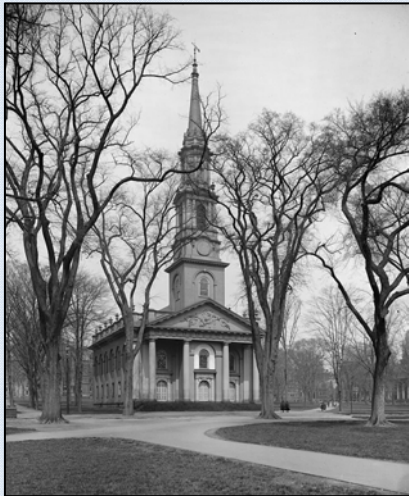
Figure 25: Center Church on the New Haven Green seen in the early twentieth century (photo: Library of Congress).
