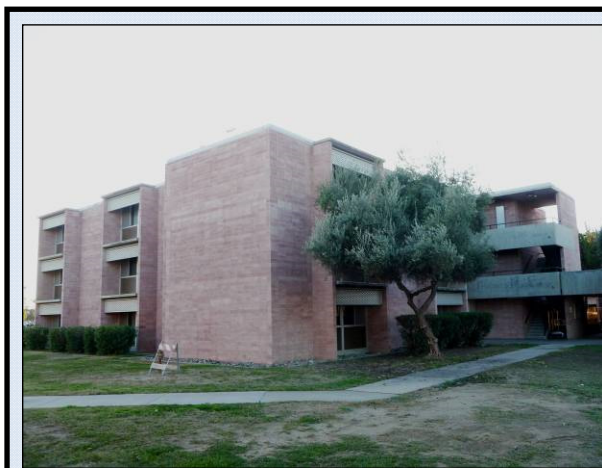
Figure 20: Building 888 at NAS Lemoore with mostly original features (photo: JRP).
