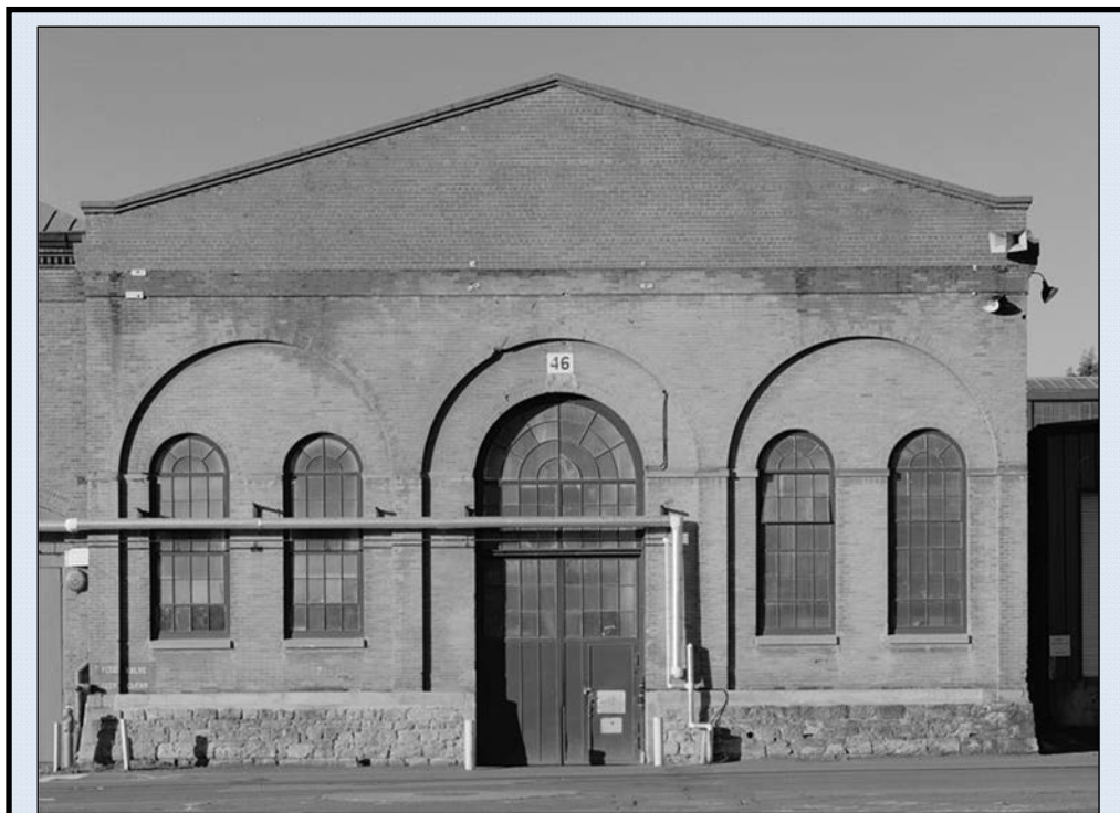
Figure 2: Building 46, an 1856 smithery, is the oldest shop building on Mare Island and one of the oldest and best preserved industrial buildings in California (photo: McDonald 1983).
