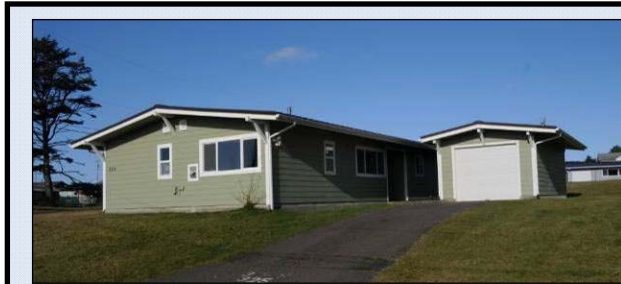
Figure 71: Building 325 is a modestly designed a Capehart program house at Naval Facility Pacific Beach by Bassetti & Morse featuring a Pacific Northwest Modern style aesthetic (photo: Sackett 2012).
