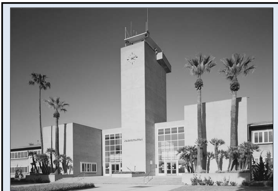
Figure 12: The administrative building at Roosevelt Naval Base, built 1940-1941, shows the influence of high European Modernism. Designer Paul Revere Williams was the first African-American to join the American Institute of Architects (AIA) in 1923 (photo: Cole, Murray and Dewey 1996).
