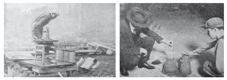
Illustrations 4 and 5: The images show the "Slump Test" inspection method for cast-in-place concrete, which is conducted on-site (Atlas Portland Cement Company 1927:12).
