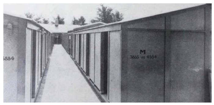
Illustration 40: Buildings often integrated both flat and corrugated asbestos-cement panels, as seen here (Johns-Manville 1944:28).
