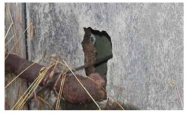
Illustration 79: Detail of a crumbled section of asbestos-cement located around a corroded pipe on Building 1507 at Picatinny Arsenal, indicating moisture as the cause (Photographer: Samantha Driscoll 2015).
