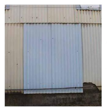
Illustration 87: Building 508 at NSF Indian Head replaced two formed corrugated asbestos-cement panels with corrugated metal panels. Attention was paid to the width of the corrugations, and the rhythm was maintained. The material should be painted to match the historic material surrounding it and camouflage the replacement material (Photographer: Samantha Driscoll 2015).
