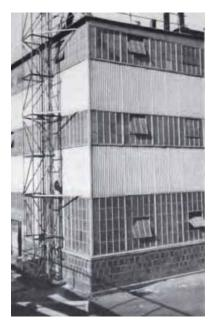
Illustration 39: An example of a curtain wall constructed with corrugated asbestos-cement panels (Johns-Manville 1944:33).
