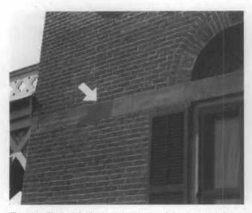
Illus. 21. Change of color over time is one of the greatest problems of synthetic substitute materials used outdoors. Ultra-violet light can cause materials to change color over time; some will lighten and others will darken. In this photograph, the synthetic patching material to the sandstone banding to the left of the window has aged to a darker color. Photos: Sharon C. Park, AIA.
