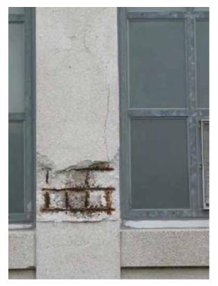
Illustration 50: The grid of the steel reinforcement is visible on NSFC Building 1, as the rusted steel has caused the delamination and spalling of the surface concrete (Graves 2012).
