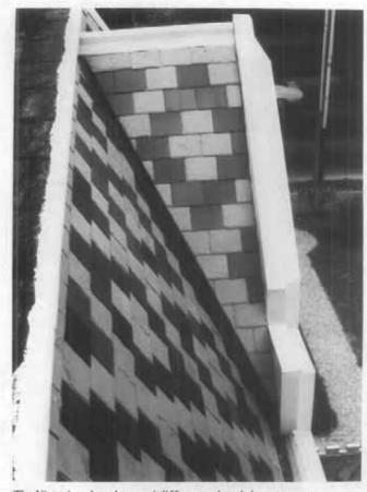
The Victorians loved to used different colored slates to create decorative patterns on their roofs, an effect which cannot be easily duplicated by substitute materials. Before any repair work on a roof such as this, the slate sizes, colors, and position of the patterning should be carefully recorded to assure proper replacement. (Ebenezer Maxwell Mansion, Philadelphia, Pennsylvania, photo courtesy of William D. Hershev)
