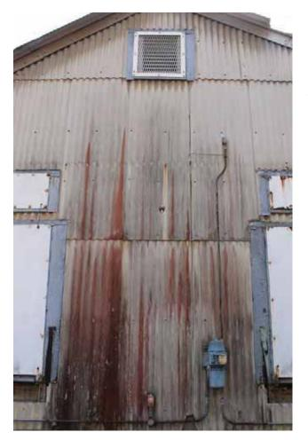
Illustration 83: The corrugated asbestos-cement cladding has severe stains, indicating lichen growth (Photographer: Samantha Driscoll 2015).
