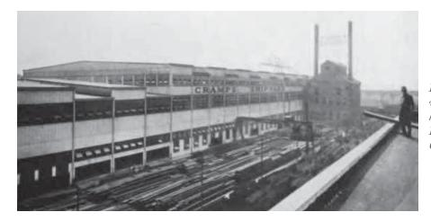
Illustration 27: Asbestos-cement corrugated siding was ideal for large buildings, especially those in harsh environments like this shipyard building in Philadelphia, Pennsylvania (Keasbey & Mattison Company 1918:11).
