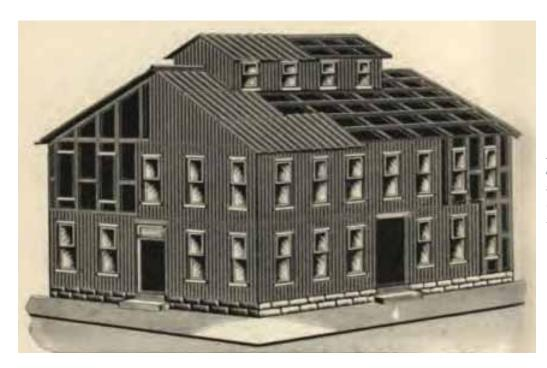
Illustration 7: An example of corrugated metal roofing and siding used on a skeleton frame building (Milwaukee Corrugating Co. 1920:154).
