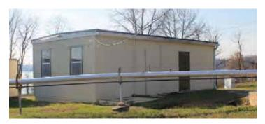
Illustration 85: Building 544D has flat panel asbestos-cement, which was set to be replaced, but instead was maintained through sealing and painting (Photographer: Samantha Driscoll 2015).
