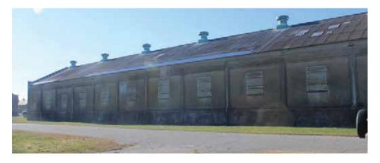
Illustration 88: Building 74 at NNSY, St. Juliens Creek Annex has several corrugated metal patches on the corrugated asbestos-cement roof. While the replacement patches have similar corrugation widths, the difference in materials in obvious. If the corrugated metal was painted, the patches would blend more with the historic fabric (Photographer: Samantha Driscoll 2016).
