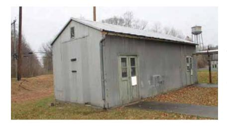
Illustration 73: Building 1506 at Picatinny Arsenal is clad in corrugated aluminum. In the center of the front elevation is a patch of in-kind material fitted with incompatible fasteners (Photographer: Samantha Driscoll 2015).
