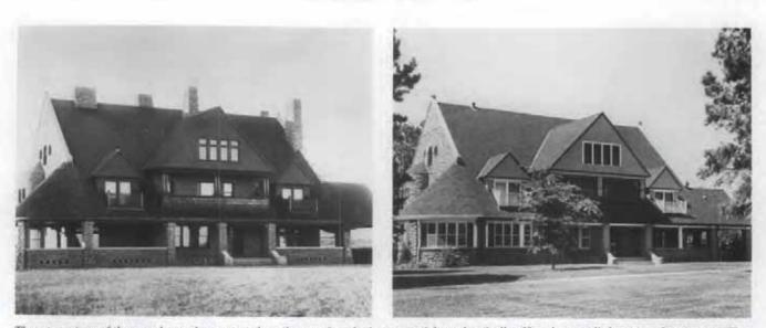
These two views of the same house demonstrate how the use of a substitute material can drastically affect the overall character of a structure. The textural interest of the original tile roof was lost with the use of asphalt shingles. Recent preservation efforts are replacing the tile roof. (Frank House, Kearney, Nebraska, photo courtesy of the Nebraska State Historical Society, Lincoln. Nebraska)
