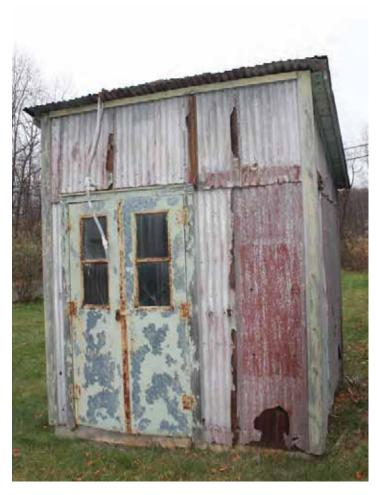
Illustration 68: Building 1504A at Picatinny Arsenal has suffered a lack of maintenance, resulting in corrosion (Photographer: Samantha Driscoll 2015).
