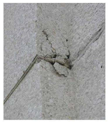
Illustration 52: An example of a pop-out around a joint on Building 1 at NSFC (Graves 2012).
