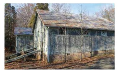
Illustration 71: Building 179 at NSF Indian Head shows the galvanized corrugated steel cladding, though not maintained, is not experiencing corrosion. The corrugated steel roof appears to have had a treatment, though it failed and corrosion has occurred (Photographer: Samantha Driscoll 2015).
