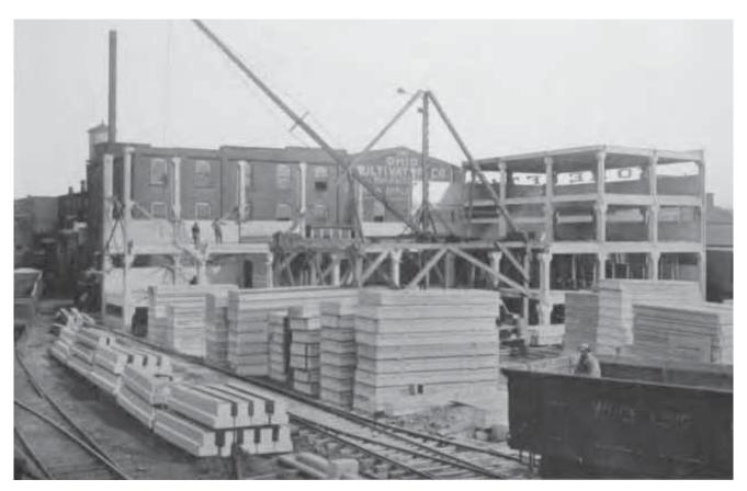
Illustration 2: A precast concrete building within the Ohio Cultivator Co. complex in Bellevue, Ohio, during construction. The precast concrete elements stacked in the foreground were delivered to the site and moved into place by a crane (Unit Construction Co. 1913:4).
