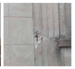
Illustration 55: Corrosion of steel reinforcement, as shown in this example from Building 173 at Picatinny Arsenal, is a common cause of spalling (Photographer: Samantha Driscoll 2015).
