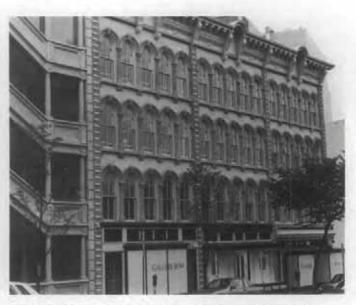
Illus. 22. A fiber reinforced polymer (fiberglass) cornice and precast concrete elements replaced deteriorated features on the 19th-century exterior. Photo: Sharon C. Park, AIA.
