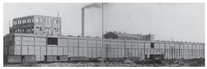
Illustration 1: The exterior of a building within the National Lead Company complex in St. Louis, which was constructed with reinforced precast concrete panels (Unit Construction Co. 1913:16).
