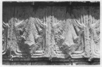
Tin shingles, commonly embossed to imitate wood or tile, or with a decorative design, were popular as an inexpensive, textured roofing material. These shingles 8<sup>3</sup>/<sub>n</sub> inch by 12<sup>1</sup>/<sub>2</sub>, inch on the exposed surface) were designed with interlocking edges, but they have been repaired by surface nailing, which may cause future leakage. (Ballard House, Yorktown, Virgina, photo by Gordie Whittington, National Park Service)
