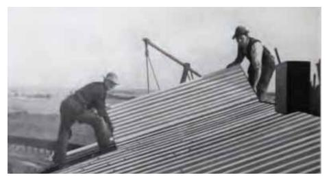
Illustration 30: The application of asbestos-cement corrugated roofing on a steel structure (Keasbey & Mattison Company 1918:28).
