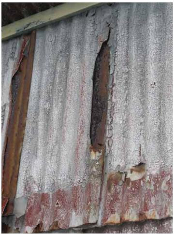
Illustration 69: Detail of corrosion on Building 1504A. Painting is the primary maintenace of corrugated steel, as it protects the steel from moisture (Photographer: Samantha Driscoll 2015).
