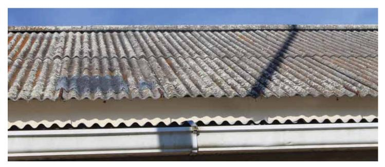
Illustration 76: Building 466 at NSF Indian Head has a corrugated asbestos-cement roof with degradation. The material has begun to break down and looks rough, which may release asbestos fibers (Photographer: Samantha Driscoll 2015).
