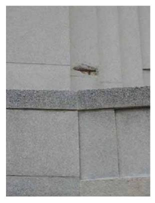
Illustration 49: A section of rusted steel reinforcement on NSFC Building 1 has resulted in the spalling of the concrete (Graves 2012).
