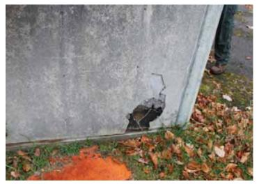
Illustration 78: Detail of a crumbled section of asbestos-cement on Building 1507 at Picatinny Arsenal (Photographer: Samantha Driscoll 2015).
