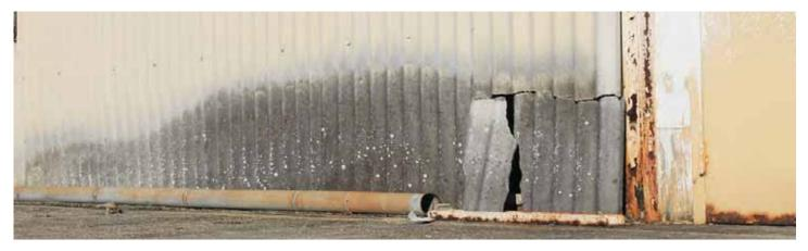
Illustration 82: Detail of the staining, erosion, discoloration, and lichen growths on Building 448, indicative of degradation (Photographer: Samantha Driscoll 2015).
