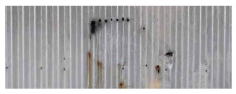
Illustration 74: Detail of the in-kind material patch on Building 1506. Note the alignments of the corrugations make the patch almost undetectable, but the corroded steel fasteners have caused staining (Photographer: Samantha Driscoll 2015).
