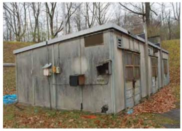
Illustration 77: Building 1507 at Picatinny Arsenal is clad in flat panel asbestos-cement that is heavily stained, indicating degradation (Photographer: Samantha Driscoll 2015).
