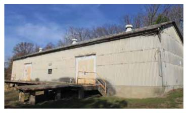
Illustration 80: Building 448 at NSF Indian Head is clad in corrugated asbestos-cement. Note the dark degradation areas along the foundation line (Photographer: Samantha Driscoll 2015).
