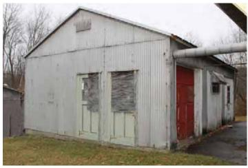
Illustration 67: Building 1504 at Picatinny Arsenal, built in 1956, is an example of aluminum corrugated metal. Note there is no evidence of corrosion (Photographer: Samantha Driscoll 2015).
