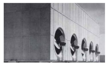
Illustration 24: An example of flat asbestos-cement panels on a cooling tower (Johns-Manville 1944:13).
