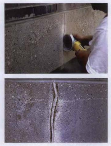
Figure 19. A high-speed grinder ia used to widen a crack in preparation for installation of a sealant. This process is called "routing." After the crack is prepared, the sealant is installed to prevent moisture infiltration through the crack. Although sealant repairs can provide a durable, watertight repair for moving cracks, they tend to be very visible.
