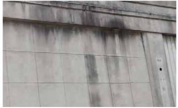
Illustration 58: Detail of staining on Building 173 at Picatinny Arsenal. The last cleaning of the concrete is estimated to have occurred between 20 and 30 years ago (Photographer: Samantha Driscoll 2015).
