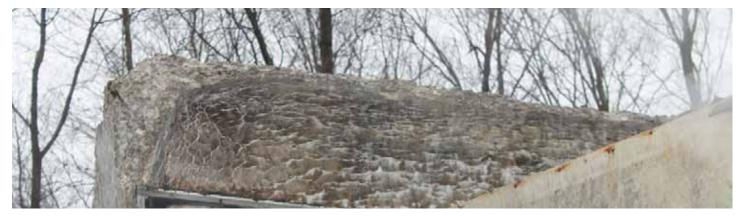
Illustration 56: Building 1507 at Picatinny Arsenal has a rather extreme example of efflorescence, cracking, and spalling due to moisture infiltration (Photographer: Samantha Driscoll 2015).
