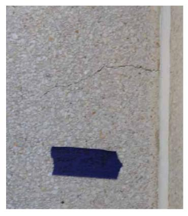
Illustration 51: An example of a hairline crack on Building 3 at NSA Bethesda. The concrete is undergoing repairs, and the blue tape is used to mark the location of a crack that will be filled with an epoxy injection (Photographer: Samantha Driscoll 2015).
