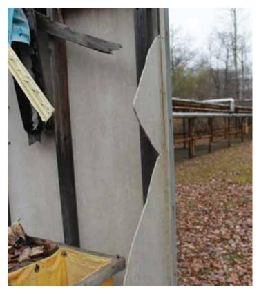
Illustration 86: Detail of Building 1508 at Picatinny Arsenal where large sections of flat panel asbestos-cement have been broken. Note the thin, brittle nature of asbestos-cement (Photographer: Samantha Driscoll 2015).
