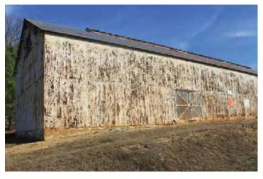
Illustration 66: Building 224 at NSF Indian Head, built in 1915, is an example of steel corrugated metal. Note the amount of corrosion below the peeling paint (Photographer: Samantha Driscoll 2015).
