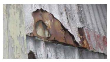
Illustration 70: Corrosion is not just an aesthetic issue, it can make the material unstable. As seen here, the corrosion has caused a hole in the corrugated steel (Photographer: Samantha Driscoll 2015).
