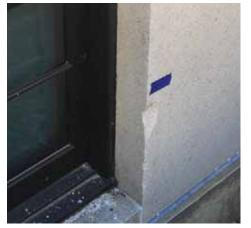
Illustration 53: An example of spalling on Building 3 at NSA Bethesda. The concrete is undergoing repairs, and the blue tape is used to mark the location of a needed repair (Photographer: Samantha Driscoll 2015).
