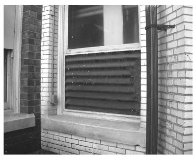
Figure 52. Air intakes can be integrated into existing upper level architectural features such as a window (ERDC-CERL 2005).
