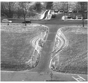
Figure 8. Roadway edge treatments near ACPs can deter their misuse.
