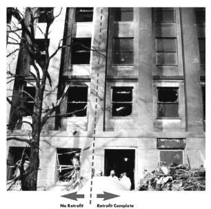
Figure 39. Pentagon immediately after September 11, 2001, showing intact blast-resistant windows at right (DON 2001).
