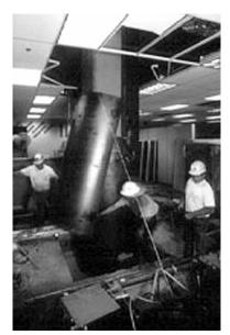
Figure 17. Seismic application of a steel jacket on an existing concrete column (Morley Builders 1997).
