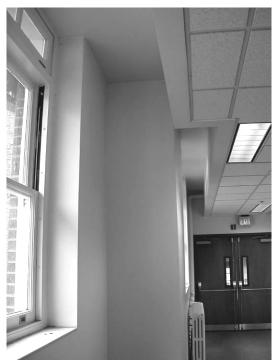
Figure 47. Ceilings dropped to accommodate new ductwork should be pulled away from historic fenestration. Historic radiators and operable windows and transoms should be retained (ERDC-CERL 2004).
