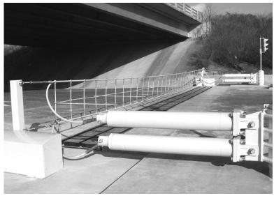
Figure 10. Above-grade components of vehicle net barriers may create a visual challenge when installed a historic landscape (Universal 2005).
