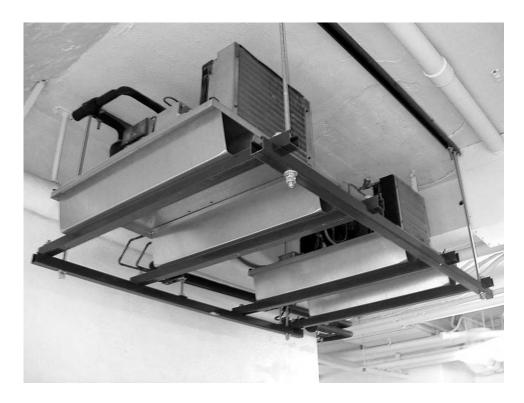
Figure 55. This ceiling mounted equipment rack will likely need horizontal or diagonal bracing to comply with the UFC (ERDC-CERL 2005).
