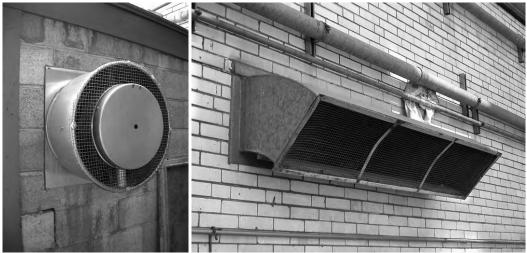
Figure 54. Exhaust vents come in various configurations and should be selected to blend with the historic architecture (ERDC-CERL 2005).
