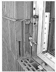
Figure 43. Window anchors in clay tile masonry (ENR 2003).
