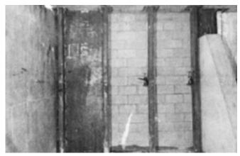
Figure 24. Steel column and plate application (Ward 2004).
