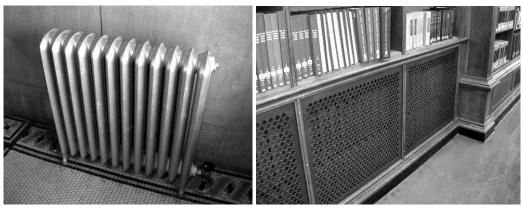
Figure 48. Cast-iron radiators can be left exposed (left) or encased in cabinetry (right) (ERDC-CERL 2005).
