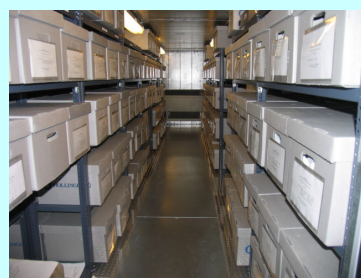
Fort Riley's Curation Facility Left: Outside of the retrofitted "meat locker." Right: Inside of the secure facility
