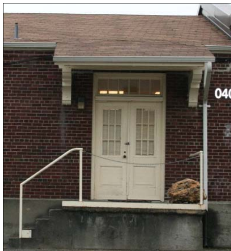
A simple entrance with a roof supported by brackets. Fort Lewis, Washington
