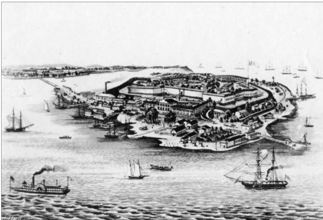
1861 drawing depicting the coastal fortification at Fort Monroe, Virginia. Drawing courtesy of Fort Monroe's Casemate Museum, Department of the Army
