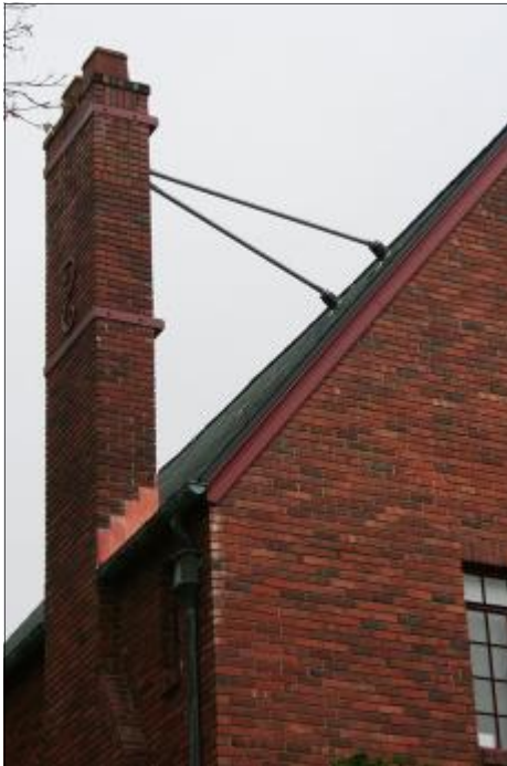
Compatible earthquake and wind retrofit. Naval Station Bremerton, Washington
