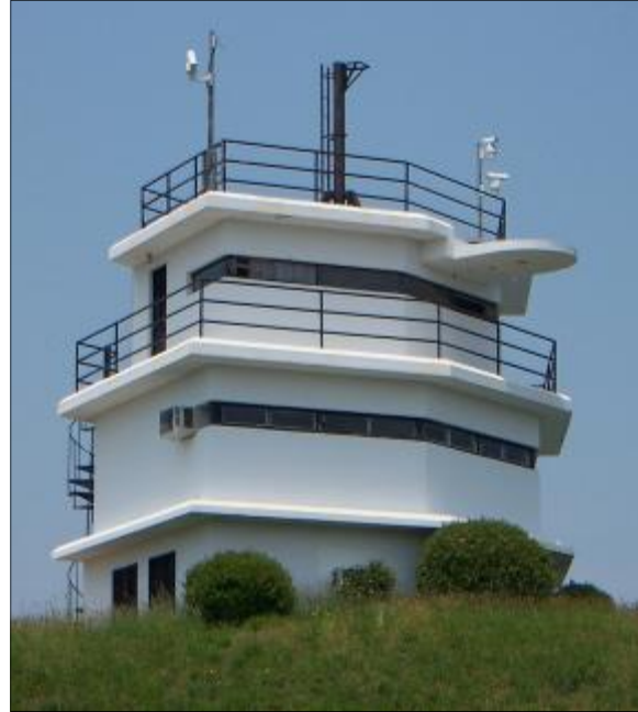
Old Military Affiliated Radio Station (M.A.R.S) designed in the International style. Fort Monroe, Virginia Photo courtesy of ERDC-CERL
