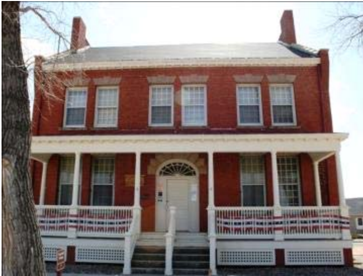
Administration Building F.E. Warren Air Force Base, Wyoming
