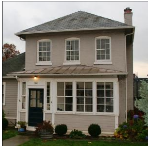
Pyramidal roof shape, former military building Vancouver Barracks, Washington
