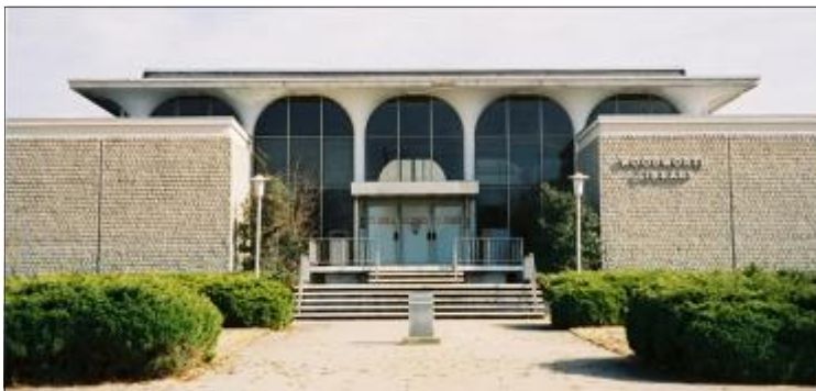
Library, Fort Gordon, Georgia, Photo courtesy of ERDC-CERL
