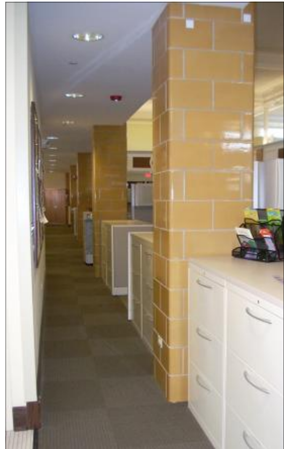
Interior columns were preserved during the rehabilitation of a former mess hall into office space. Naval Station Great Lakes, Illinois
