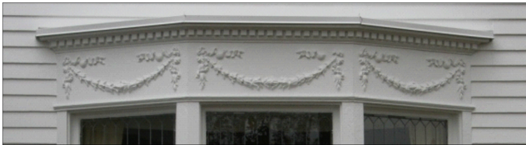
Garlands and dentil molding accent bay window. Naval Station Bremerton, Washington
