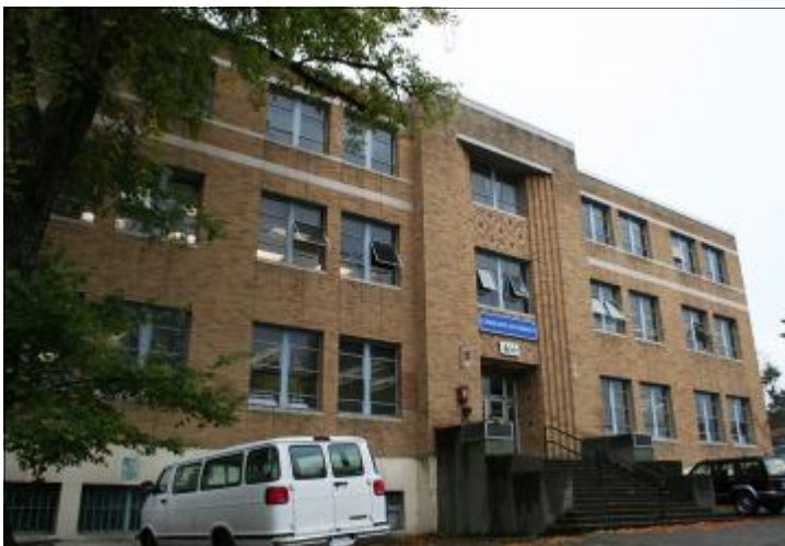
Administration Building Naval Station Bremerton, Washington
