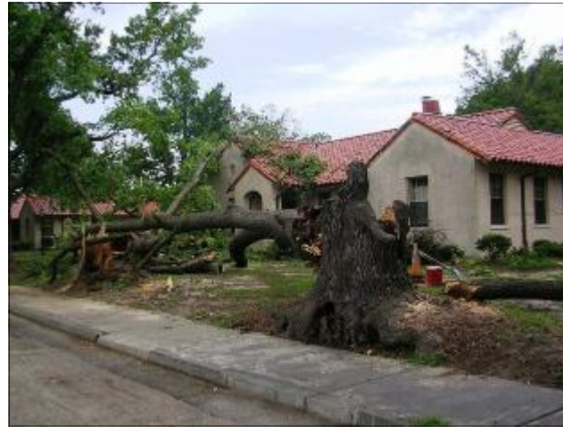
Fallen trees can harm historic buildings. Fort Bragg, North Carolina Photo courtesy of Fort Bragg CRMP
