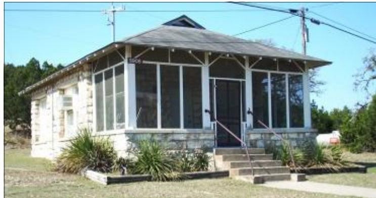
This house built by soldiers has unique features such as a gable-on-hip roof and engaged porch. Camp Bullis, Texas
