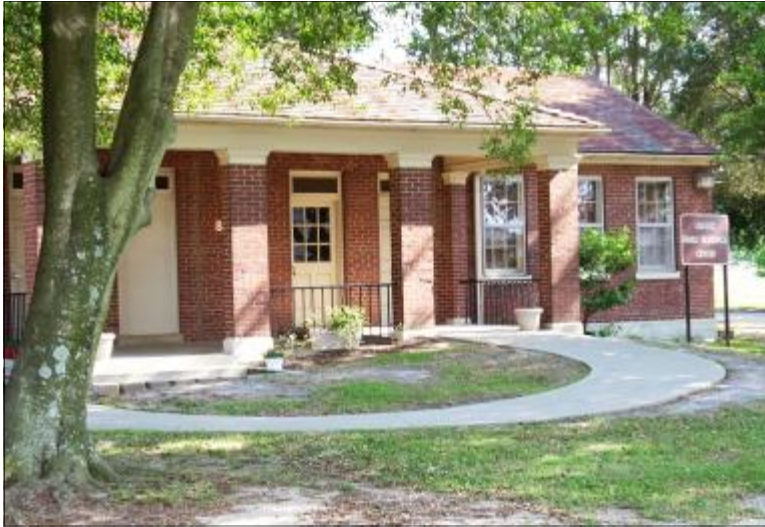
This curved ramp at Fort Bragg, North Carolina uses the landscape and has minimal impact to the historic building.
