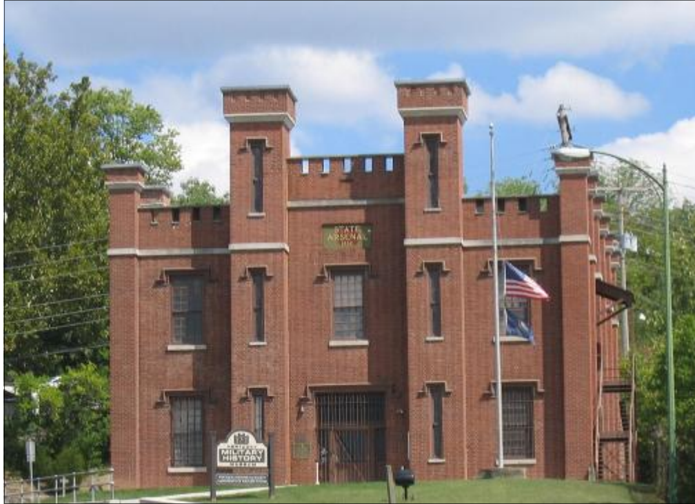
Old State Arsenal for Kentucky constructed in 1850. Currently home to the Kentucky Military History Museum. Frankfort, Kentucky. Photo courtesy of the Kentucky Army National Guard
