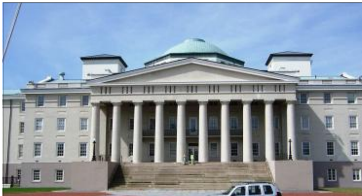
Naval Hospital with a later addition of the dome Portsmouth Naval Hospital, Virginia Photo courtesy of ERDC-CERL
