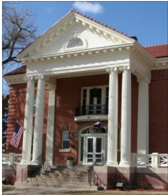
Wood was used for all types of architectural details including cornices, dentil moldings, columns and pediments. F.E. Warren Air Force Base, Wyoming
