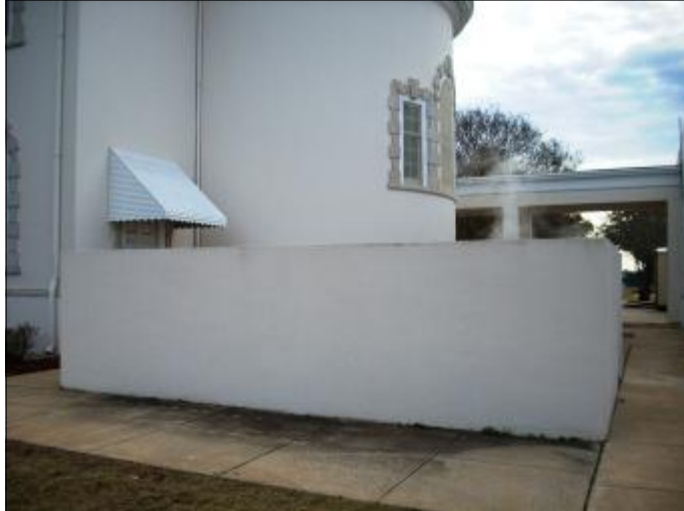
A wall constructed, using compatible materials, to screen a large HVAC system. Fort Benning, Georgia
