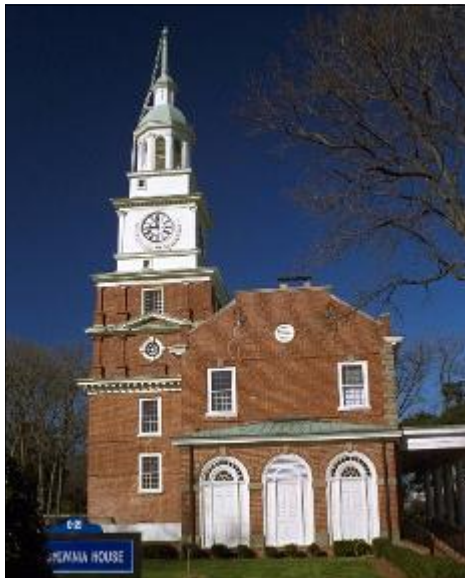
Pennsylvania Building, Naval Base Norfolk, Virginia Photo courtesy of the Department of the Navy
