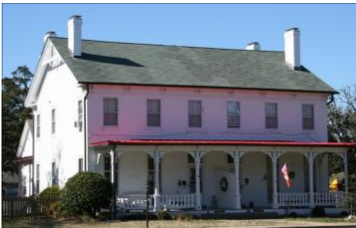
Quarters 15, Fort Monroe, Virginia
