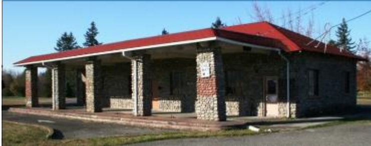
Service Station Fort Lewis, Washington
