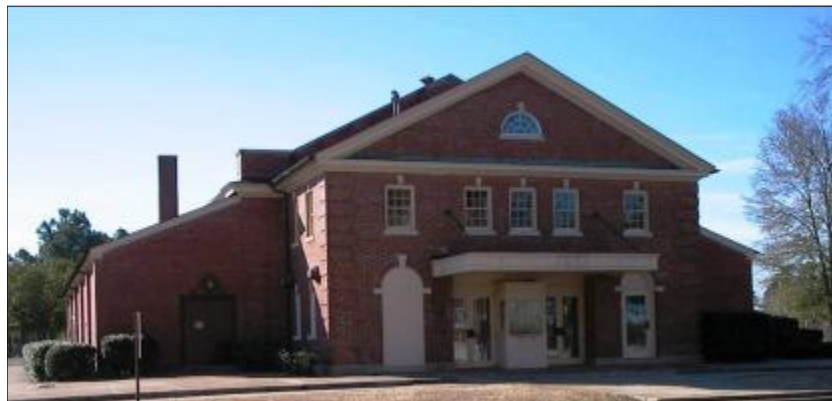
The side additions to this 1933 theatre were constructed in 1939 and thus are considered historic additions. Fort Bragg, North Carolina.
