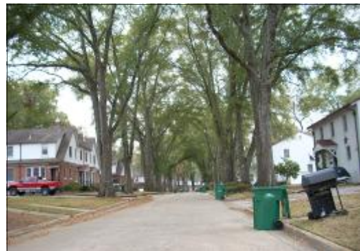
Alleyways can be important character-defining features of historic neighborhoods. Fort Benning, Georgia
