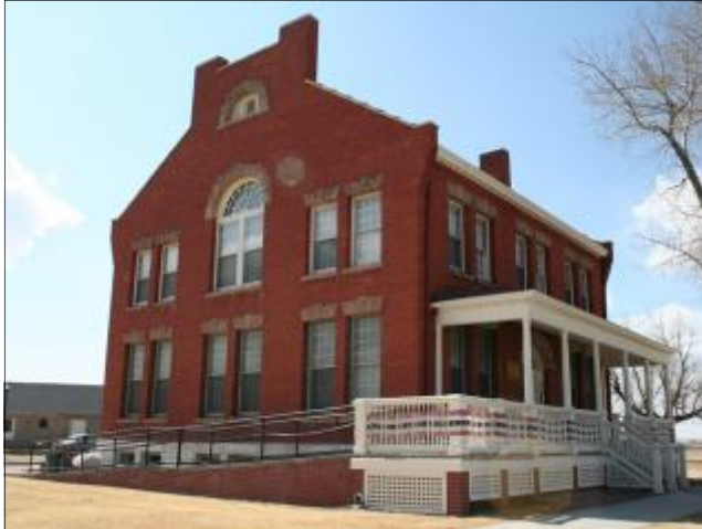
The handicap ramp was added to the side of this building to minimize the impact but provide accessibility. F.E. Warren Air Force Base, Wyoming
