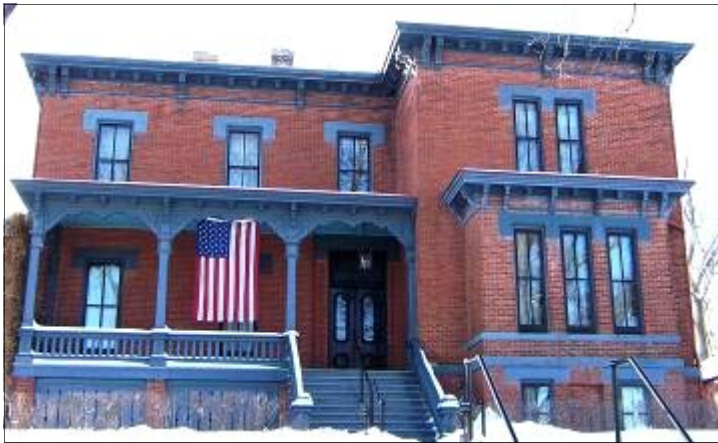
Former military Commanding General's Quarters Omaha Barracks, Nebraska, Photo courtesy of ERDC-CERL
