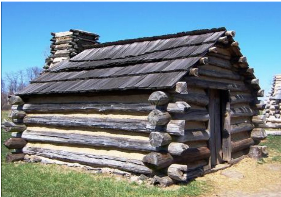
A reconstructed cabin at Valley Forge, Pennsylvania portraying the typical construction of early military buildings. Photo courtesy of ERDC-CERL
