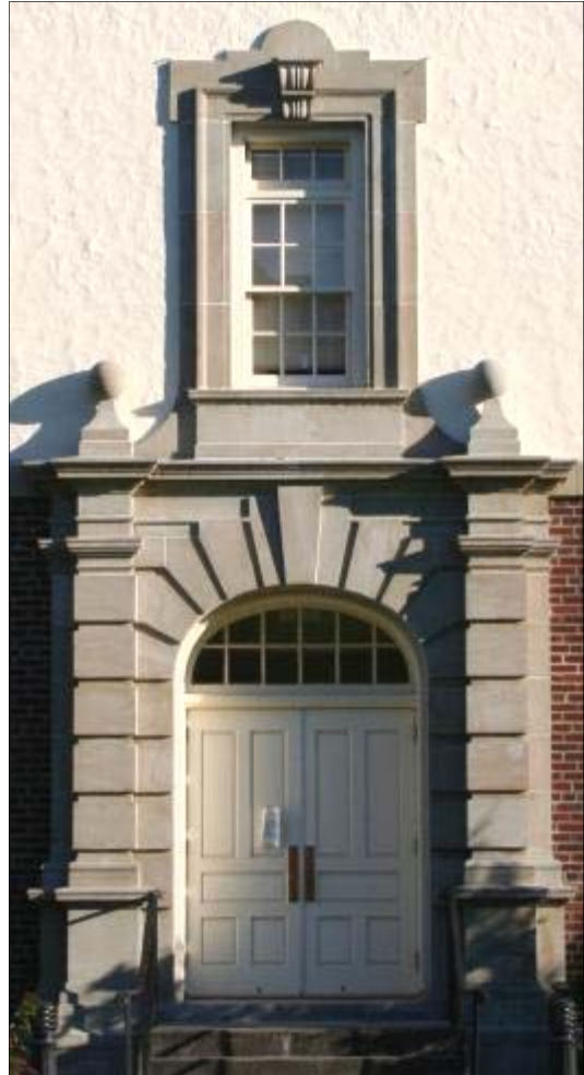
Barrack entrance with original doors and windows. Fort Lewis, Washington
