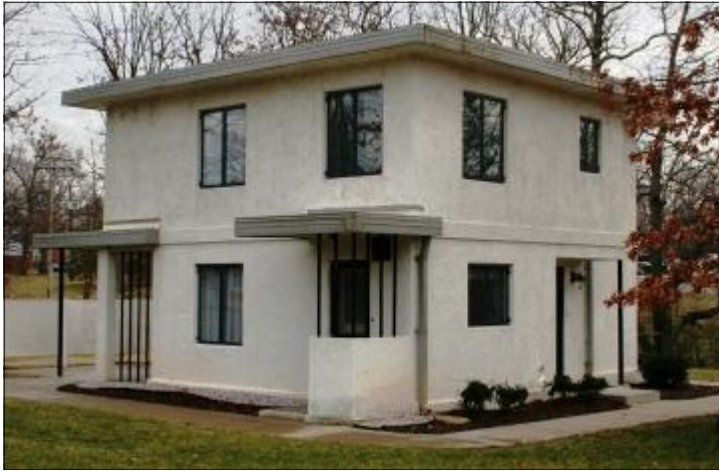
Thermo-Con House, Fort Belvoir, Virginia
