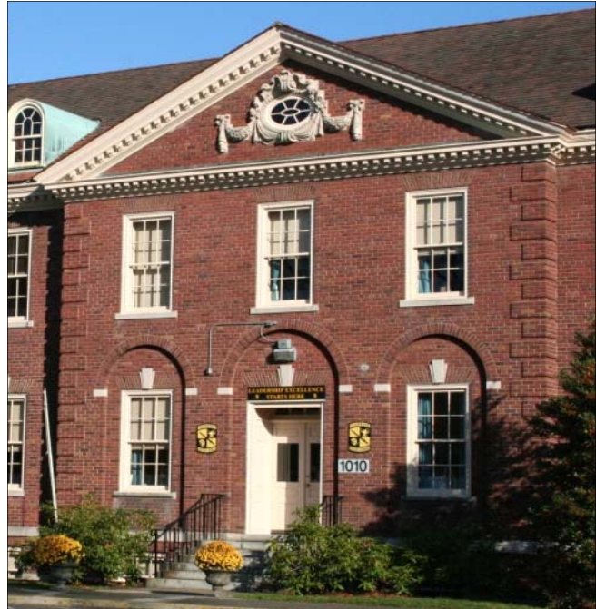
Various decorative architectural details such as quoins, dentil cornice, pediment, recessed arches and garland add character to a building. Fort Lewis, Washington
