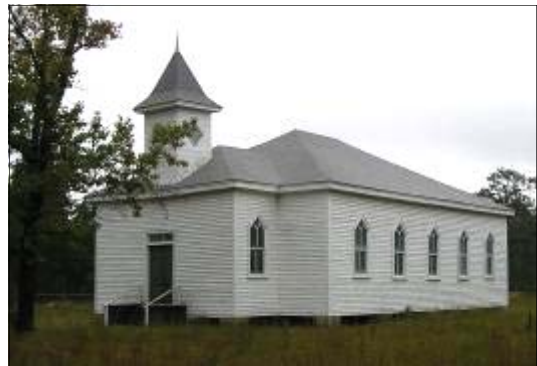
Sandy Grove Church designed and constructed by local community members in a vernacular building tradition. Fort Bragg, North Carolina Photo courtesy of Fort Bragg CRMP
