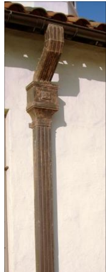
Example of a historic copper gutter. Randolph Air Force Base, Texas
