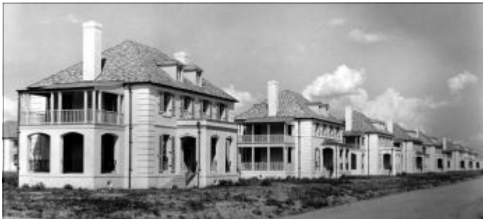
1932 historic photo of Officer quarters Barksdale Air Force Base, Louisiana National Archives, 342-FH Box 3B-16032 Barksdale Field LA NCO Quarters, Box 1055
