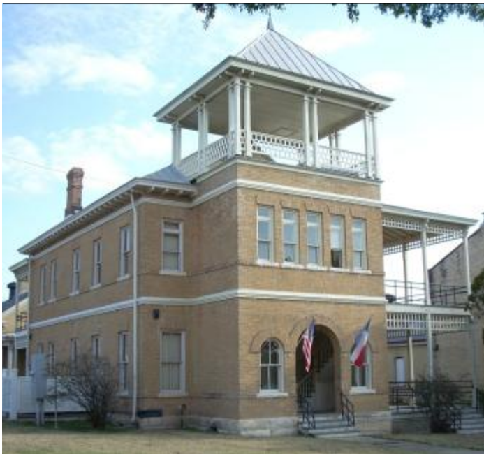
Band Hall Building Fort Sam Houston, Texas
