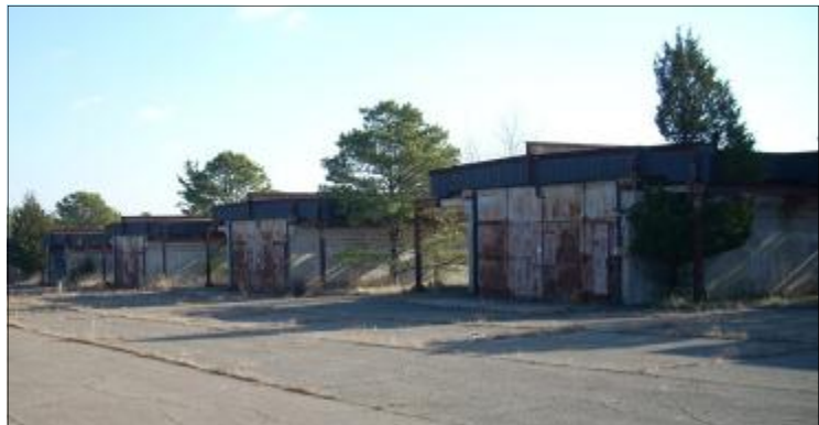
Cold War era building and missile shelters constructed as part of the air defense program. (Present-day photos) McGuire Air Force Base, New Jersey
