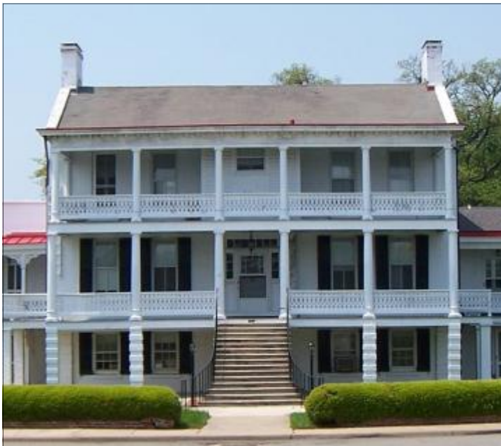
Quarters 1, Commanding Officer's Quarters Fort Monroe, Virginia Photo courtesy of ERDC-CERL
