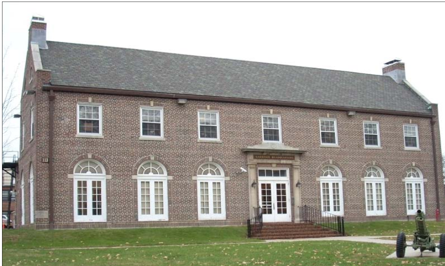
This building depicts a side gable roof with parapet ends. Fort Hamilton, New York
