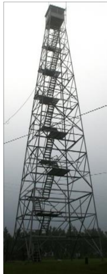
Metal provides the structural framework for this fire tower at Fort Stewart, Georgia.
