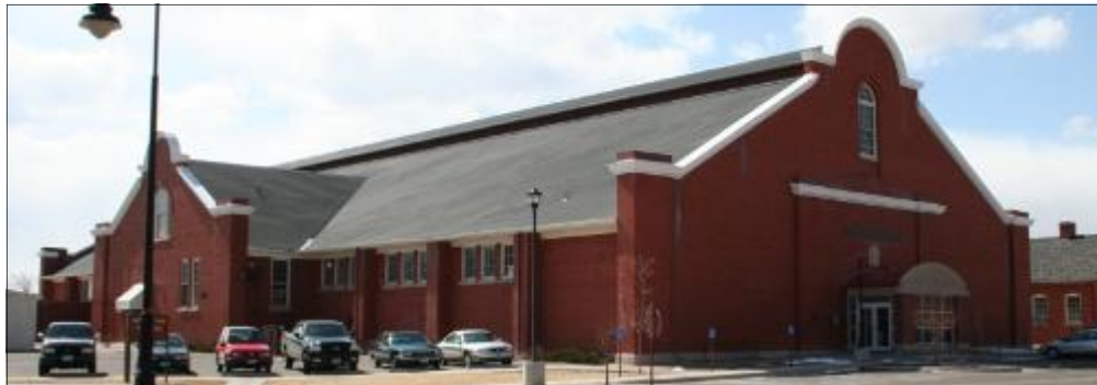
Prior to demolishing a historic building, seek other uses for the building such as adaptive reuse. This former riding arena was converted into a gym. F.E. Warren Air Force Base, Wyoming
