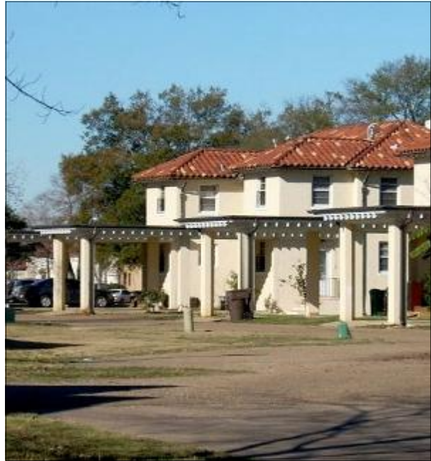
Addition of compatible carports to historic housing. Maxwell Air Force Base, Alabama
