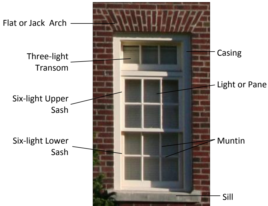
Original 6 over 6 double-hung wood sash window with a three-light transom.
