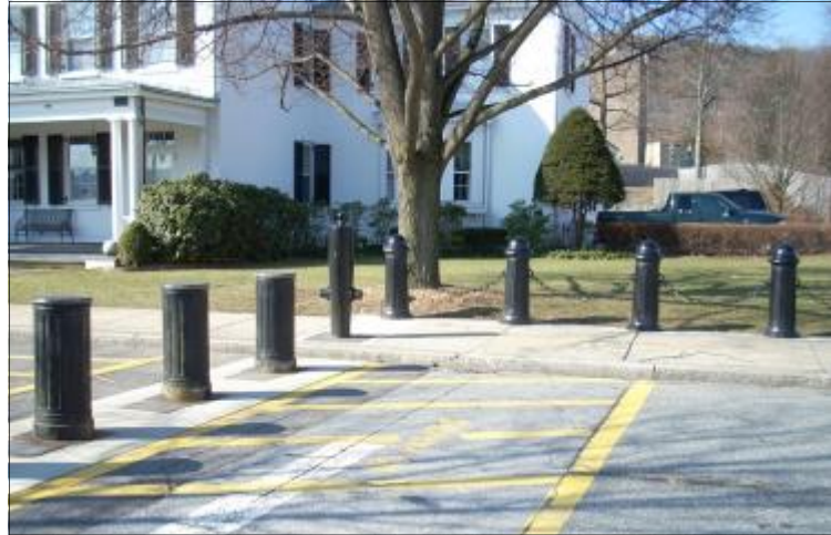
New bollards replicating historic ones lessen the visual impact to a historic district. United States Military Academy, New York
