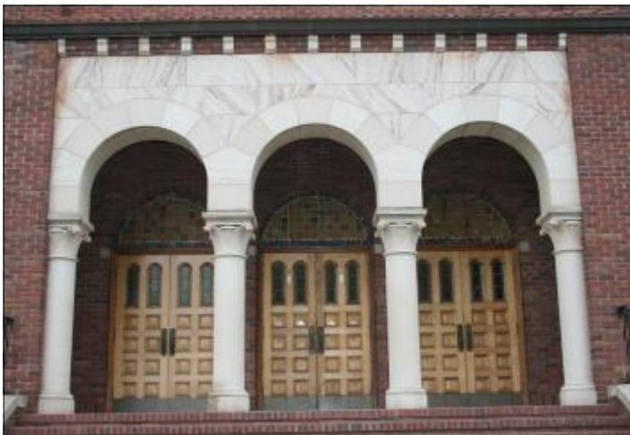
Contrasting building materials can provide architectural interest to walls. Fort Lewis, Washington
