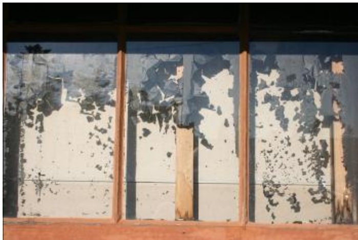
The effects of painting surfaces not meant to be painted. Avoid painting brick, concrete and glass, if not historically painted.
