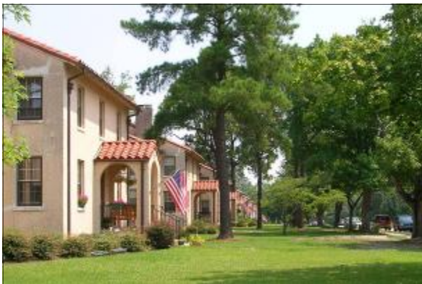
Historic family housing streetscape enhances the quality of the environment at Fort Bragg, North Carolina. Photo courtesy of Fort Bragg CRMP
