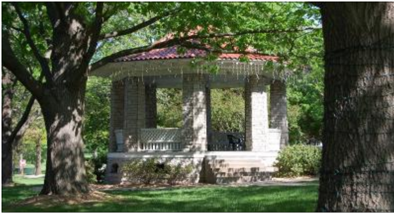
This historic gazebo is an important element in the historic district at Fort Leavenworth, Kansas.
