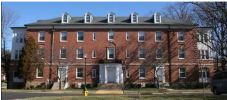
Multi-unit Family Housing Marine Corps Base Quantico, Virginia
