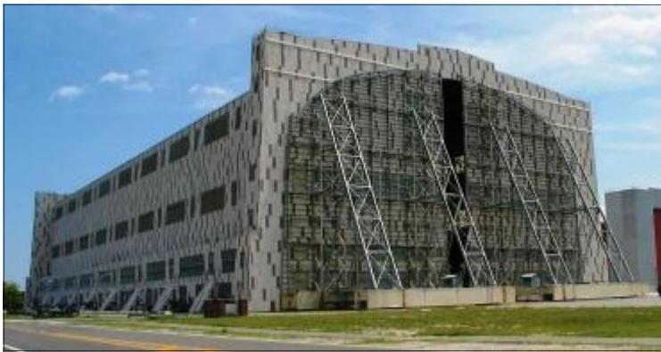
Hangar 1 Naval Air Engineering Station Lakehurst, New Jersey Photo courtesy of NAES Lakehurst Natural/Cultural Resources Manager
