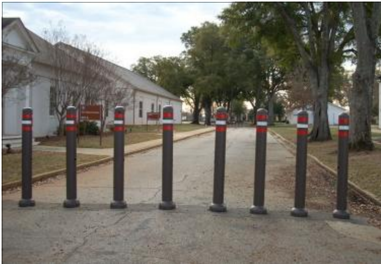
Rather than demolishing a historic paving pattern, use bollards to close off roads. Fort Benning, Georgia
