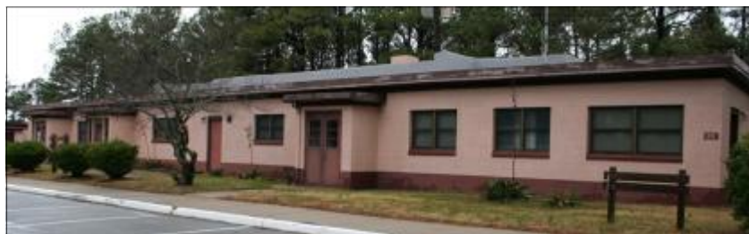
Barracks, Fort Eustis-Fort Story, Virginia
