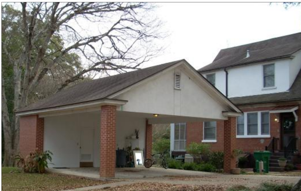
New carport utilizes similar building materials to minimize its impact to the historic district. Fort Benning, Georgia
