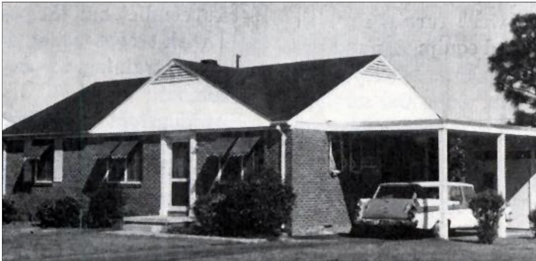
House constructed through the Wherry program at Fort Bragg, North Carolina. ca. 1950s Photo courtesy of Fort Bragg CRMP Archives.
