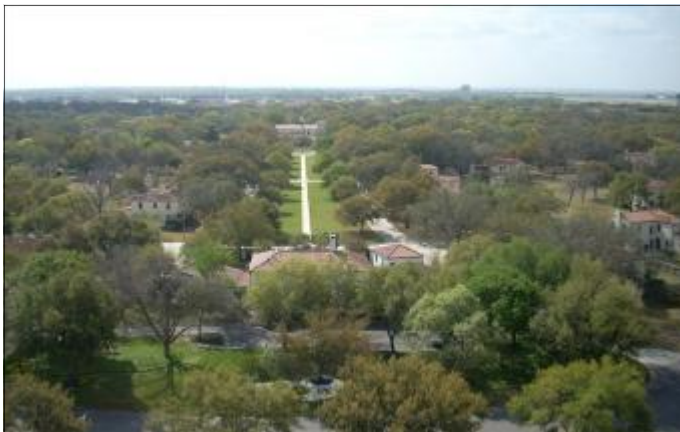
Central axes and symmetry play vital roles in the design of community plans and should be protected and preserved. Randolph Air Force Base, Texas
