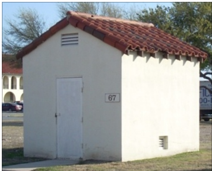
Historic accessory building, flare room Randolph Air Force Base, Texas
