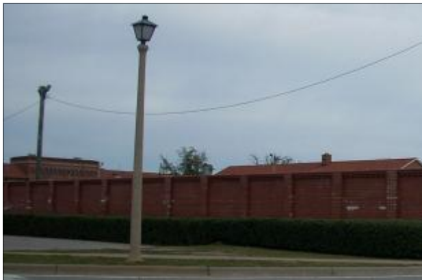
Contemporary wall constructed in brick to be compatible with the character of the historic district. Fort Benning, Georgia
