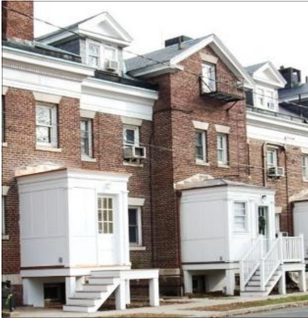
Compatible rear porch additions of officer housing provides an additional bathroom. Fort Hamilton, New York
