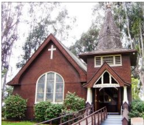
Former military St. Peter's Chapel (Shingle), Mare Island Naval Shipyard, California Photo courtesy of ERDC-CERL
