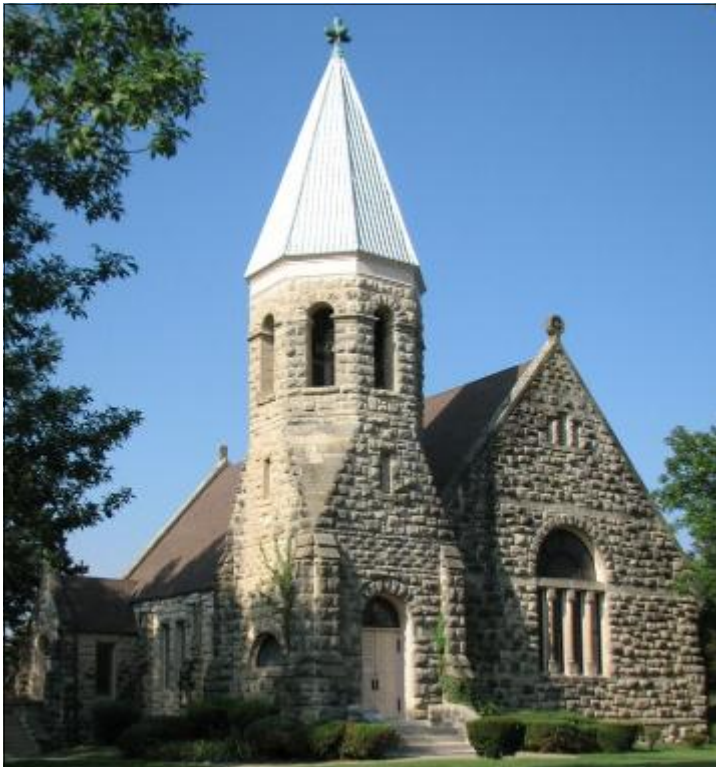
Chapel Fort Riley, Kansas Photo courtesy of Fort Riley Public Works, Conservation and Restoration Branch
