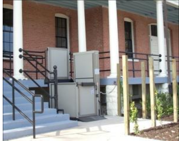
The impact of chair lifts can be softened with a vegetative screen such as the use of vines. Fort Sam Houston, Texas
