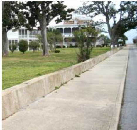
Sidewalks can add to the historic character of a designed streetscape. Naval Air Station Pensacola, Florida
