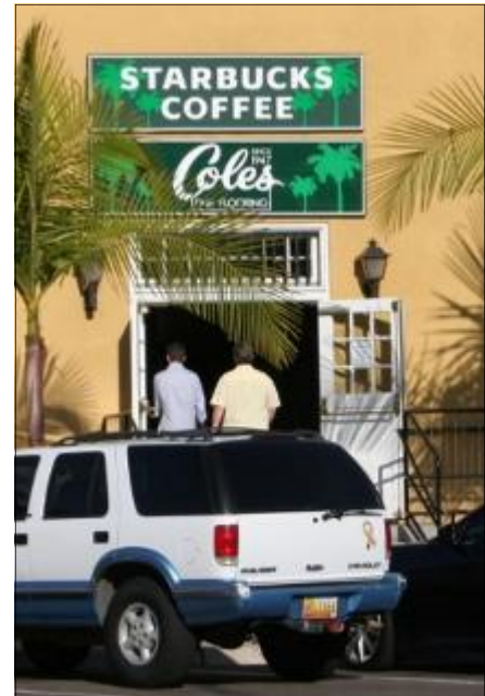
Example of new signage designed to be compatible with the character of a historic building. Marine Corps Recruit Depot, San Diego, California
