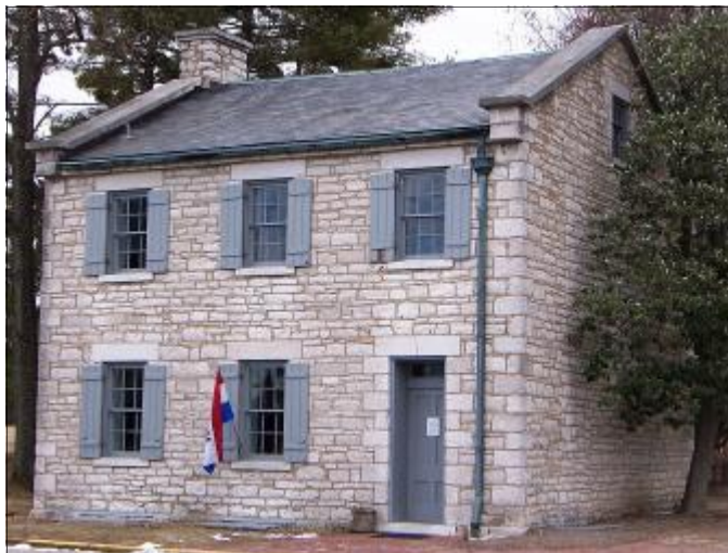
Former military Laborer's House, Jefferson Barracks, Missouri Photo courtesy of ERDC-CERL
