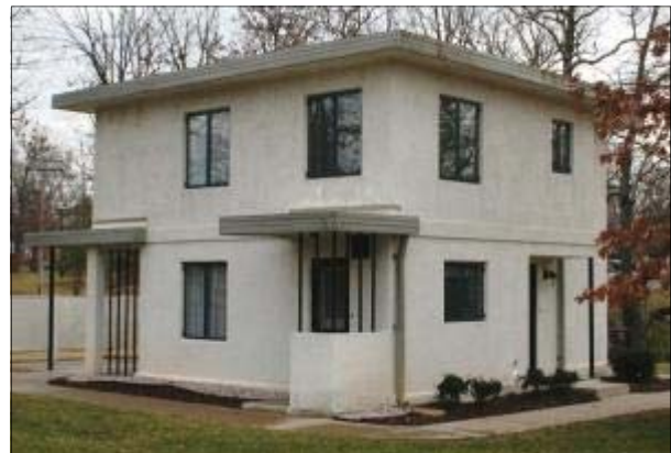
Flat (with eaves) roof shape, Fort Belvoir, Virginia
