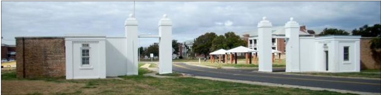
Historic wall and gate contributes to the historic character of the shipyard at the Naval Air Station Pensacola, Florida
