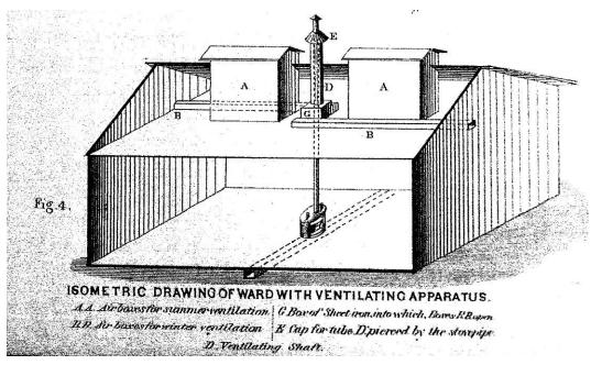
Figure 115. Isometric drawing of a ventilating a typical ward for the Circular #10 hospitals (NARA Washington, DC, RG 112, Entry 63, Box 3).
