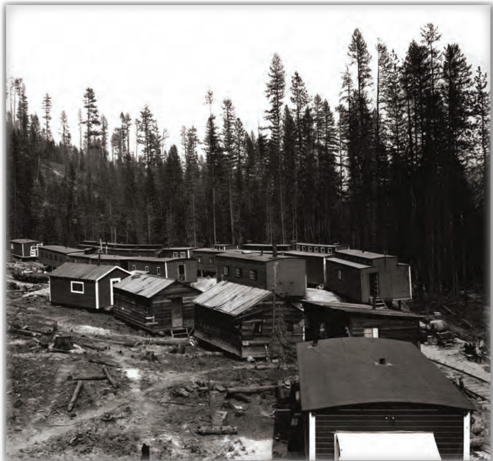
Example of a Portable Lumber Camp. Montana, Unknown Date (U.S. Forest Service).
