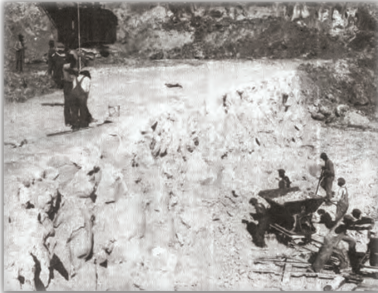
Mining Operation at the Albion Kaolin Company Site Near Hephzibah, Georgia. The men atop the vertical cut appear to be preparing to pry off a fresh face. Unknown Date (Burgess 1985).
