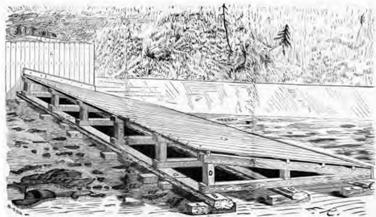
Hollow Frame Dam
