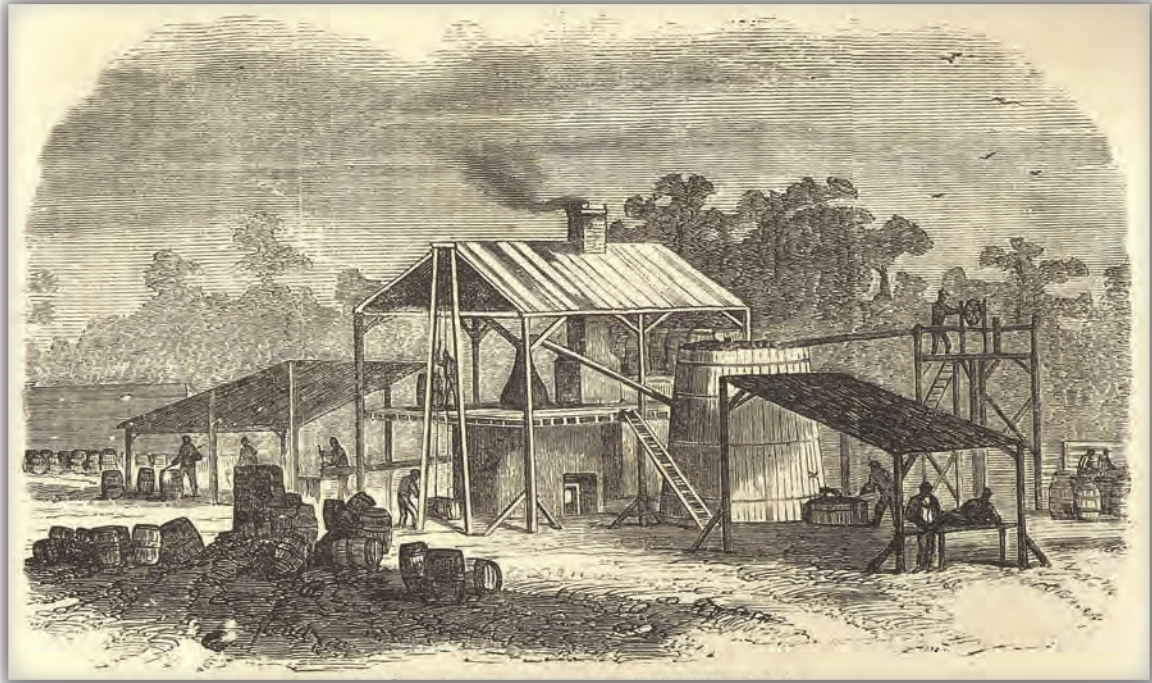
Activities Associated With Turpentine Distilling (courtesy of Fort Bragg Department of Public Works).
