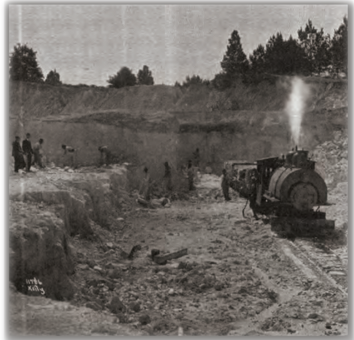
Bauxite Lens Exposed at the top of a Kaolin Mine, Georgia, circa 1920s (Stull 1920).
