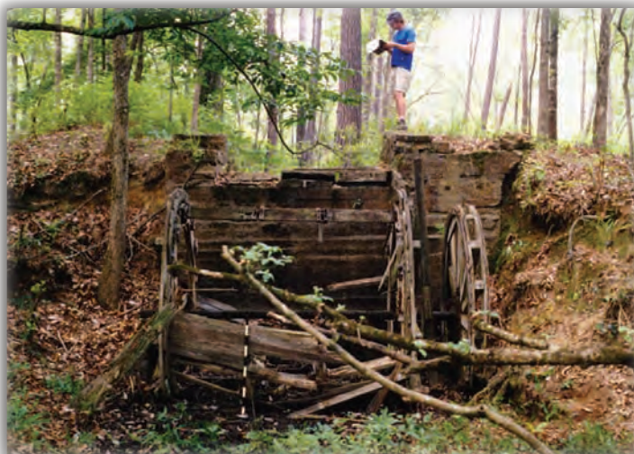
Overshot Wheel, Woodruff Mill (Site 9CE1735), Fort Benning, Chattahoochee County, Georgia (Cowie 2000).
