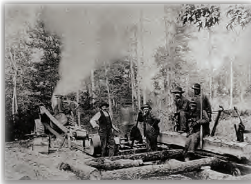
Portable Sawmill Showing the Circular Saw, Steam Engine, and Belting System. Newton County, Georgia, unknown date (Georgia Archives).
