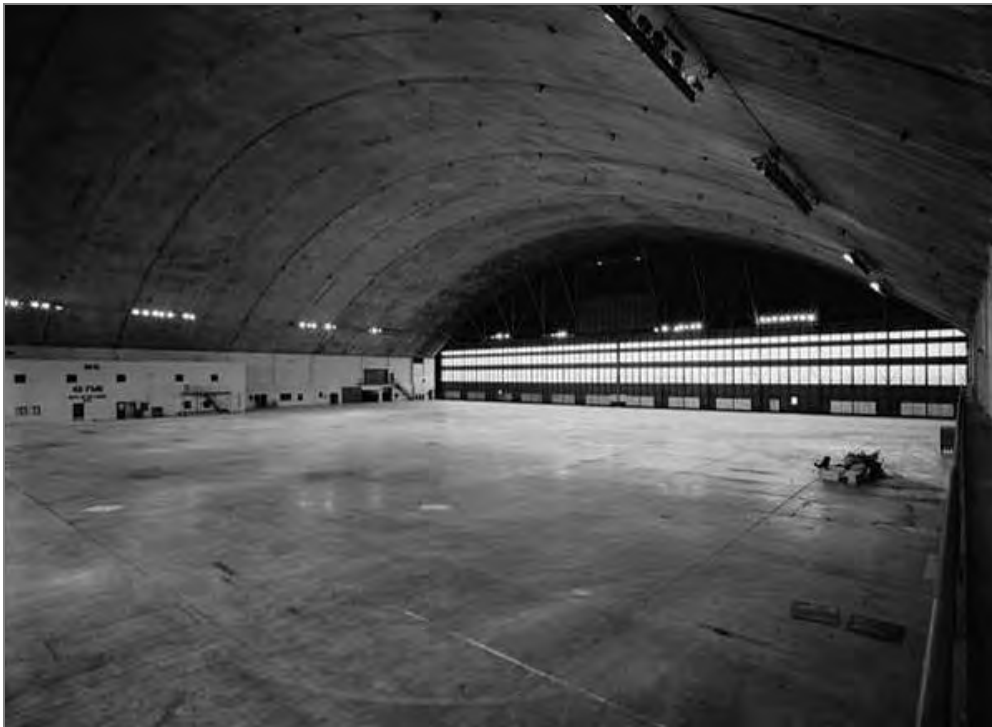
FIGURE 5-2. INTERIOR OF LORING AFB CONCRETE HANGAR
