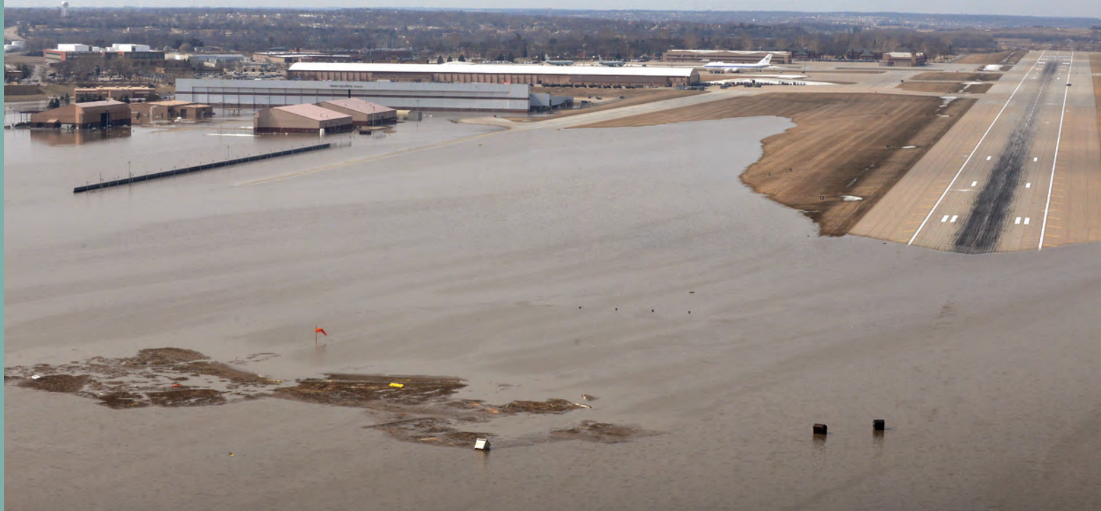
Flooding from the 2019 “bomb cyclone” inundates portions of Offutt Air Force Base, headquarters of the U.S. Strategic Command. Photo: TSgt. Rachelle Blake/USAF.
