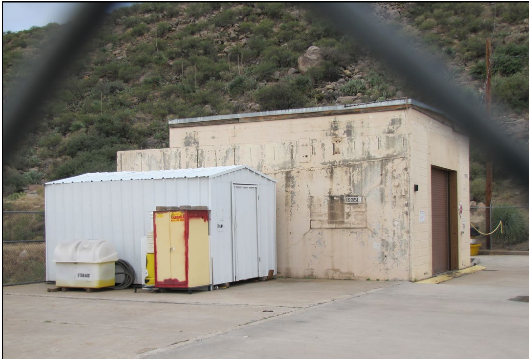
Figure 404. Building 19351 (concrete block) and no number (metal) at WSMR (ERDC-CERL 2016).
