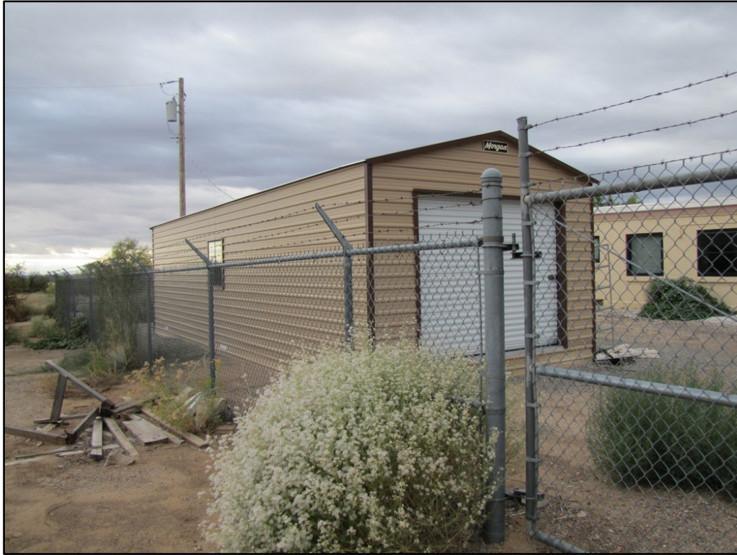
Figure 446. No Number at WSMR (ERDC-CERL 2016).
