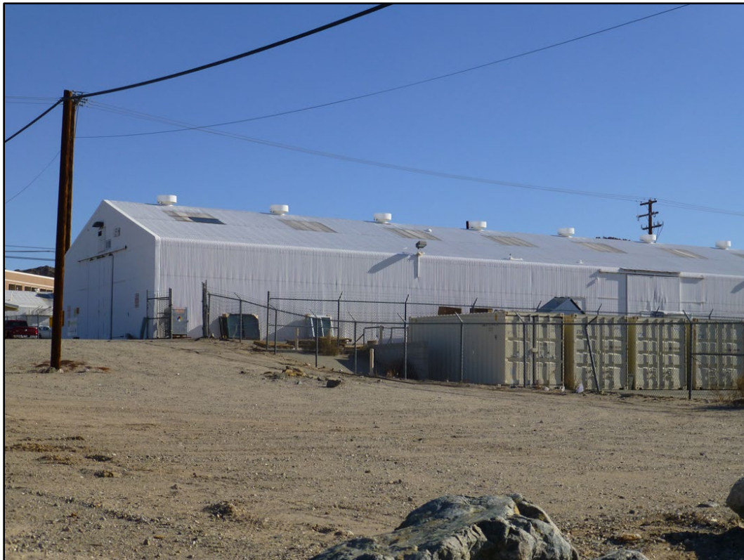
Figure 296. Building 1118 at MCAGCC Twentynine Palms (ERDC-CERL 2016).
