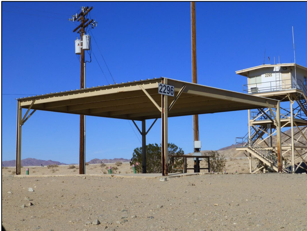
Figure 308. Building 2296 at MCAGCC Twentynine Palms (ERDC-CERL 2016).
