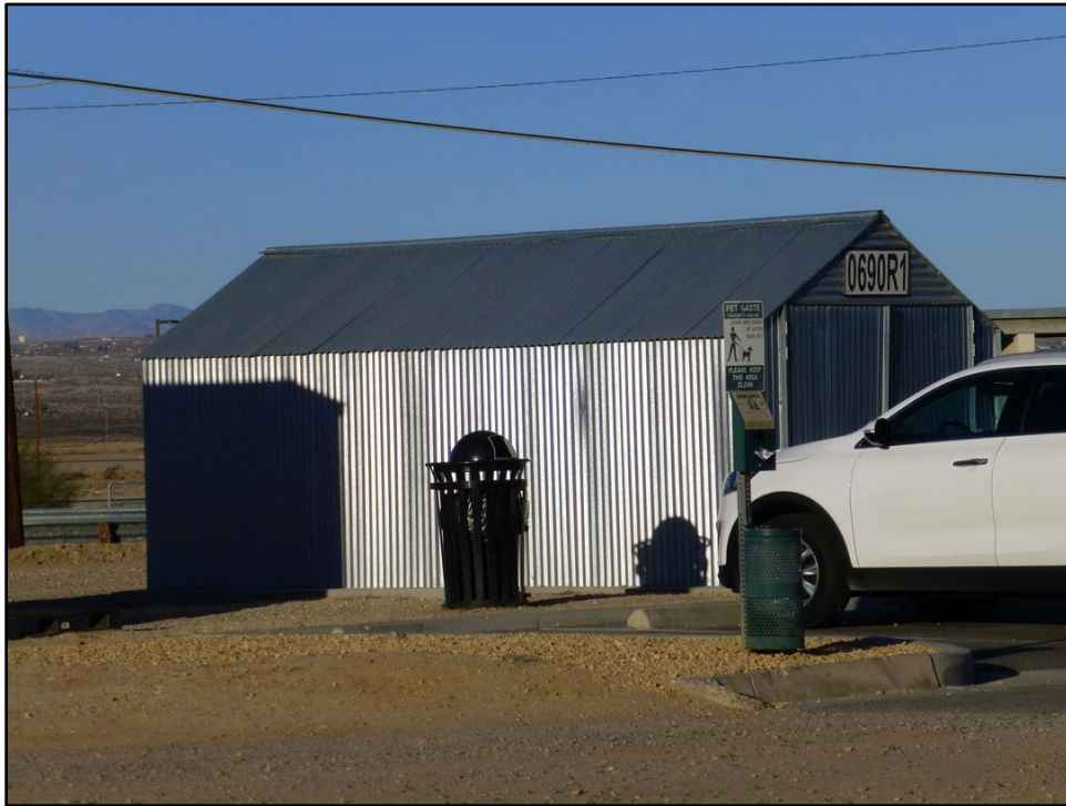
Figure 218. Building 0690R1 at MCAGCC Twentynine Palms (ERDC-CERL 2016).
