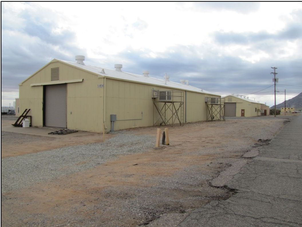
Figure 397. Buildings 1852 and 1854 at WSMR (ERDC-CERL 2016).
