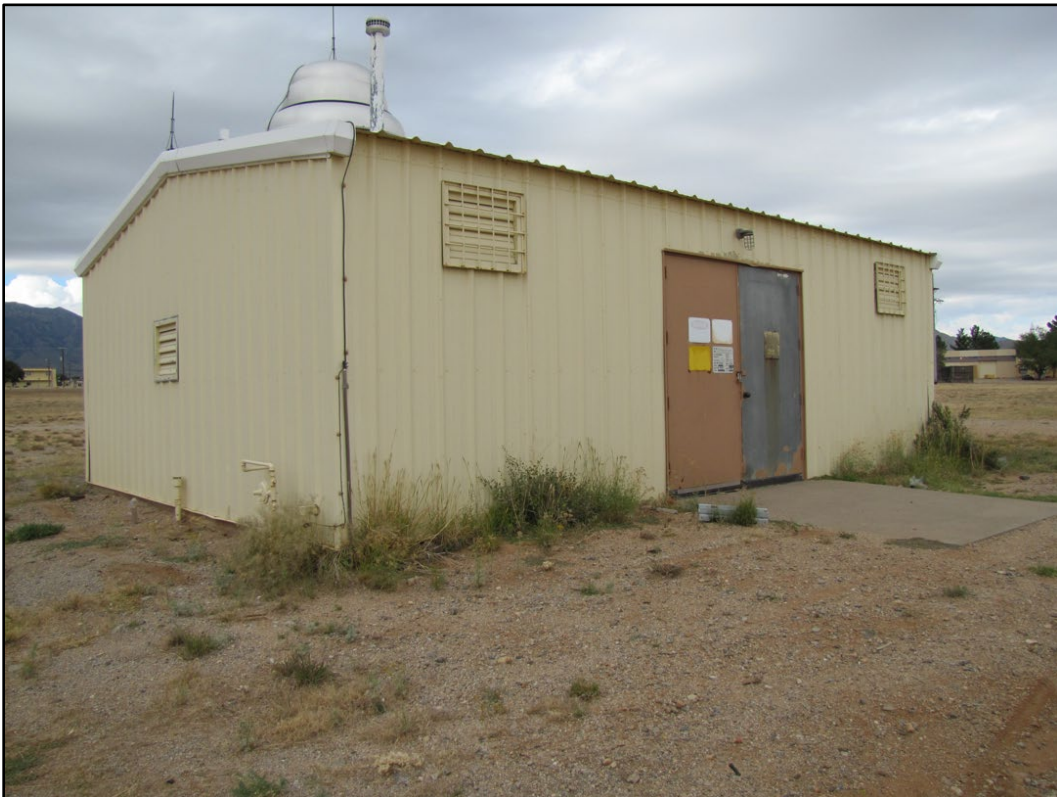
Figure 387. Building 302A at WSMR (ERDC-CERL 2016).
