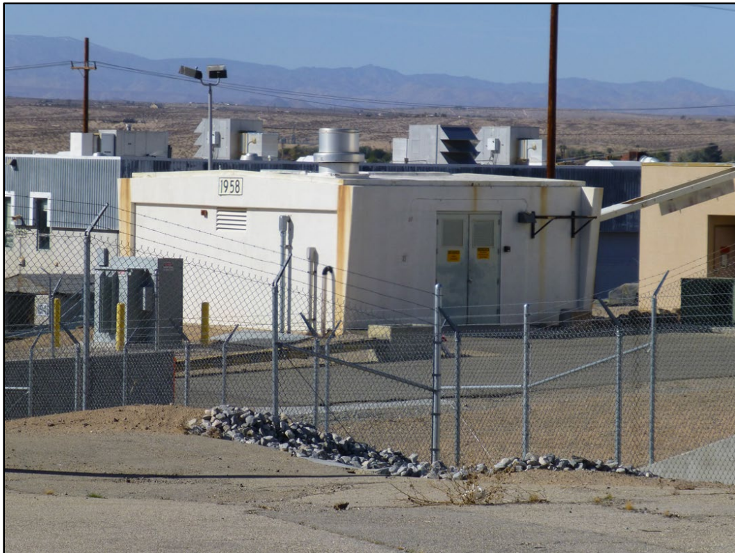
Figure 306. Building 1958 at MCAGCC Twentynine Palms (ERDC-CERL 2016).
