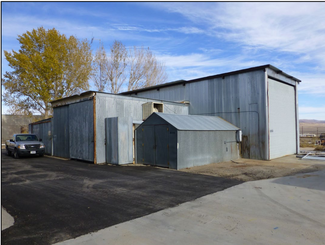
Figure 360. Buildings 10857 and 10858 at NAWS China Lake (ERDC-CERL 2016).
