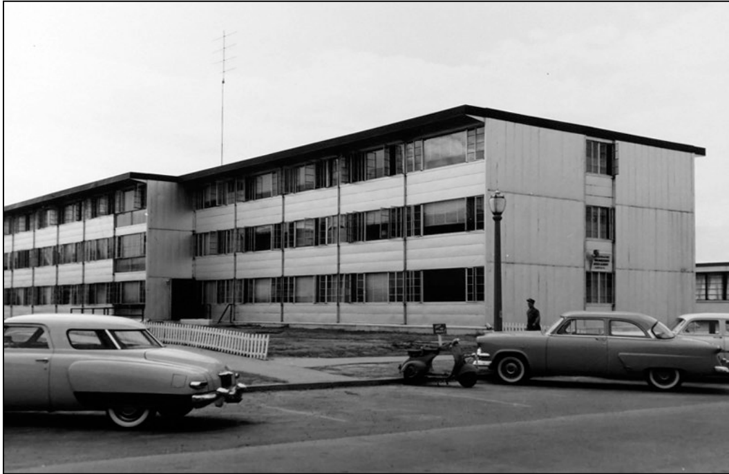
Figure 119. Exterior of a prefabricated metal barracks used as the Non-Commissioned Officers' Training Academy, Barksdale AFB, Louisiana, 1955 (NARA College Park, RG342-B).
