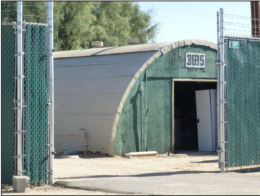
Figure 313. Building 3815 at MCAGCC Twentynine Palms (ERDC-CERL 2016).
