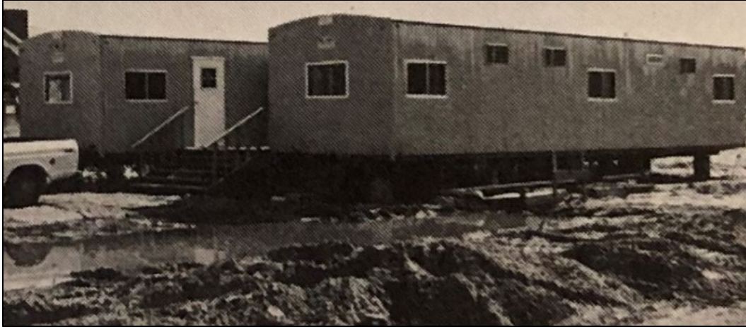
Figure 185. An arched-roofed modular clean-room manufactured by Williams Mobile Offices. It had toilets, showers, lockers, HVAC systems, and an air filtration system, 1984 (Williams Mobile Offices, "The company behind these buildings is Williams," The Military Engineer 76, no. 492 (March–April 1984): 129).
