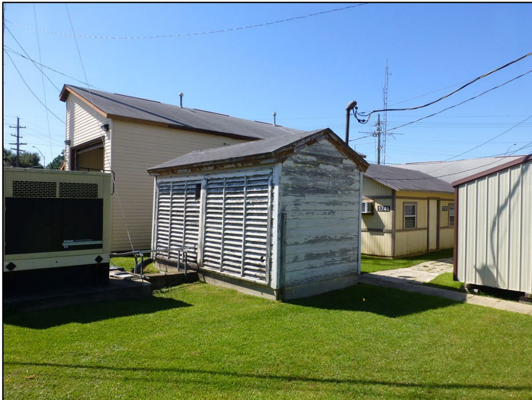
Figure 287. No Number at Fort Polk (ERDC-CERL 2016).
