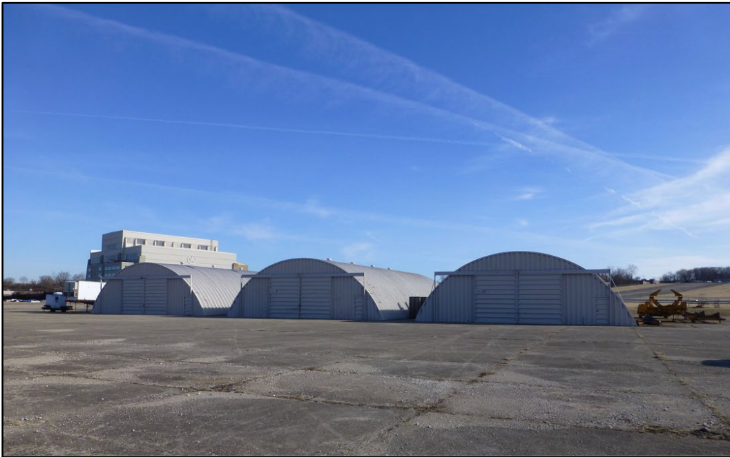
Figure 239. Buildings 107 (right), 111 (middle), and No Number (left) at Wright–Patterson AFB (ERDC-CERL 2017).
