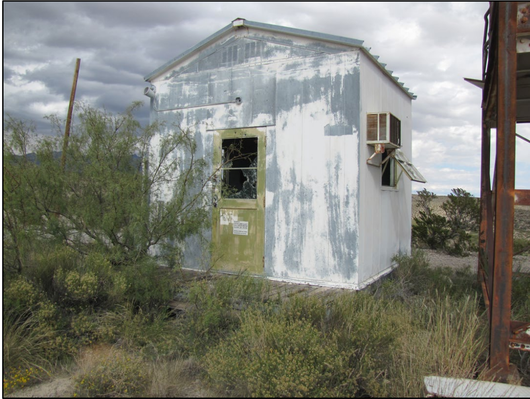
Figure 434. No Number at WSMR (ERDC-CERL 2016).
