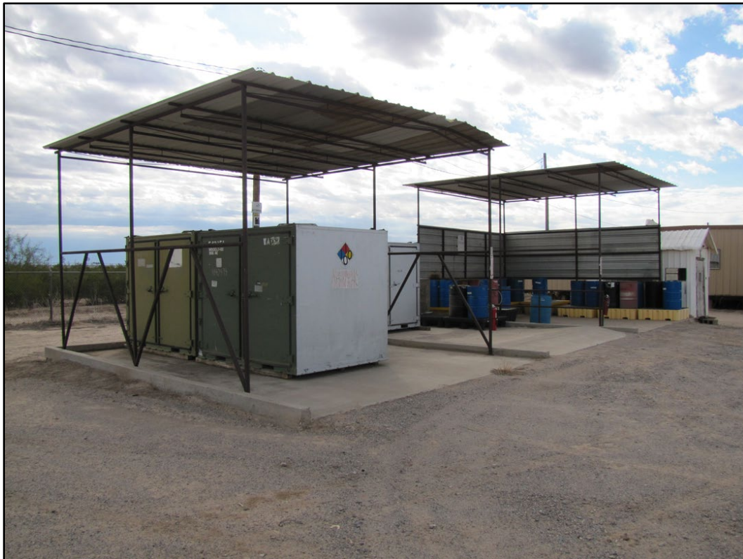
Figure 431. No Numbers at WSMR (ERDC-CERL 2016).
