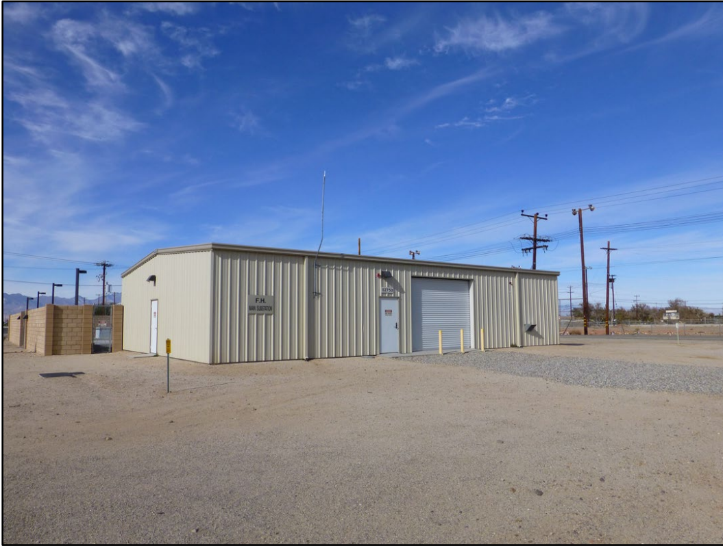
Figure 355. Building 02750 at NAWS China Lake (ERDC-CERL 2016).
