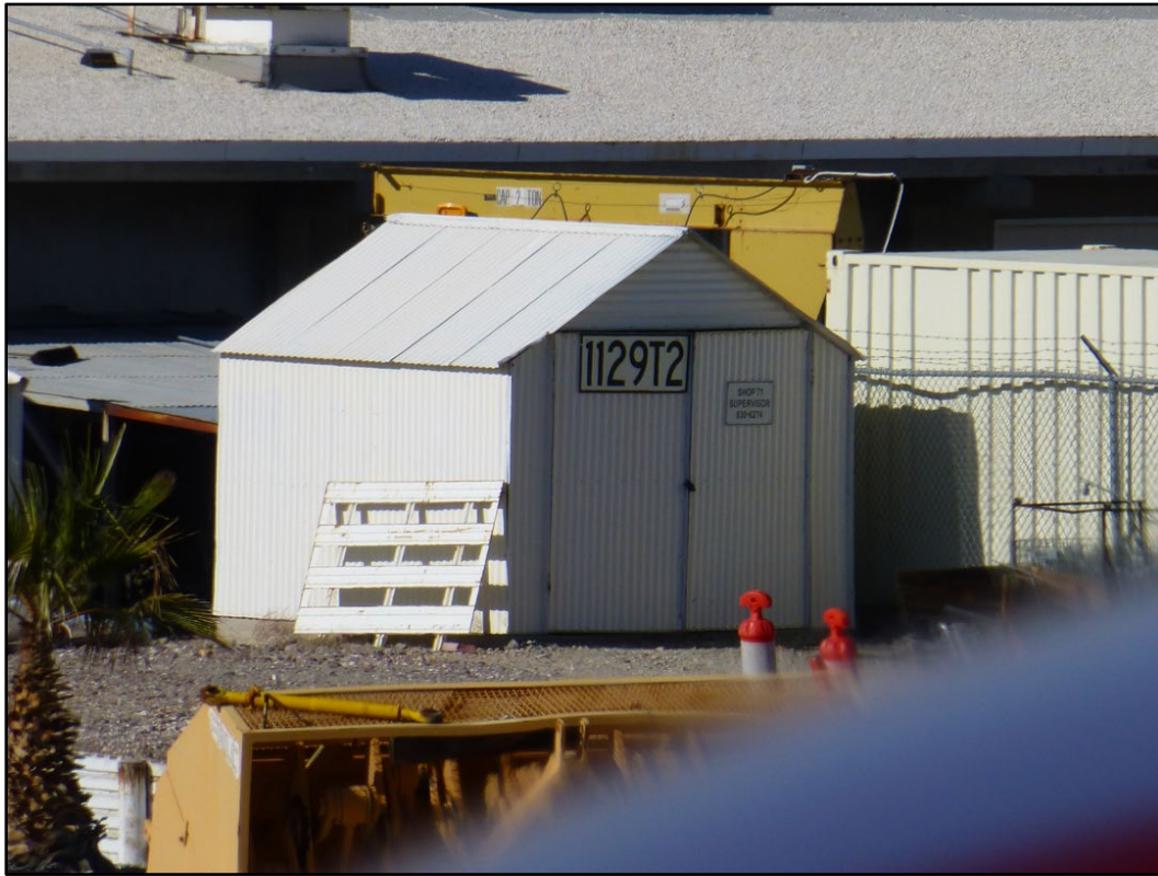
Figure 299. Building 1129T2 at MCAGCC Twentynine Palms (ERDC-CERL 2016).
