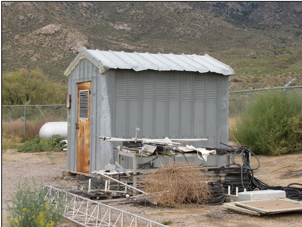
Figure 445. Building No Number at WSMR (ERDC-CERL 2016).
