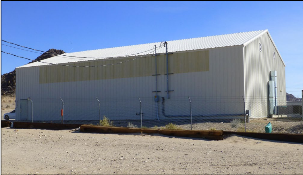
Figure 321. No Number at MCAGCC Twentynine Palms (ERDC-CERL 2016).
