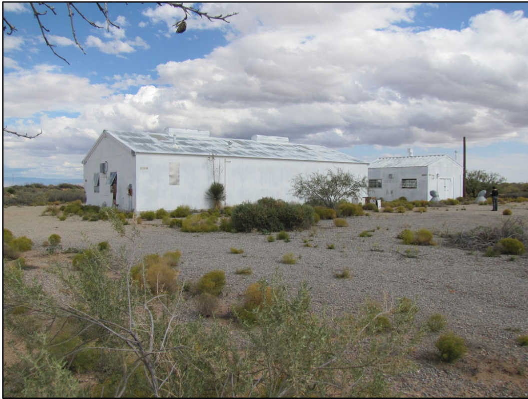
Figure 416. Buildings 23514 (left) and 23511 (right) at WSMR (ERDC-CERL 2016).
