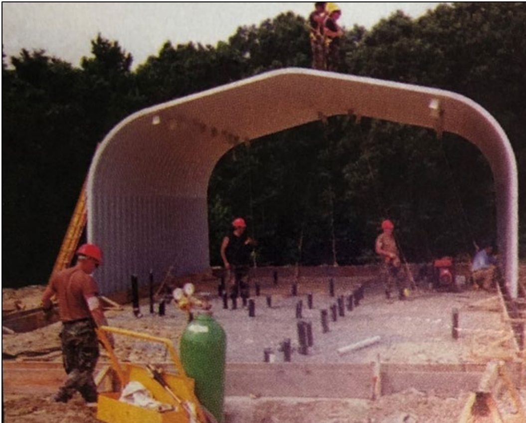
Figure 198. One of four ABMs erected by the Air National Guard using the UBM-2000 at their Regional Training Center, North Carolina, 1997 ("New UBM," The Military Engineer 89, no. 582 (Jan. 1997): 346).
