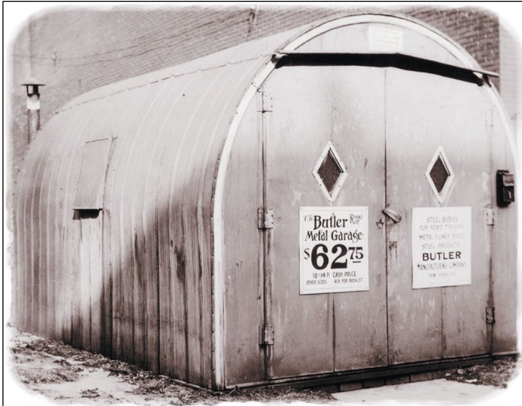
Figure 3. The first model of corrugated metal garages sold by Butler, 1909 (Butler Manufacturing Company, “Built By Hand, Backed By Experience,” About, accessed August 20, 2021, https://www.butlermfg.com/about/ ).
