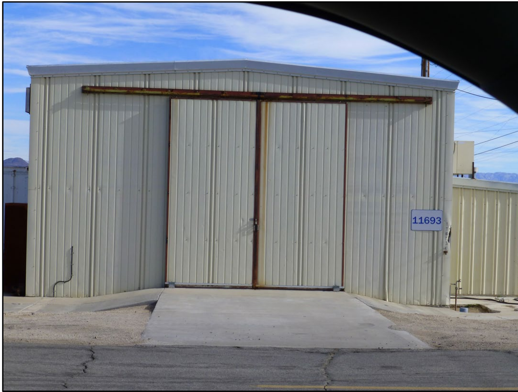
Figure 369. Building 11693 at NAWS China Lake (ERDC-CERL 2016).
