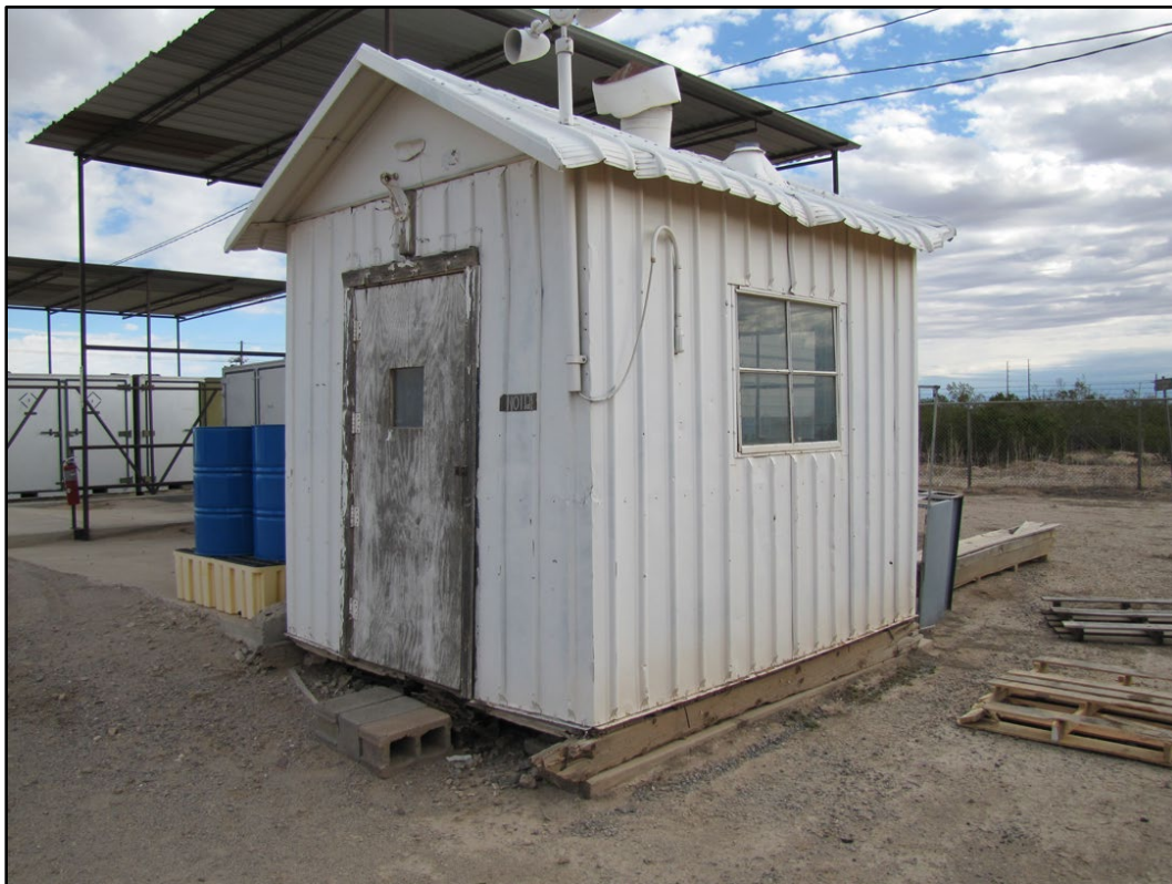
Figure 232. Building 1128 at WSMR (WSMR 2016).
