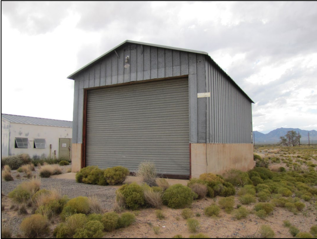
Figure 438. No Number at WSMR (ERDC-CERL 2016).
