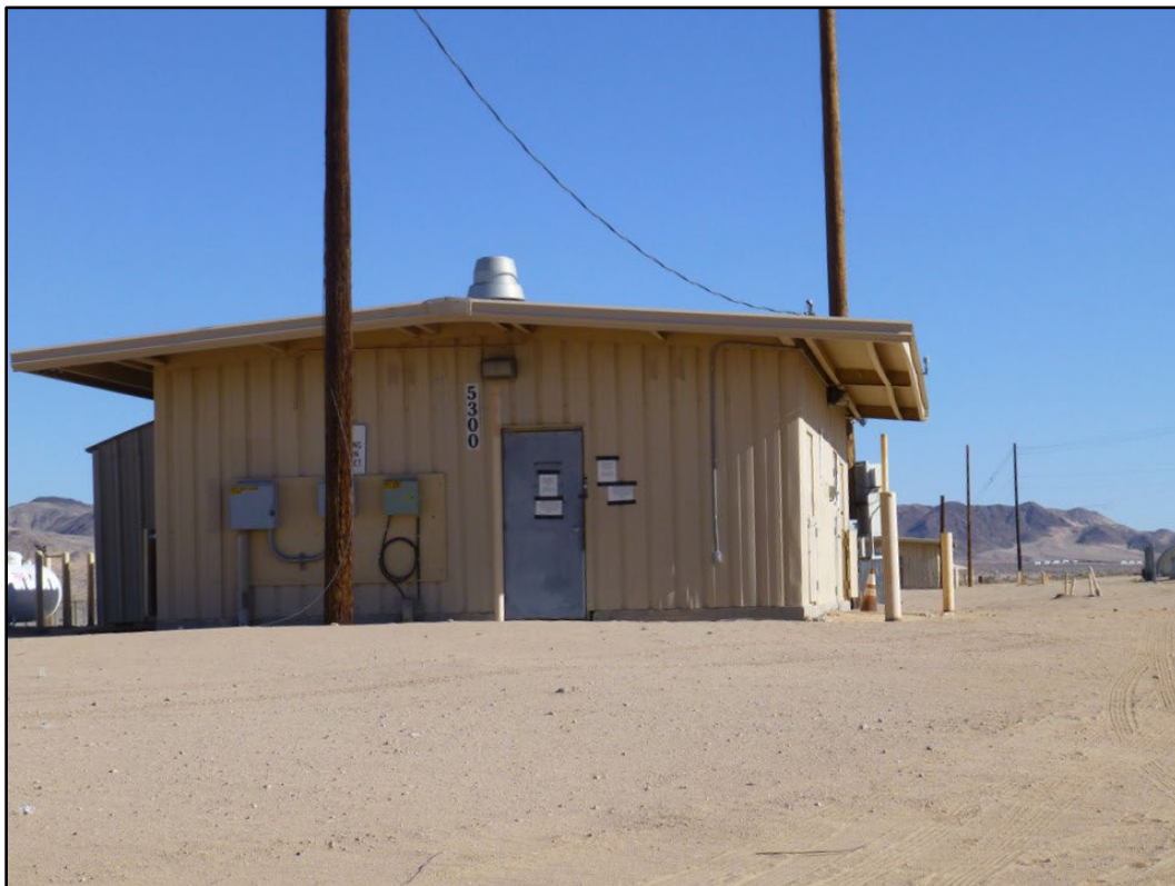
Figure 314. Building 5300 at MCAGCC Twentynine Palms (ERDC-CERL 2016).
