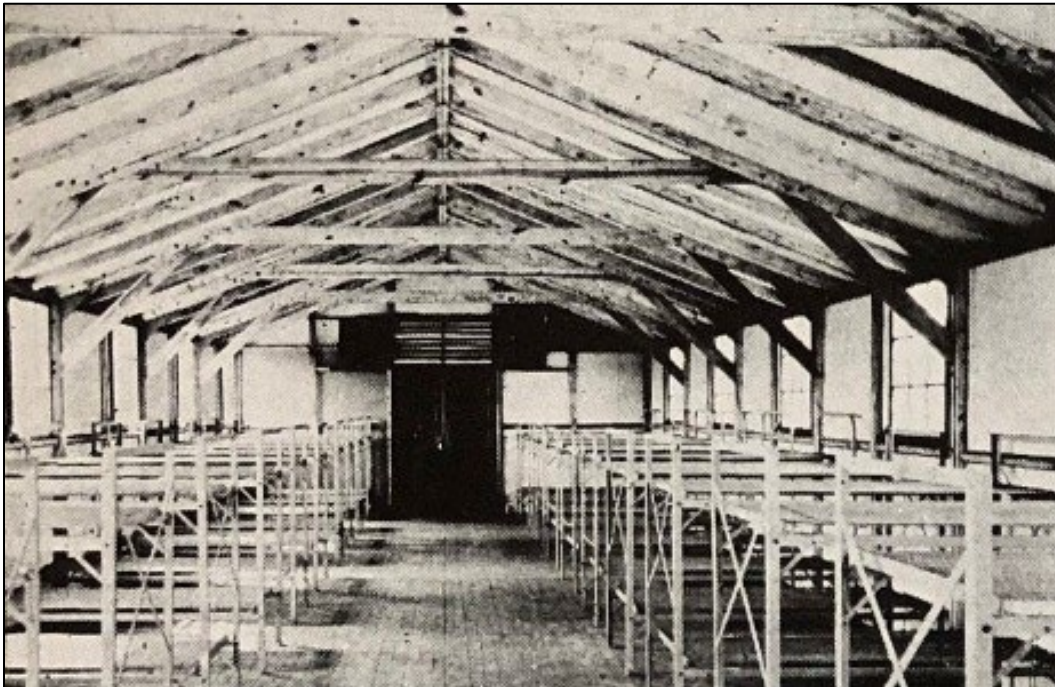
Figure 41. The interior of a fully completed Bush Type-B building with rows of bunkbeds along each side, November 1943 (Clinton G. Bush Co., "Bush Housing for Labor," Prefabricated Homes 1-5 (Nov. 1943): 6).
