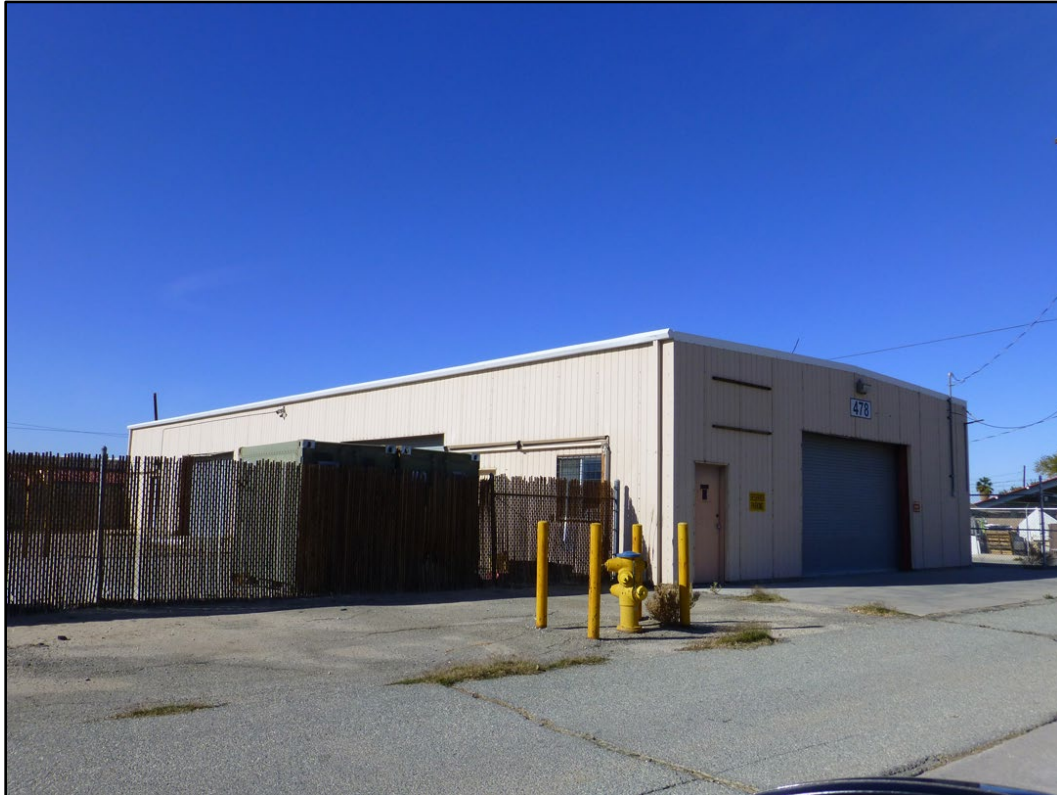
Figure 217. Building 478 at MCAGCC Twentynine Palms (ERDC-CERL 2016).
