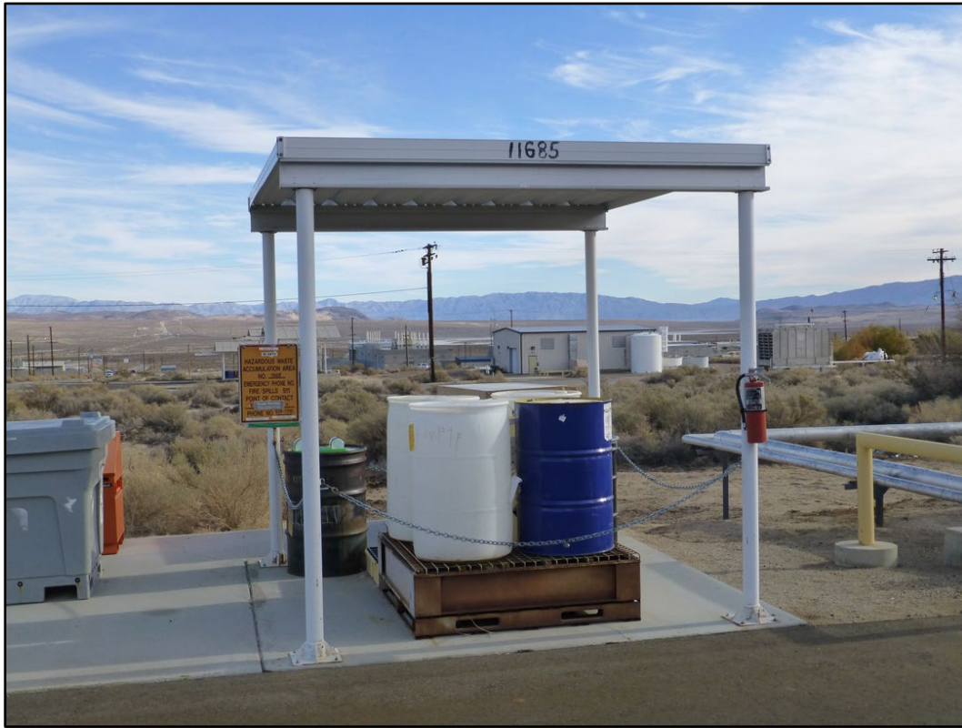
Figure 367. Building 11685 at NAWS China Lake (ERDC-CERL 2016).
