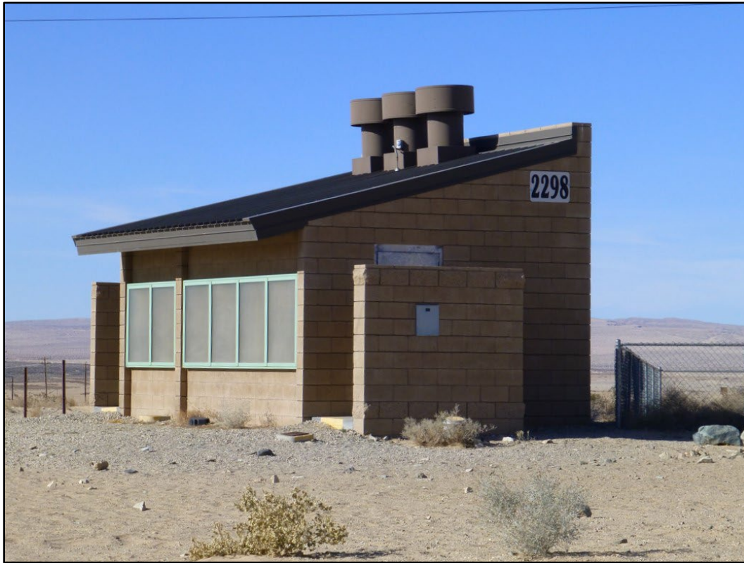
Figure 311. Building 2298 at MCAGCC Twentynine Palms (ERDC-CERL 2016).
