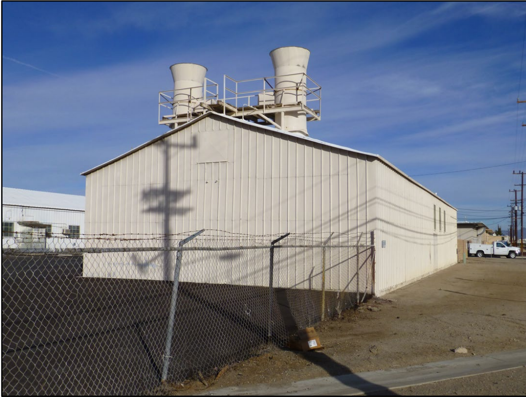
Figure 339. Building 00576 at NAWS China Lake (ERDC-CERL 2016).
