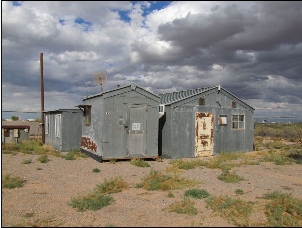
Figure 442. No Numbers at WSMR (ERDC-CERL 2016).
