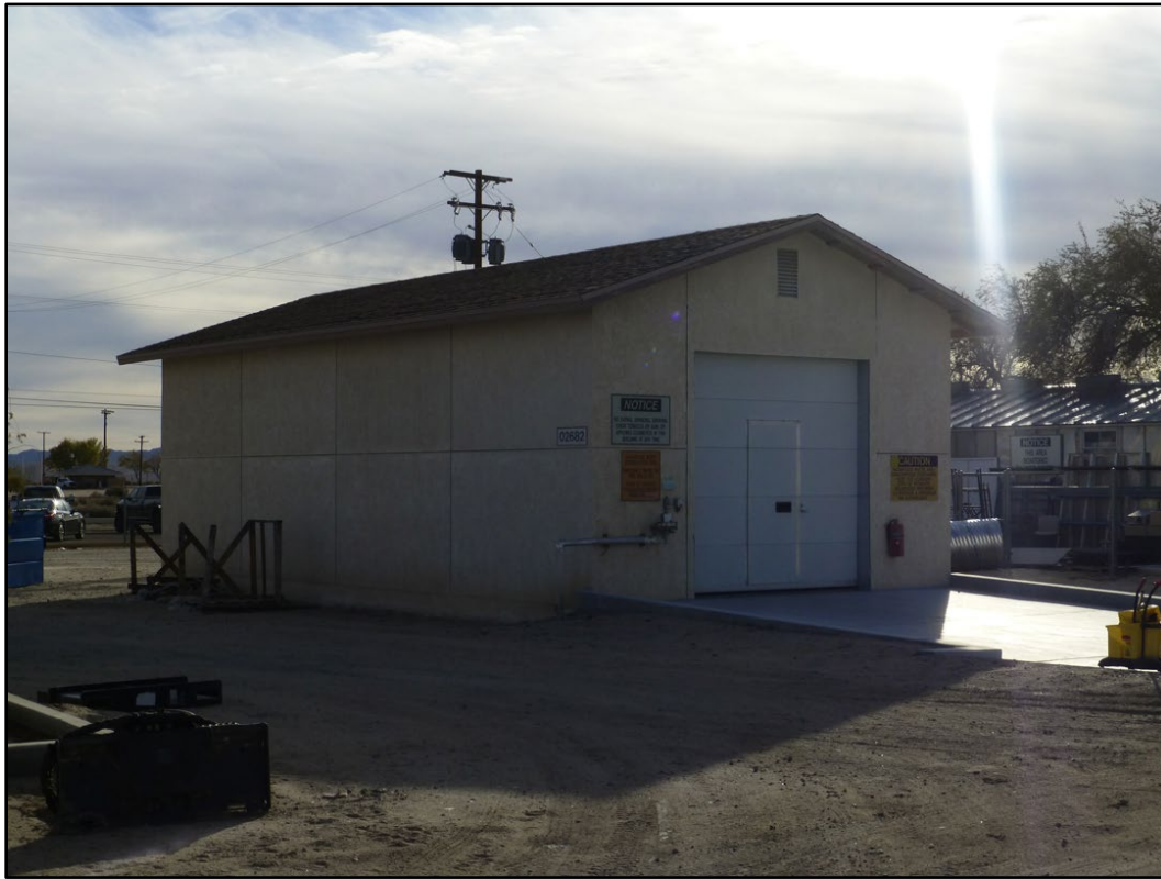
Figure 353. Building 02682 at NAWS China Lake (ERDC-CERL 2016).
