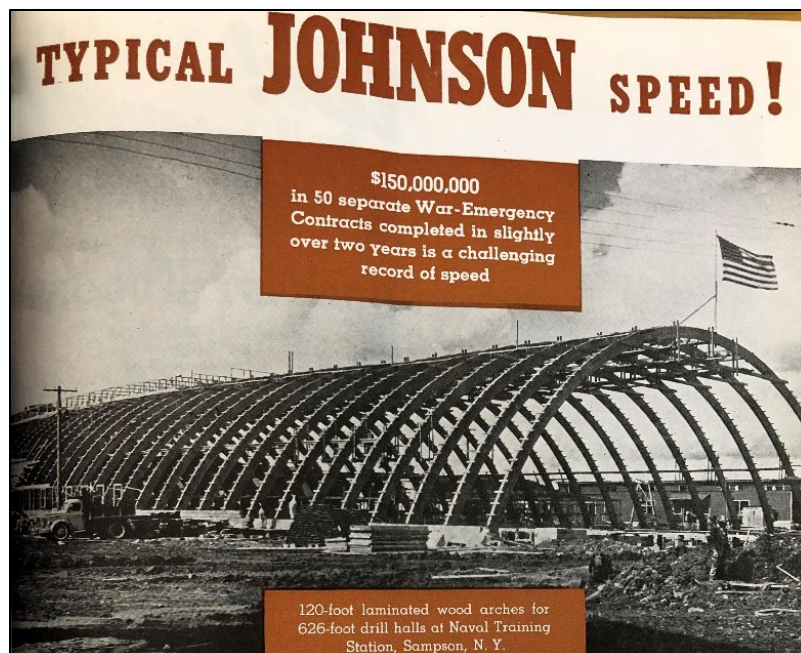
Figure 57. One of the six large naval drill halls constructed by Johnson using wooden laminated arches with horizontal connection pieces preinstalled on the arch before erection to speed production, Sampson Naval Station, New Jersey, 1944 (John A. Johnson Contracting Corporation, “War speed is typical Johnson Speed!” Prefabricated Homes 1-5 (Feb. 1944): n.p.).
