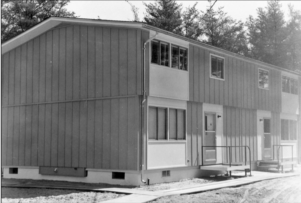
Figure 158. A recently erected duplex that cost between $10,000 and $11,000 to construct, with each unit featuring three bedrooms, a dining/living room, a kitchen, and one-and-one-half baths, Andrews AFB, Maryland, 1964 (NARA College Park, RG342-B).
