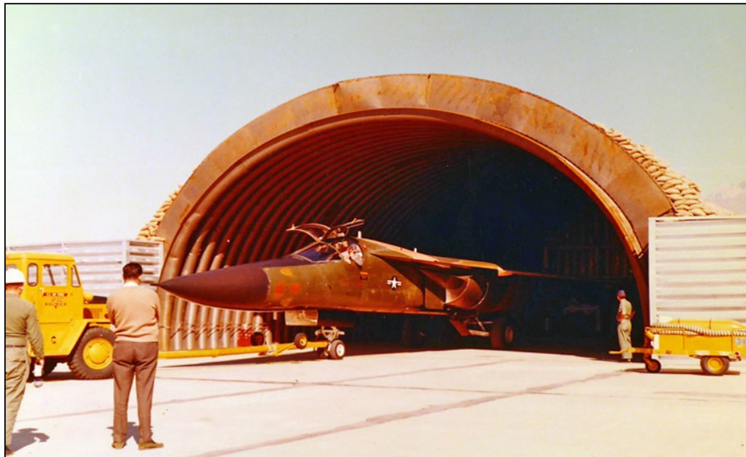
Figure 171. A prototype of a protective aircraft structure being tested by the Air Force at Holloman AFB, Otero County, New Mexico, Feb. 1968 (NARA College Park RG 342-B).
