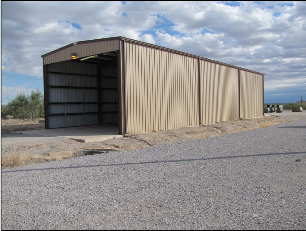
Figure 432. No Number at WSMR (ERDC-CERL 2016).
