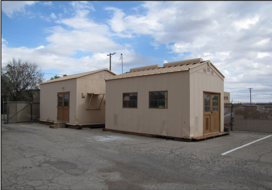
Figure 448. No Numbers at WSMR (ERDC-CERL 2016).
