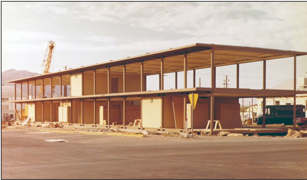
Figure 164. Modular barracks under construction, Nellis AFB, Nevada, 1968 (NARA College Park, RG342-B).
