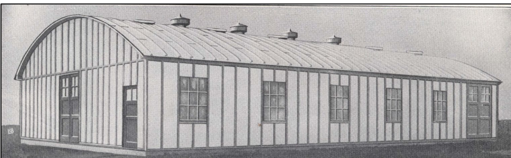
Figure 11. A Mesker prefabricated building being used as a warehouse featuring large loading doors, personnel doors, skylights, and significant ventilation, Two Rivers, WI, 1928 (Geo. L. Mesker & Company, "Mesker store fronts and metal building products," Evansville, IN: Geo. L. Mesker Steel Corporation, 1928. https://archive.org/details/GeoLMeskerstorefrontsandmetalbuilding0001/ , 16).
