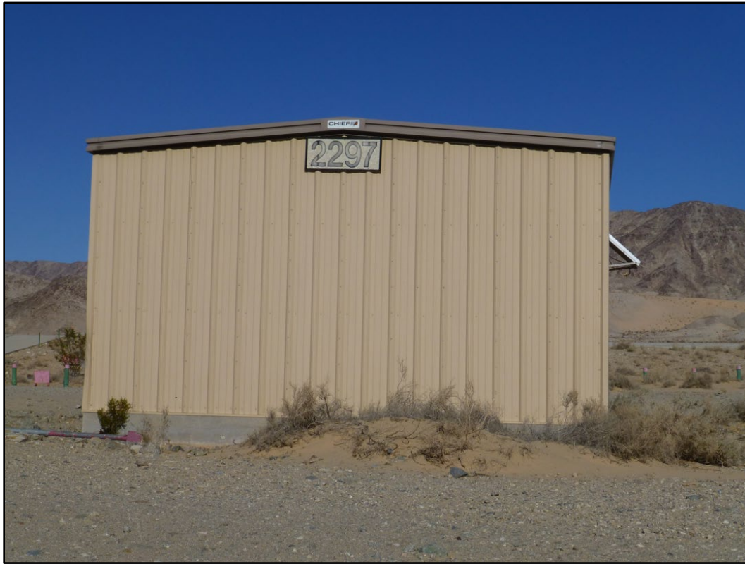
Figure 309. Building 2297 at MCAGCC Twentynine Palms (ERDC-CERL 2016).
