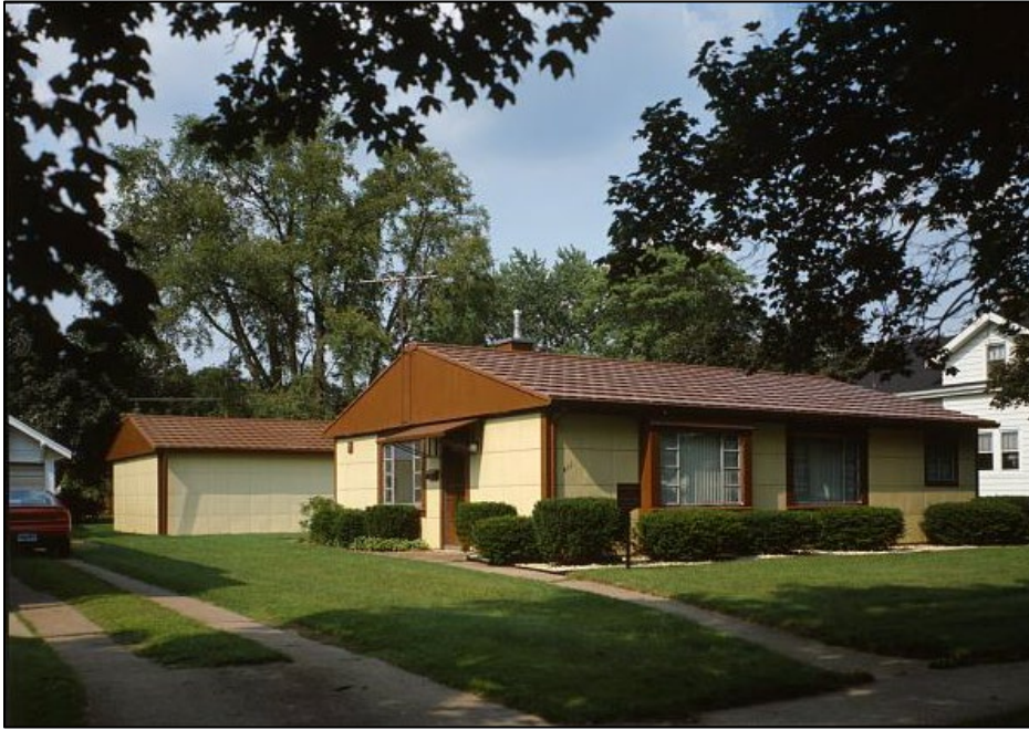
Figure 127. Oblique of a Lustron house in Chesterton, Indiana, constructed in 1950 (Library of Congress HABS IND,64-CHEST,1-).
