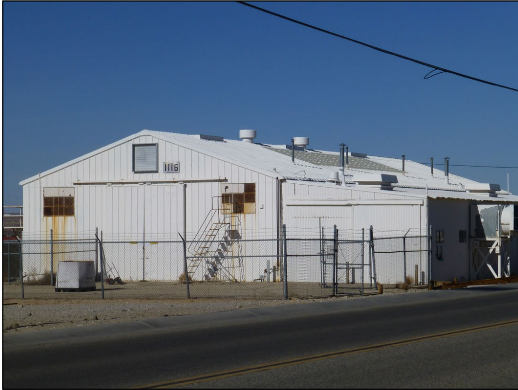
Figure 295. Building 1116 at MCAGCC Twentynine Palms (ERDC-CERL 2016).
