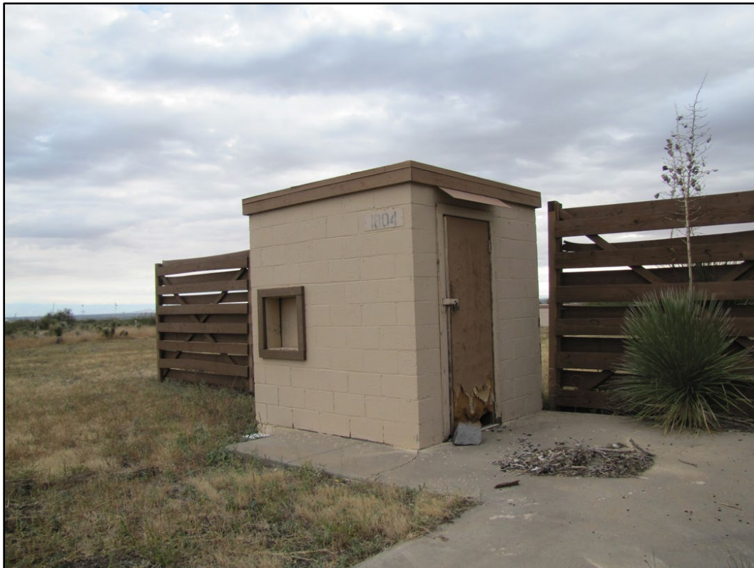
Figure 395. Building 1804 at WSMR (ERDC-CERL 2016).
