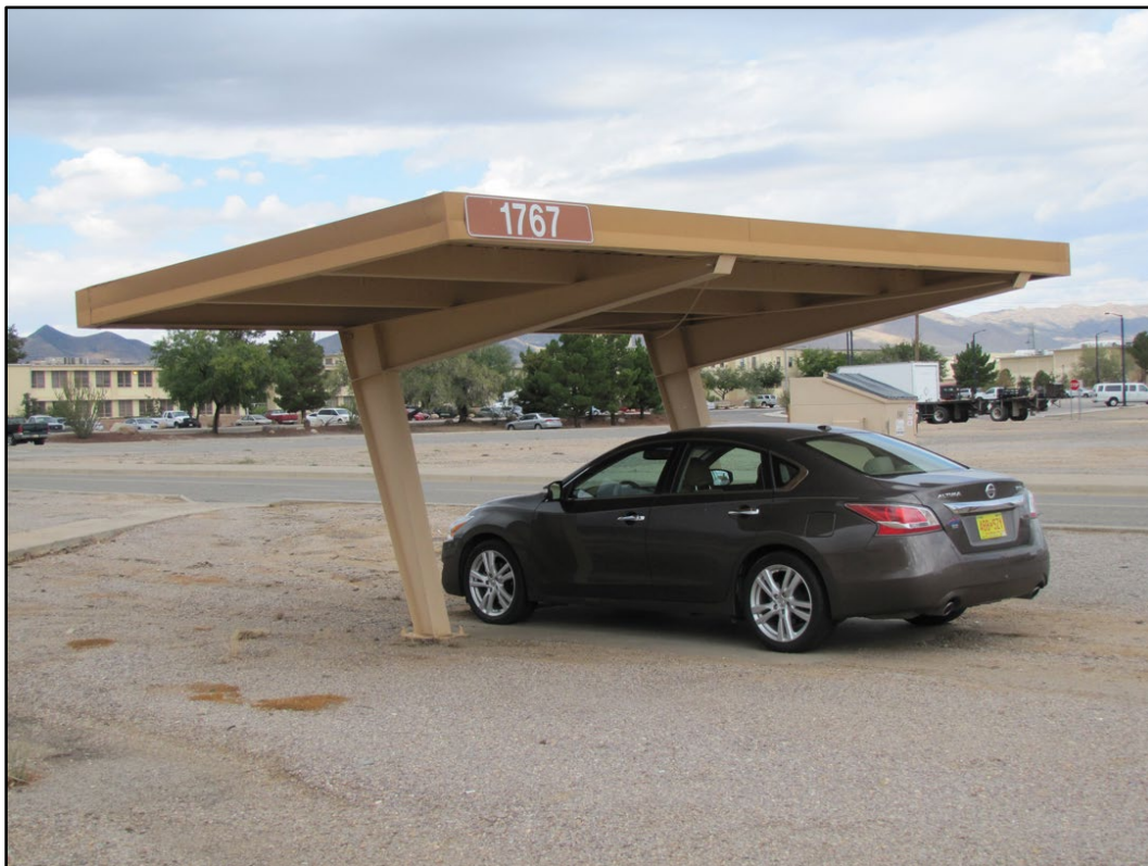
Figure 393. Building 1767 at WSMR (ERDC-CERL 2016).
