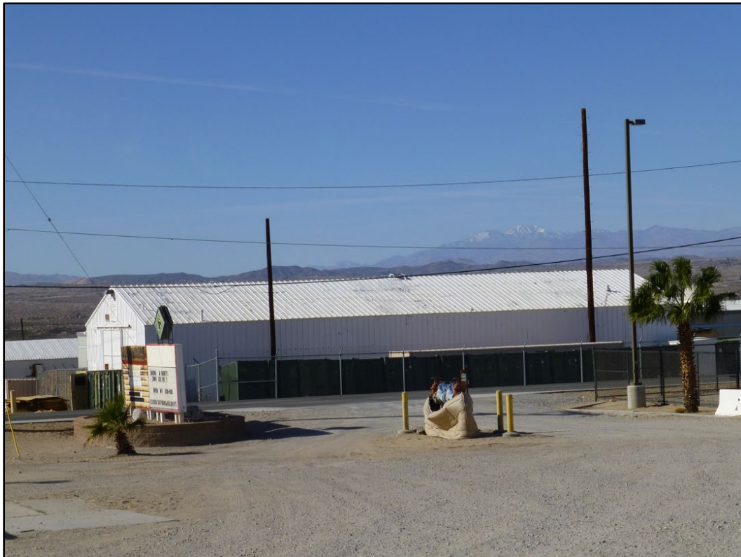
Figure 318. No Number at MCAGCC Twentynine Palms (ERDC-CERL 2016).
