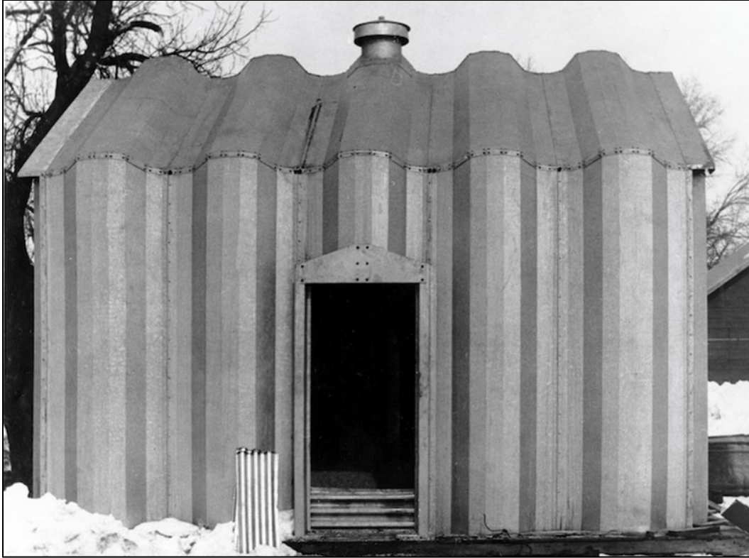
Figure 99. The S-Span was the first self-framing structure manufactured by Behlen Manufacturing of Columbus, Nebraska, 1950 (Behlen Manufacturing Company, "One of Many Firsts," History, accessed December 18, 2018, https://www.behlenmfg.com/history ).
