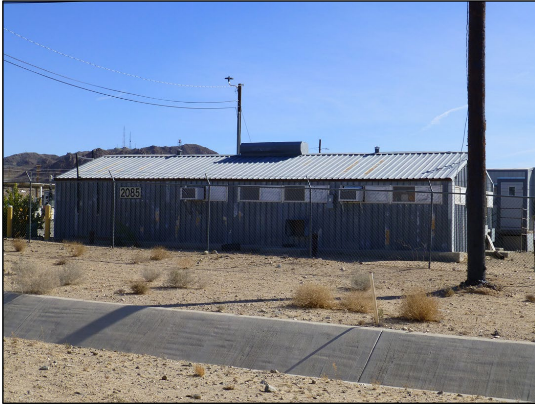
Figure 307. Building 2085 at MCAGCC Twentynine Palms (ERDC-CERL 2016).
