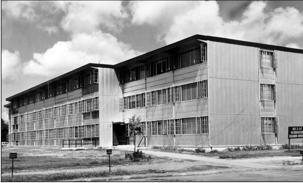
Figure 121. Exterior of a prefabricated metal barracks used as part of the Non-Commissioned Officers' Training Academy as well as housing the Second Air Force Headquarters' Squadron Division, showing the location of the main door on the center portion of the structure, Barksdale AFB, Louisiana, Date Unknown (NARA College Park, RG342-B).
