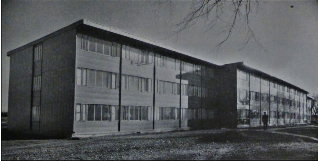
Figure 113. Prefabricated metal barracks, Offutt AFB, Omaha, Nebraska, 1952 ("Airman's Dormitory of prefab steel parts goes up fast, provides more privacy and comfort than old barracks for less money," Magazine of Buildings: House and Home Edition 1, no. 1 (Jan.-March 1952): 154-155).
