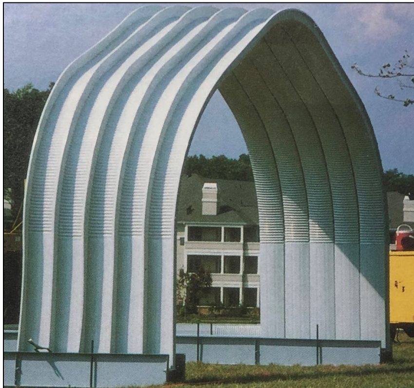
Figure 197. A section constructed using the UBM-2000 as part of a demonstration for "scores of observers representing construction, military, and foreign government sectors," 1993 ("Random Rubble: MIC's UBM-2000," The Military Engineer 85, no. 540 (Nov.-Dec. 1993): 71).
