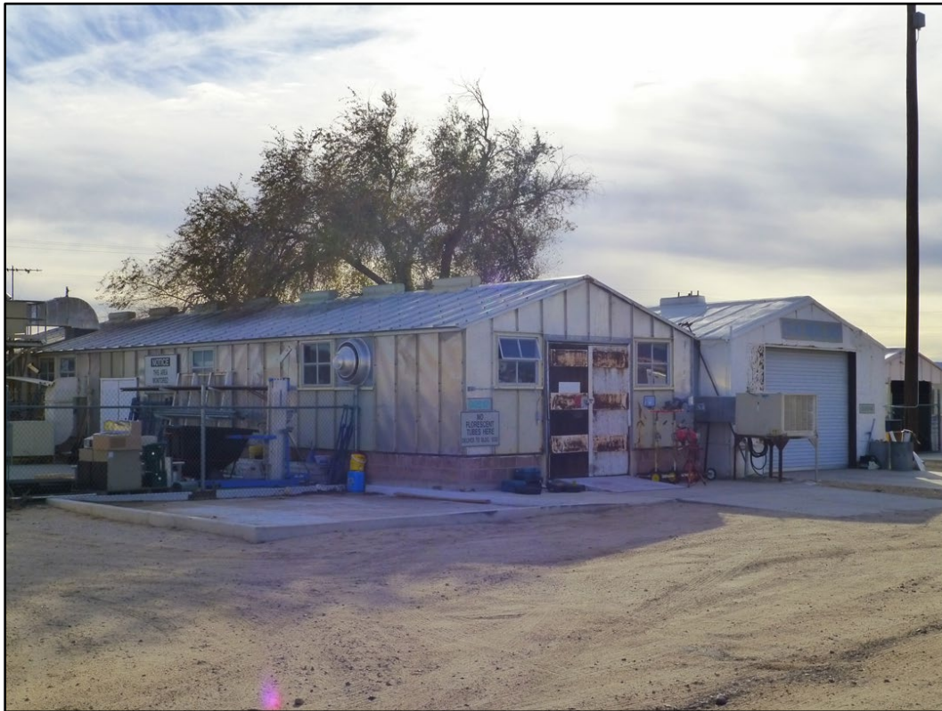
Figure 351. Buildings 02612 (left) and 02614 (right) at NAWS China Lake (ERDC-CERL 2016).
