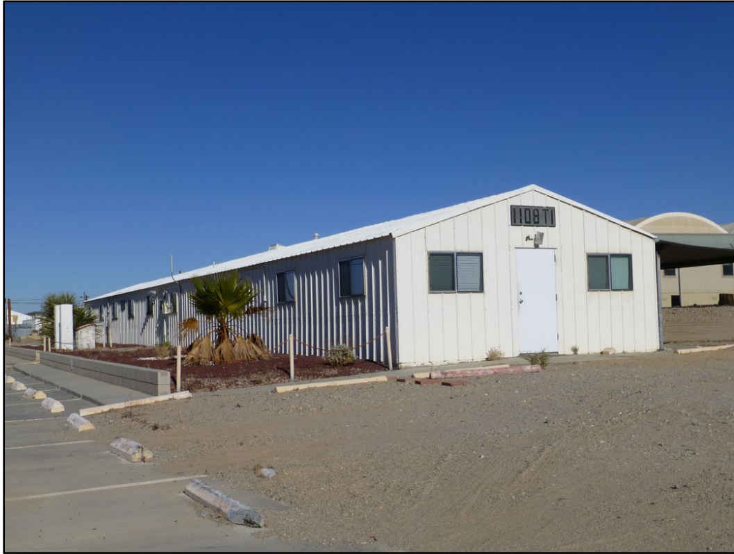
Figure 293. Building 1108T1 at MCAGCC Twentynine Palms (ERDC-CERL 2016).
