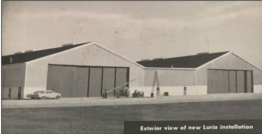
Figure 130. Exterior of two connected “girder-type” Luria Engineering Hangars erected for Bell Aircraft Corporation (Luria Engineering Company, “Bell Aircraft Corporation Chooses Luria Standardized Buildings,” Architectural Forum 102 (Jan.–March 1955): 206).
