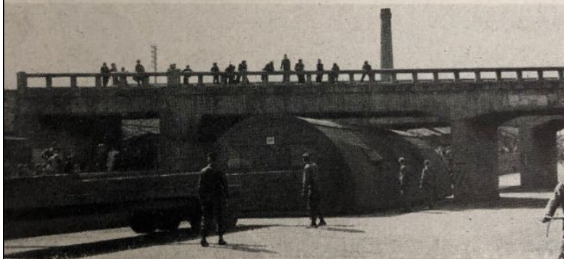
Figure 9. Rolling a Quonset under a Bridge
