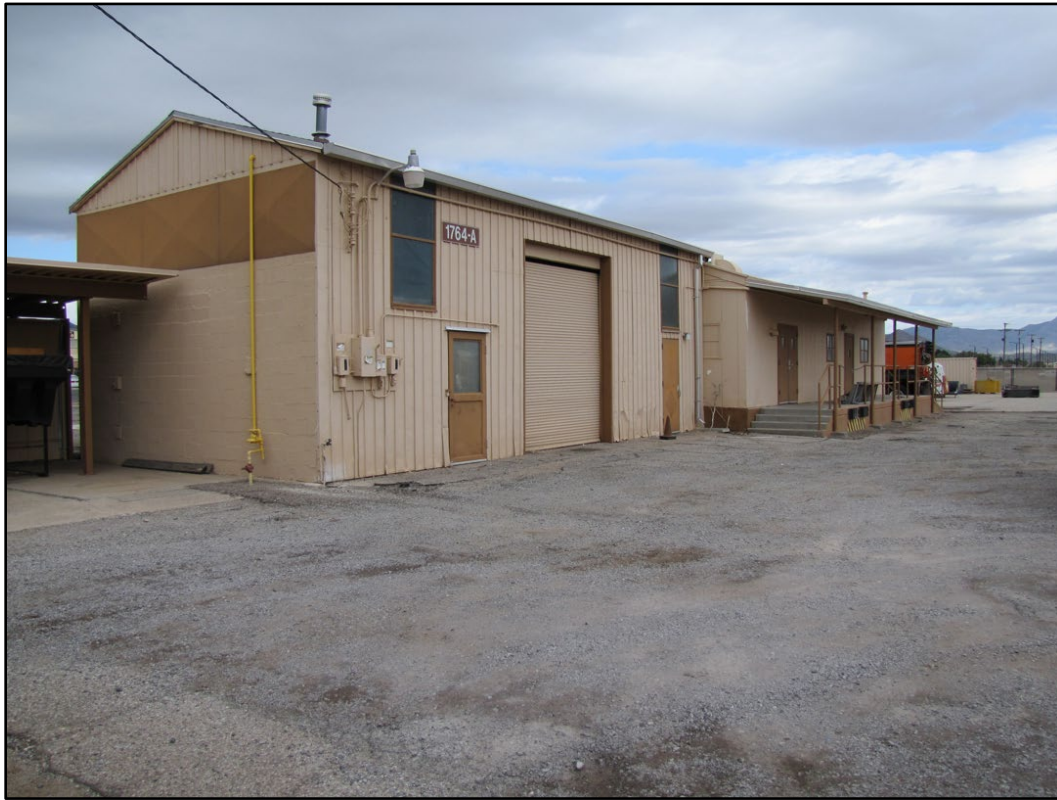
Figure 392. Buildings 1764A and 1764B at WSMR (ERDC-CERL 2016).
