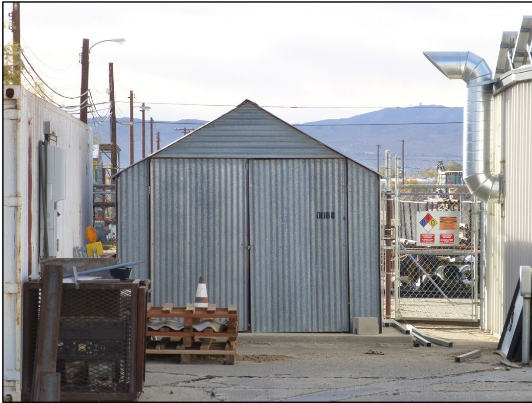
Figure 345. Building 01188 at NAWS China Lake (ERDC-CERL 2016).
