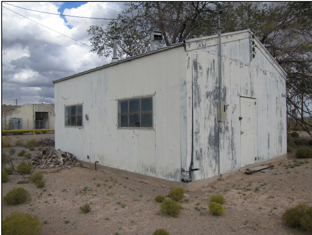
Figure 441. No Number at WSMR (ERDC-CERL 2016).
