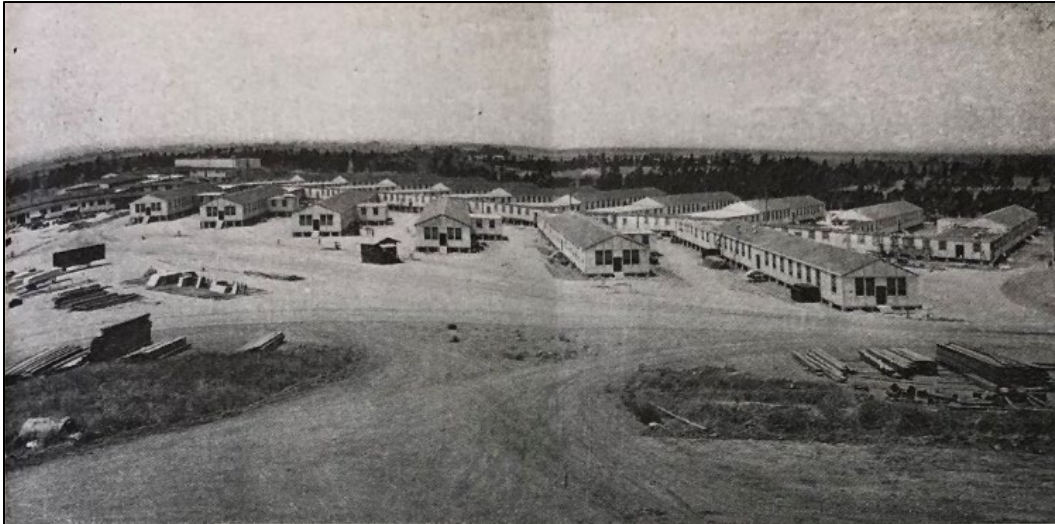
Figure 49. An overview of a naval hospital erected by Modulok in an “unusual herring-bone plan” with one central corridor running in between the two rows of 210’ hospital wards, Southern California (“Prefabricated Naval Hospitals and Housing,” Prefabricated Homes 1-5 (Oct. 1944): 14–15 & 21, 21).
