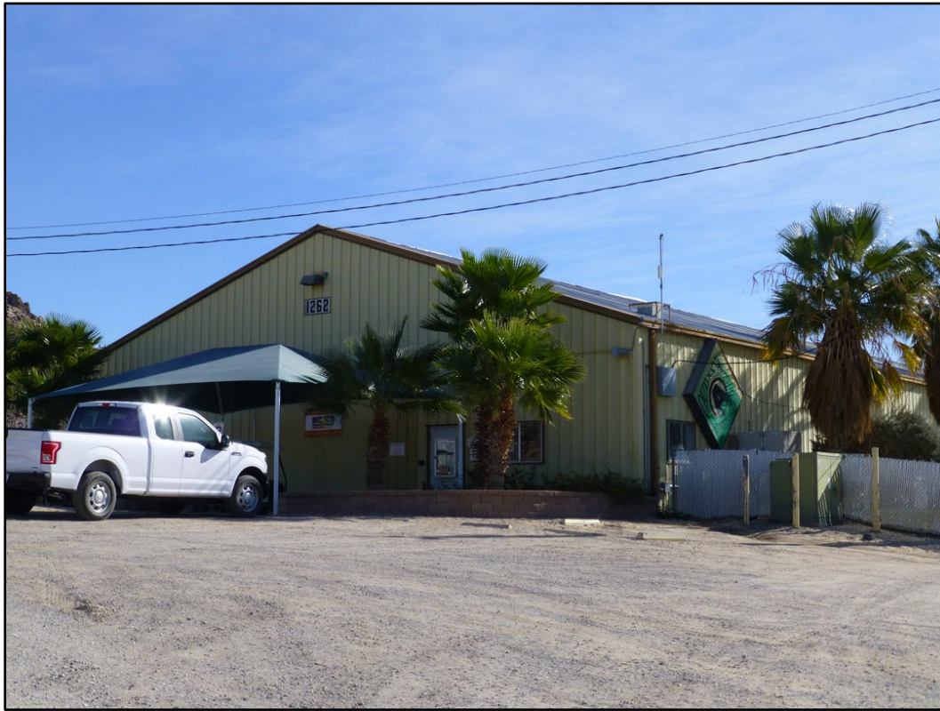
Figure 301. Building 1262 at MCAGCC Twentynine Palms (ERDC-CERL 2016).
