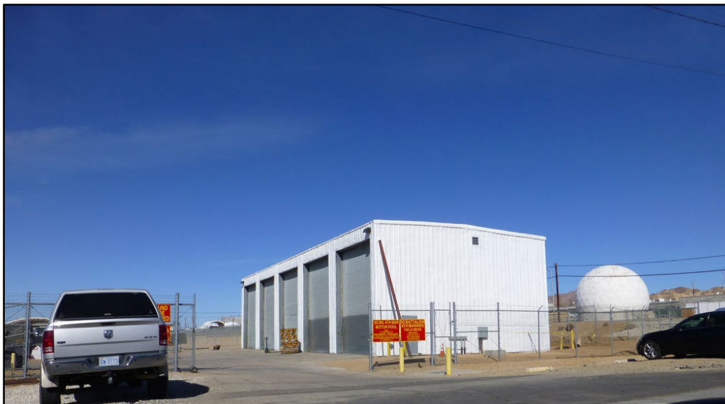
Figure 320. No Number at MCAGCC Twentynine Palms (ERDC-CERL 2016).
