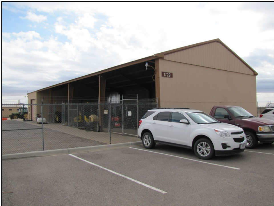
Figure 236. Building 1729 at WSMR (WSMR 2016).
