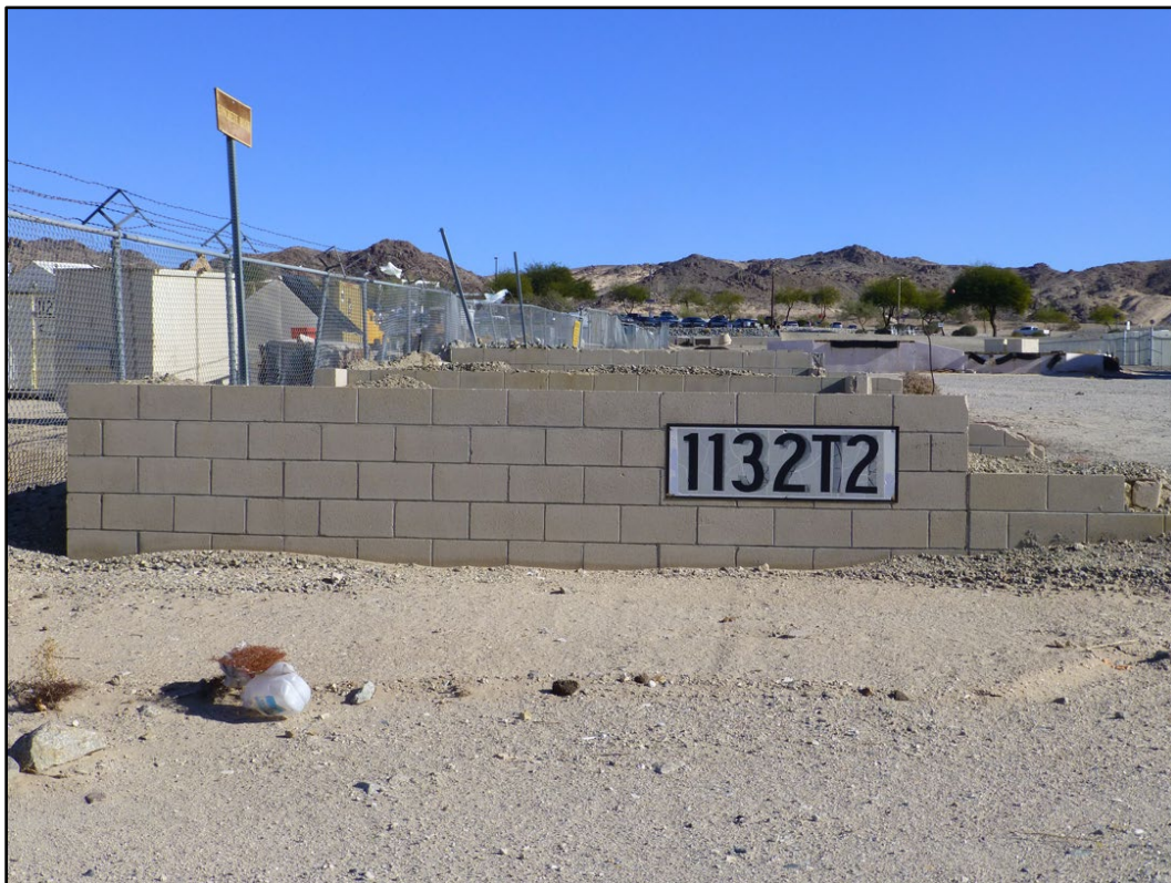
Figure 300. Building 1132T2 at MCAGCC Twentynine Palms (ERDC-CERL 2016).
