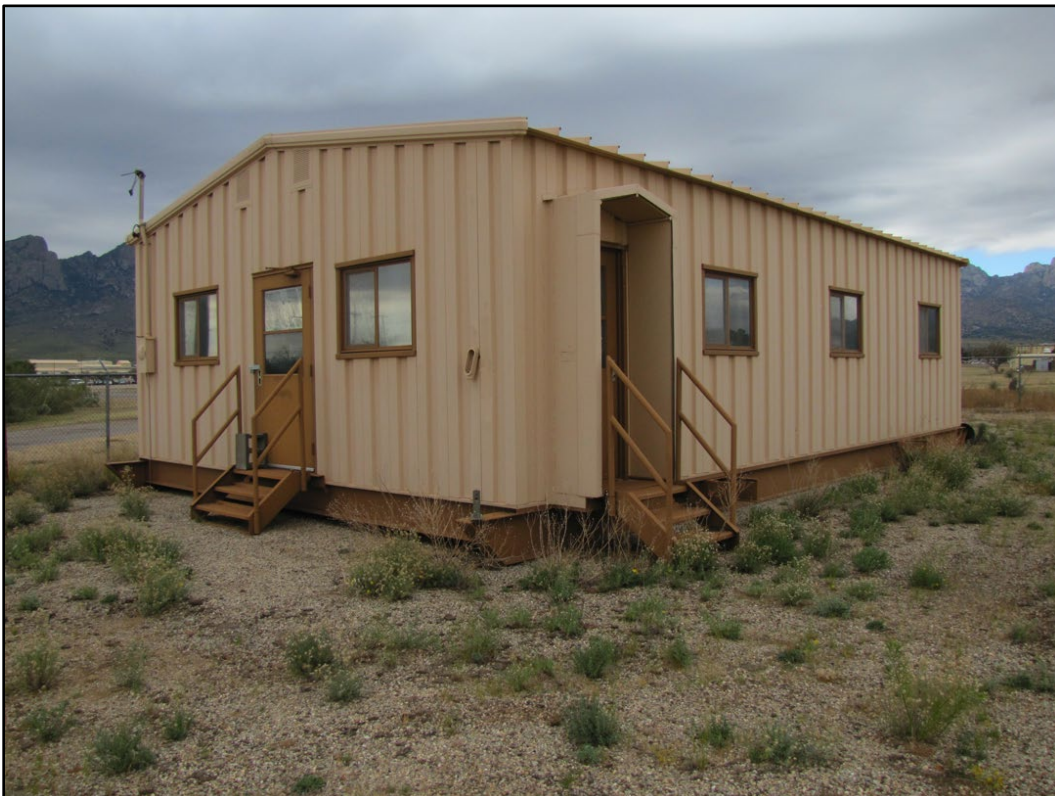
Figure 449. No Number at WSMR (ERDC-CERL 2016).
