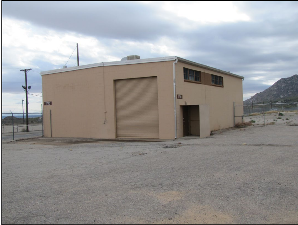
Figure 233. Building 1710 at WSMR (WSMR 2016).
