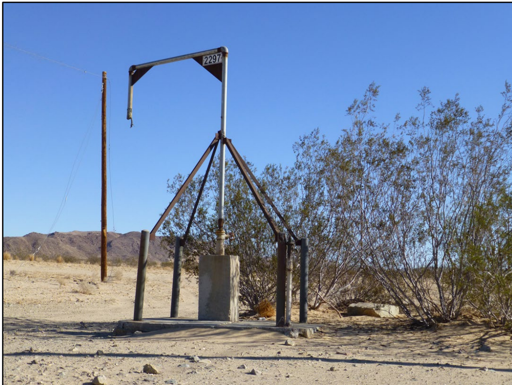
Figure 310. Building 2297 at MCAGCC Twentynine Palms (ERDC-CERL 2016).
