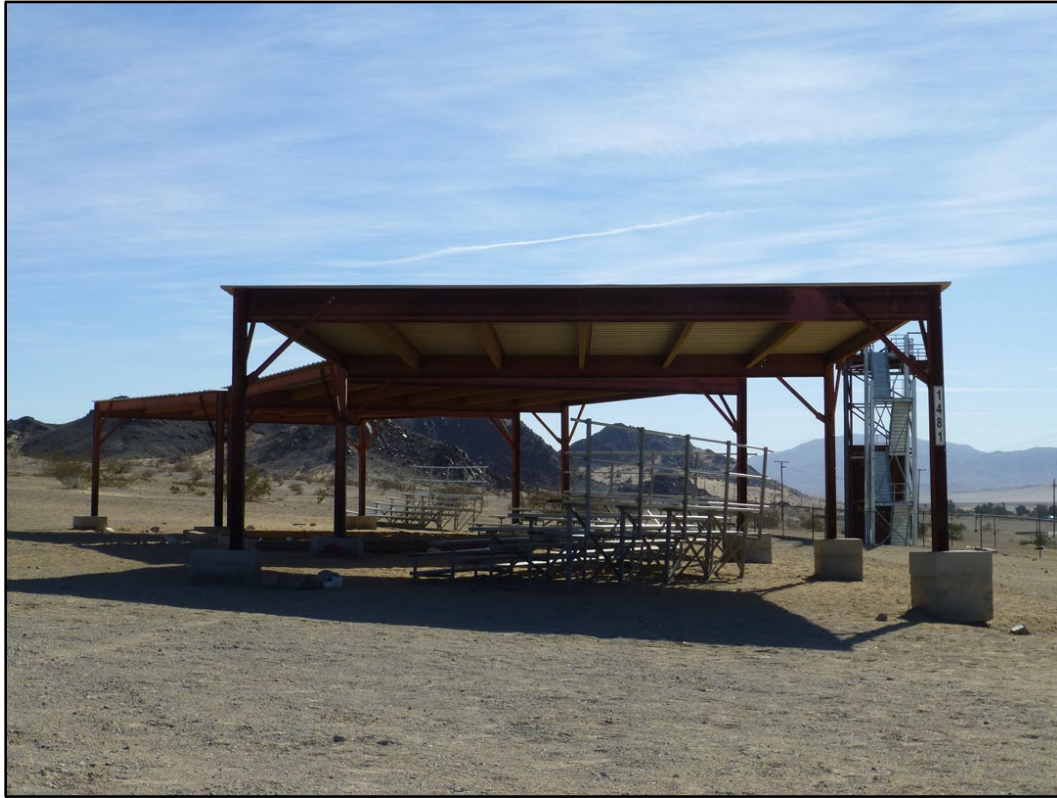
Figure 303. Building 1481 at MCAGCC Twentynine Palms (ERDC-CERL 2016).
