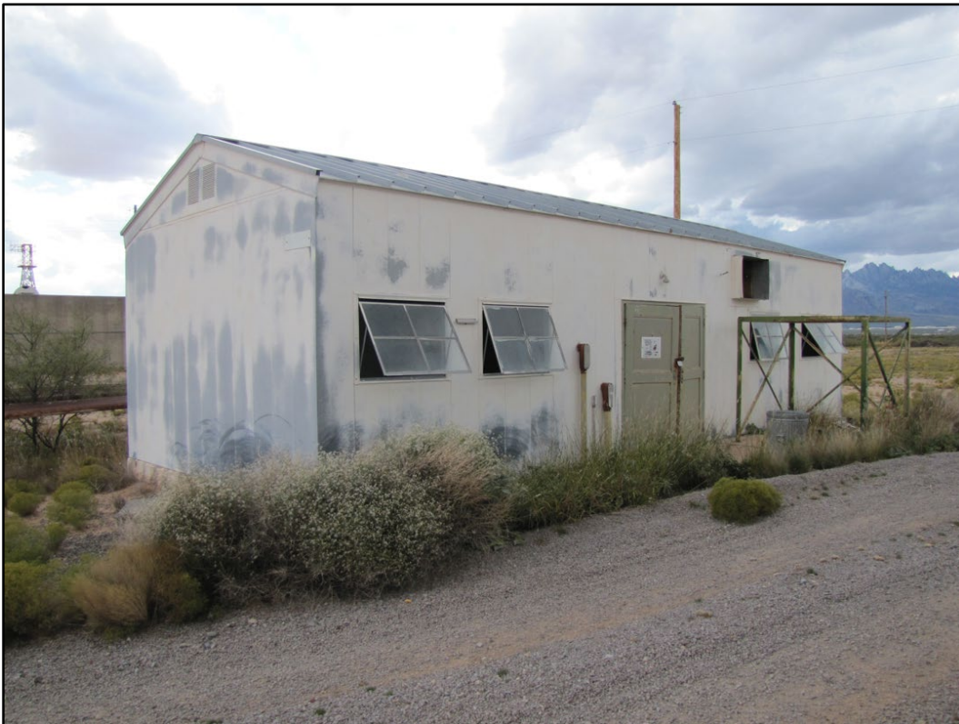
Figure 439. No Number at WSMR (ERDC-CERL 2016).
