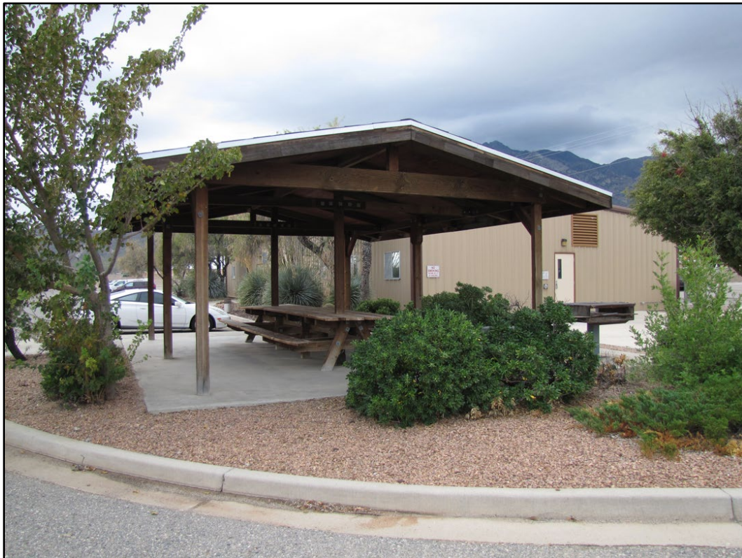
Figure 447. No Number at WSMR (ERDC-CERL 2016).
