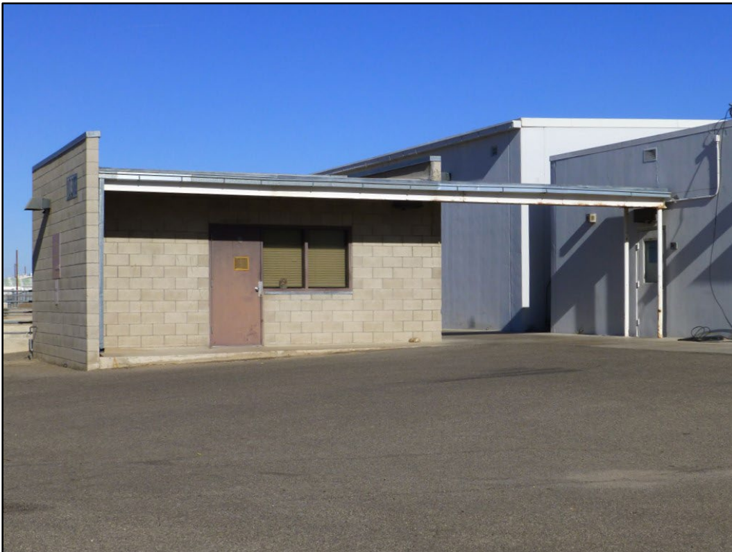
Figure 292. Building 1103T2 at MCAGCC Twentynine Palms (ERDC-CERL 2016).
