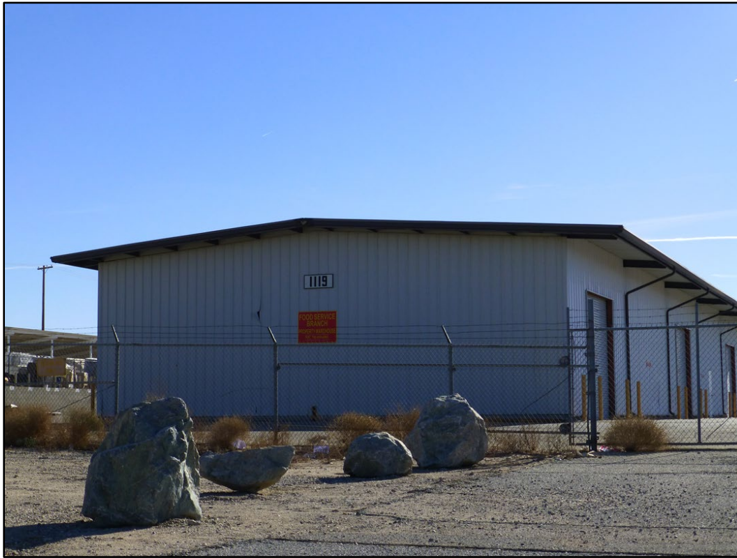
Figure 297. Building 1119 at MCAGCC Twentynine Palms (ERDC-CERL 2016).
