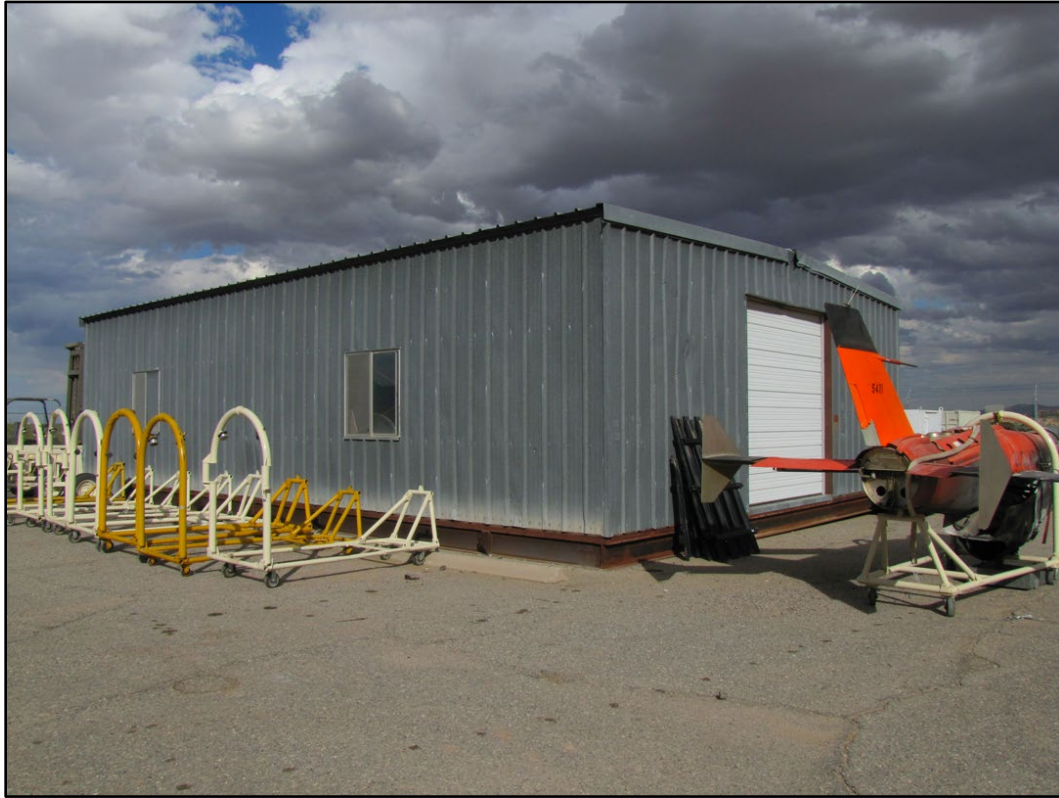
Figure 444. No Number at WSMR (ERDC-CERL 2016).
