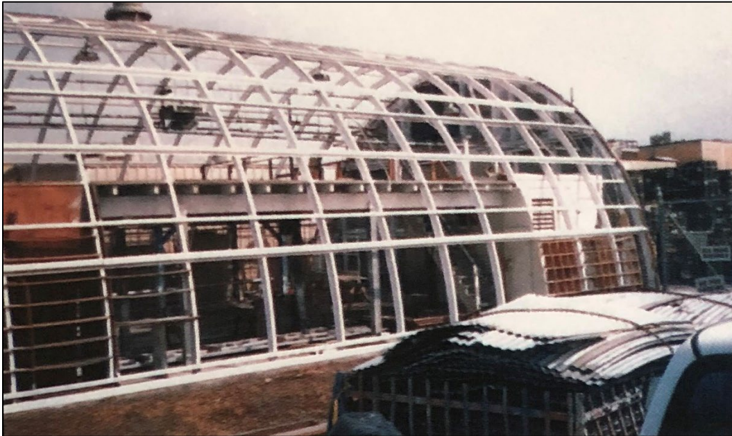
Figure 191. A Quonset hut being rehabilitated by Curveline, Inc., unknown location, 1996 (Curveline, Inc., “New Products & Services: Curved Panels,” Military Engineer 88, no. 581 (Dec. 1996): 68).
