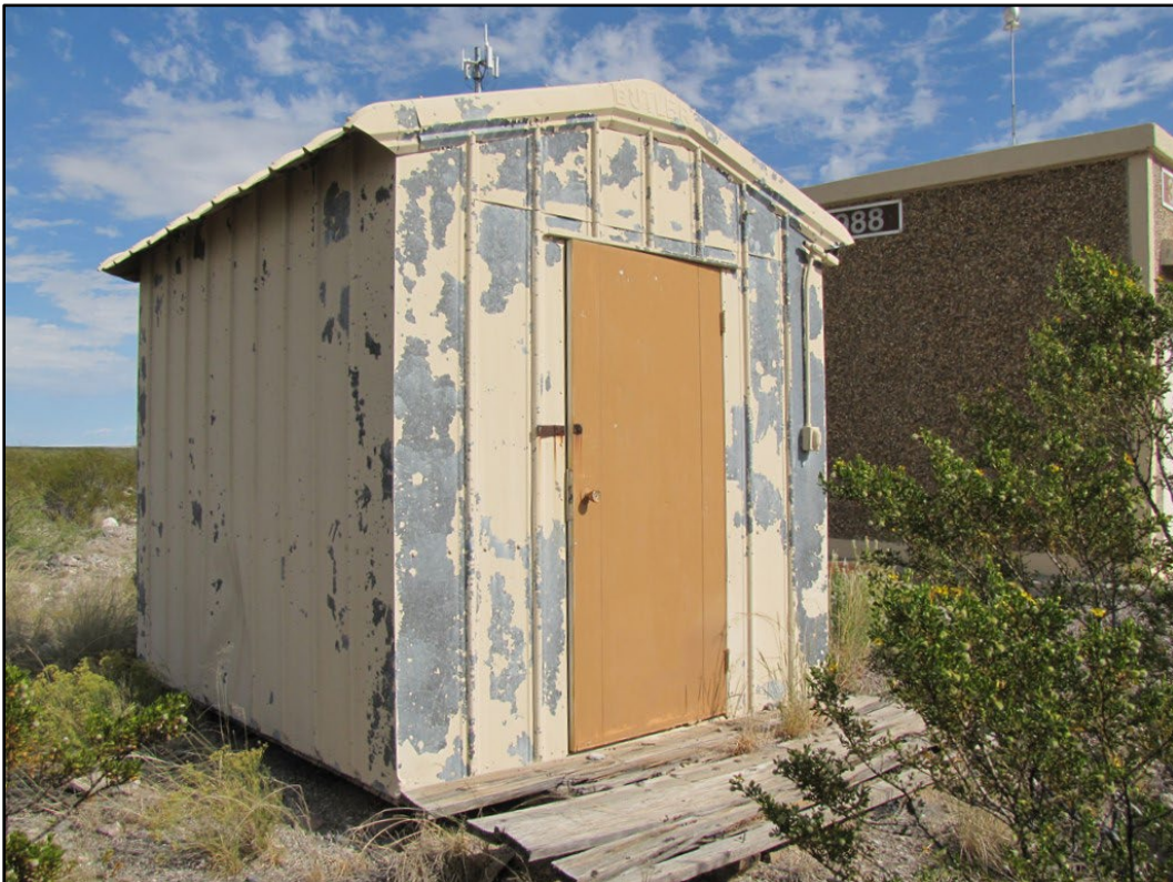
Figure 433. No Number at WSMR (ERDC-CERL 2016).
