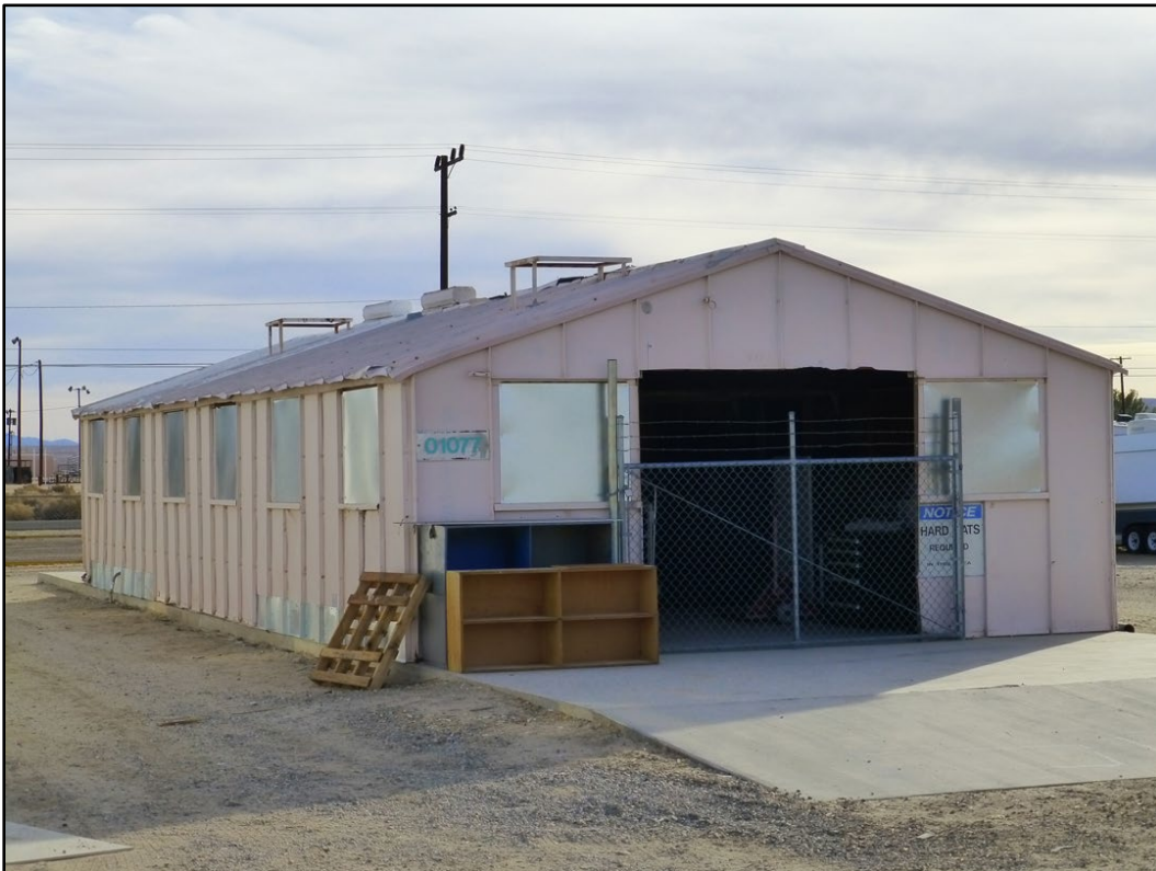
Figure 342. Building 01077 at NAWS China Lake (ERDC-CERL 2016).
