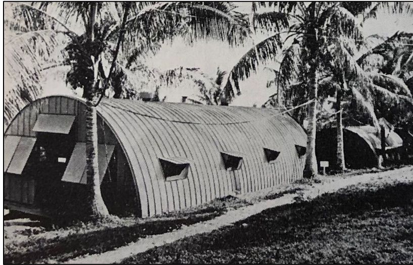
Figure 20. Oblique of a Butler hut deployed in a tropical environment, 1944 ("Prefabricated Emergency Housing and Structures for the Armed Forces," Prefabricated Homes 1-5 (1944): 16-17 ).
