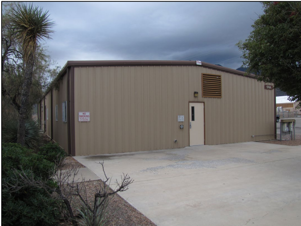
Figure 385. Building 174A at WSMR (ERDC-CERL 2016).
