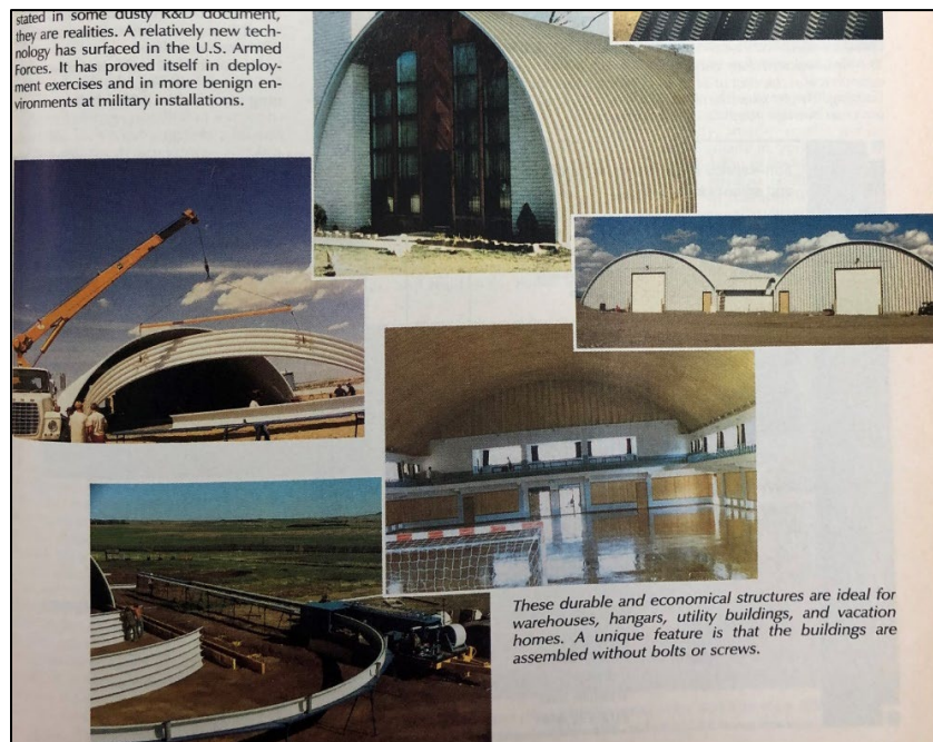
Figure 195. Images of ABM System structures showing both the construction method for and versatility of this building system, 1990 (Forrest T. Gay, “Steel Buildings – On the Double,” The Military Engineer 82, no. 535 (May–June 1990): 53–54).
