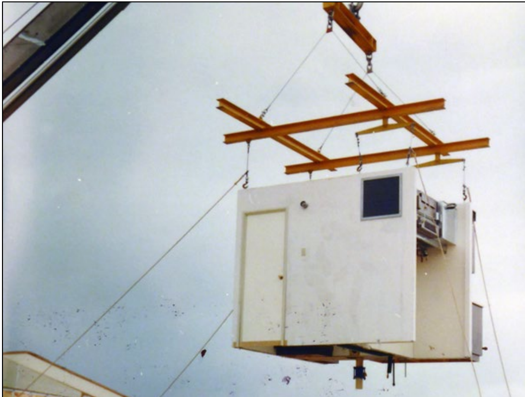
Figure 162. A completed utility core being lifted into place by a crane, George AFB, California 1971 (NARA College Park, RG342-B).
