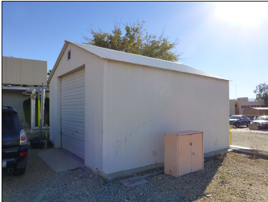
Figure 322. No Number at MCAGCC Twentynine Palms (ERDC-CERL 2016).
