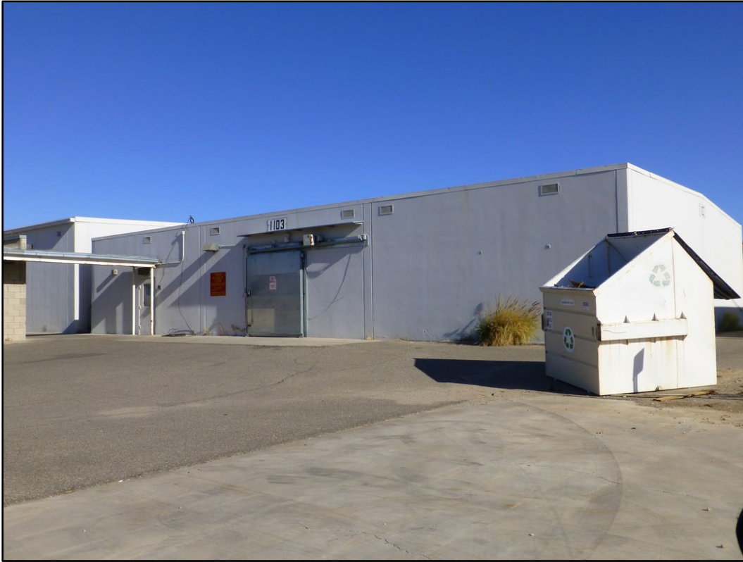
Figure 291. Building 1103 at MCAGCC Twentynine Palms (ERDC-CERL 2016).
