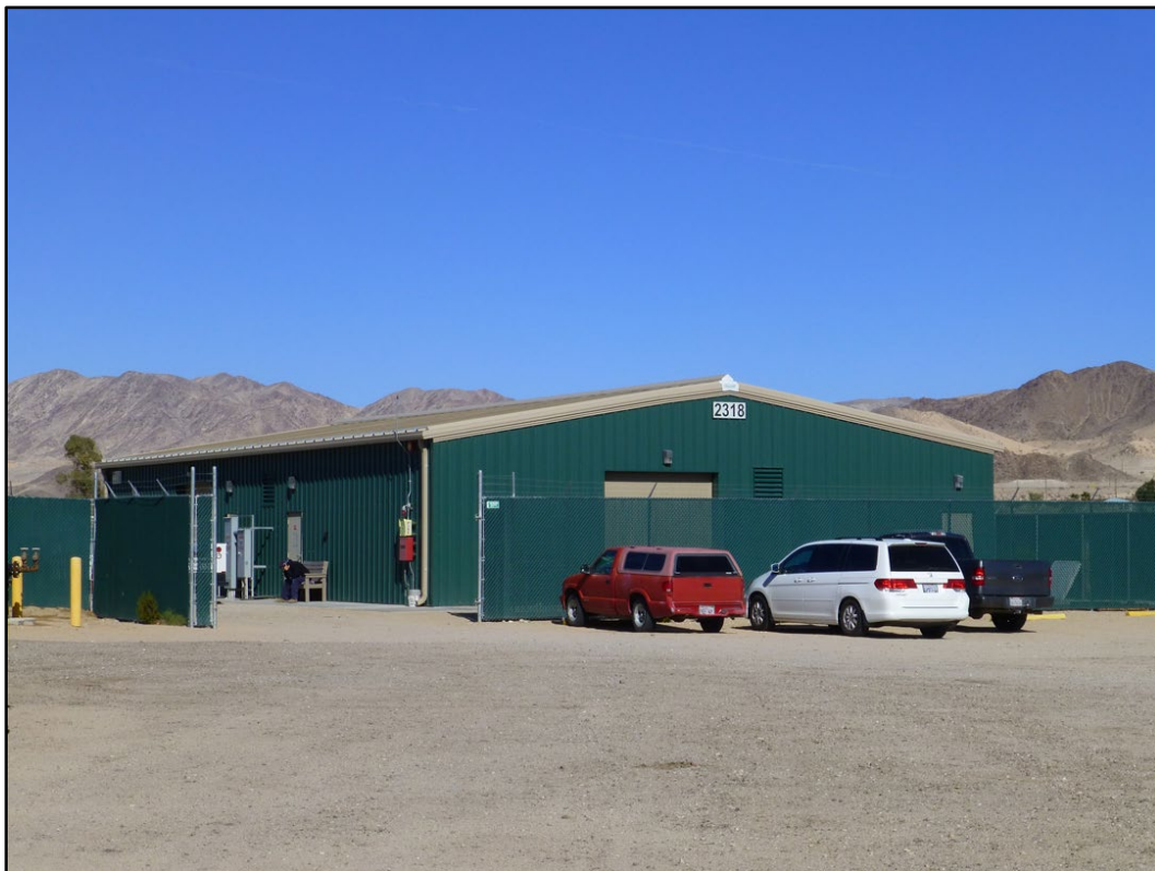
Figure 312. Building 2318 at MCAGCC Twentynine Palms (ERDC-CERL 2016).
