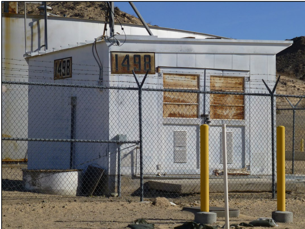
Figure 304. Building 1498 at MCAGCC Twentynine Palms (ERDC-CERL 2016).
