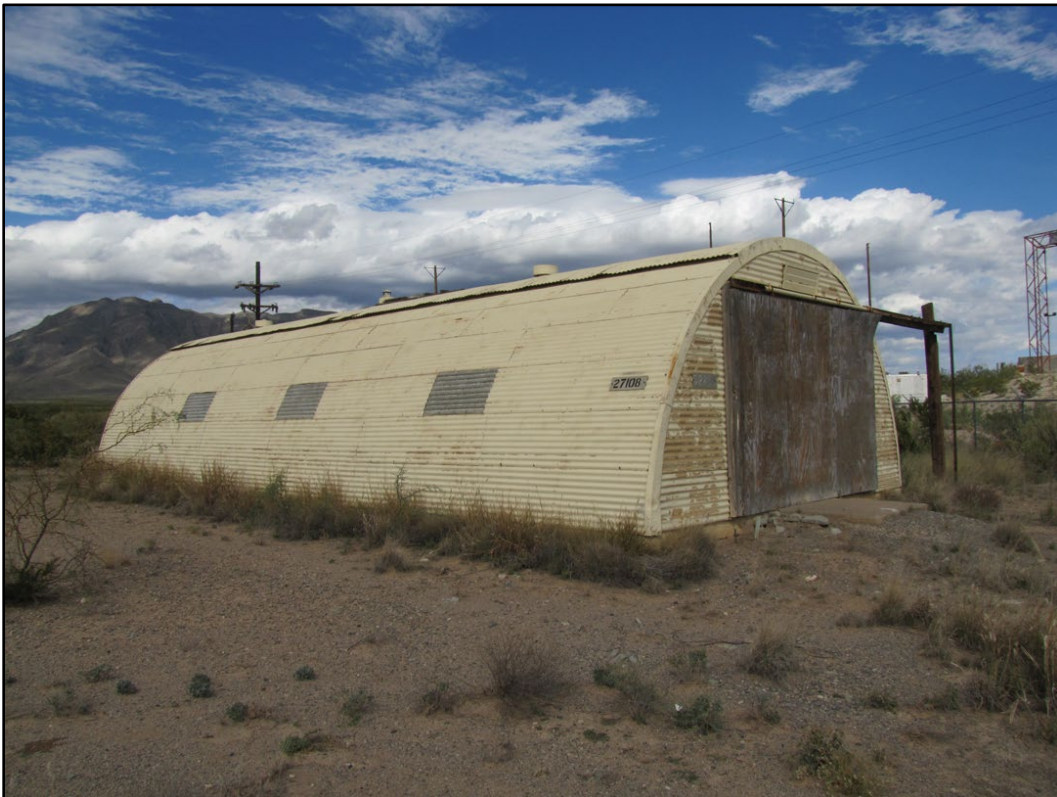
Figure 419. Building 27108 at WSMR (ERDC-CERL 2016).
