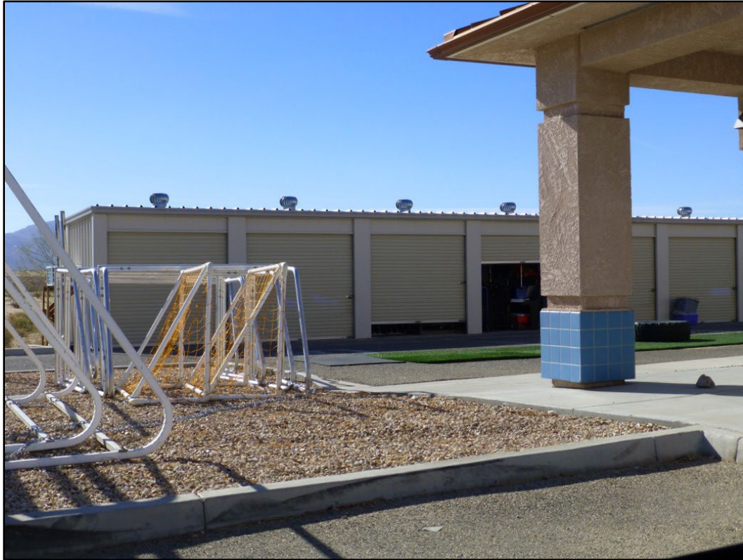
Figure 317. No Number at MCAGCC Twentynine Palms (ERDC-CERL 2016).
