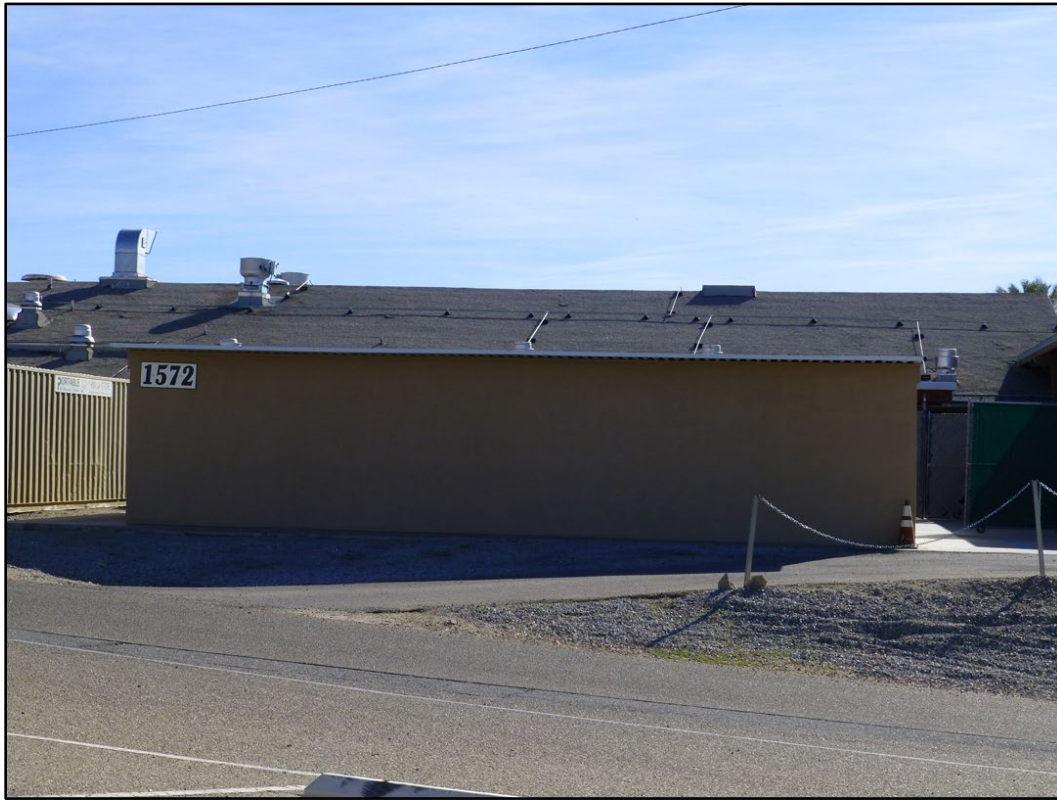
Figure 305. Building 1572 at MCAGCC Twentynine Palms (ERDC-CERL 2016).
