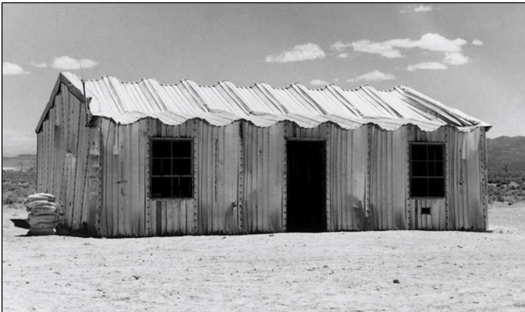
Figure 100. A Behlen frameless stressed skin building after surviving an atomic blast at Yucca Flats, Nevada, 1955 (Behlen Manufacturing Company, "Bomb Shelters," History, accessed December 18, 2018, https://www.behlenmfg.com/history ).
