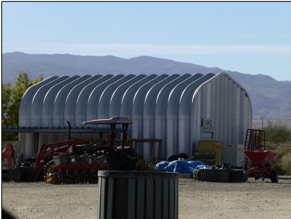
Figure 219. Building 1092 at MCAGCC Twentynine Palms (ERDC-CERL 2016).
