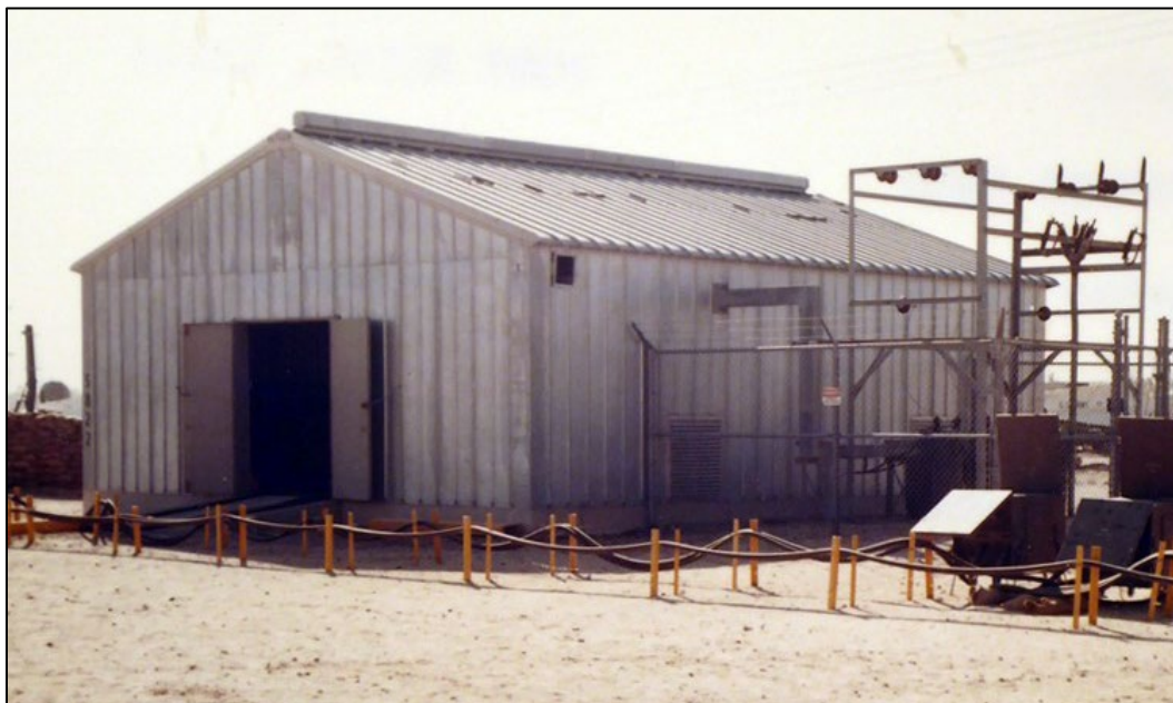
Figure 150. A Butler building used as a converter shed, a typical US military utilization of small metal prefabricated building where a wooden structure would provide a fire hazard, Fort Bliss, Texas, 1966 (NARA 111-CCS).
