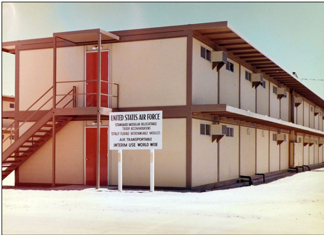
Figure 166. Modular barracks at Nellis AFB, Nevada photographed shortly after completion, 1968 (NARA College Park, RG342-B).
