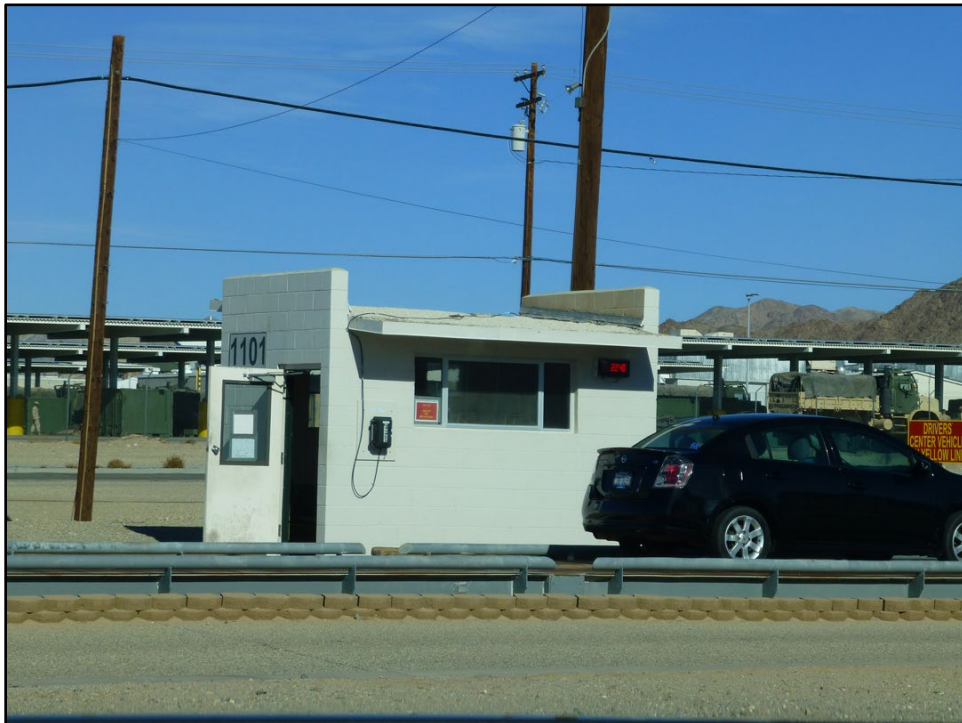
Figure 221. Building 1101 at MCAGCC Twentynine Palms (ERDC-CERL 2016).
