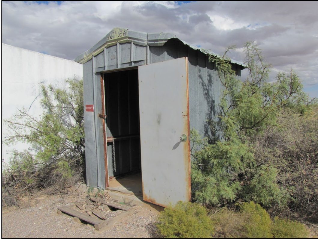
Figure 436. No Number at WSMR (ERDC-CERL 2016).
