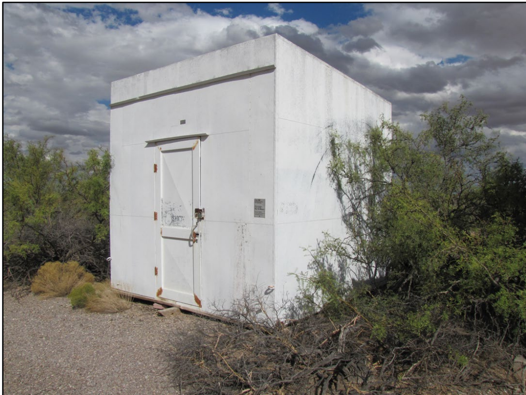
Figure 437. No Number at WSMR (ERDC-CERL 2016).
