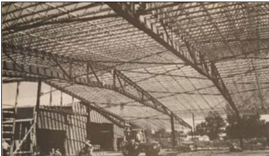
Figure 210. The frame of a building erected by TrusWal Systems Inc. showing the SpaceJoist Webs in the flat chord truss (Jack N. Schmidt, “Schmidt: Truss Business Will Double in Next 10 Years,” Automation in Housing and Building System News (Feb. 1979): 55).
