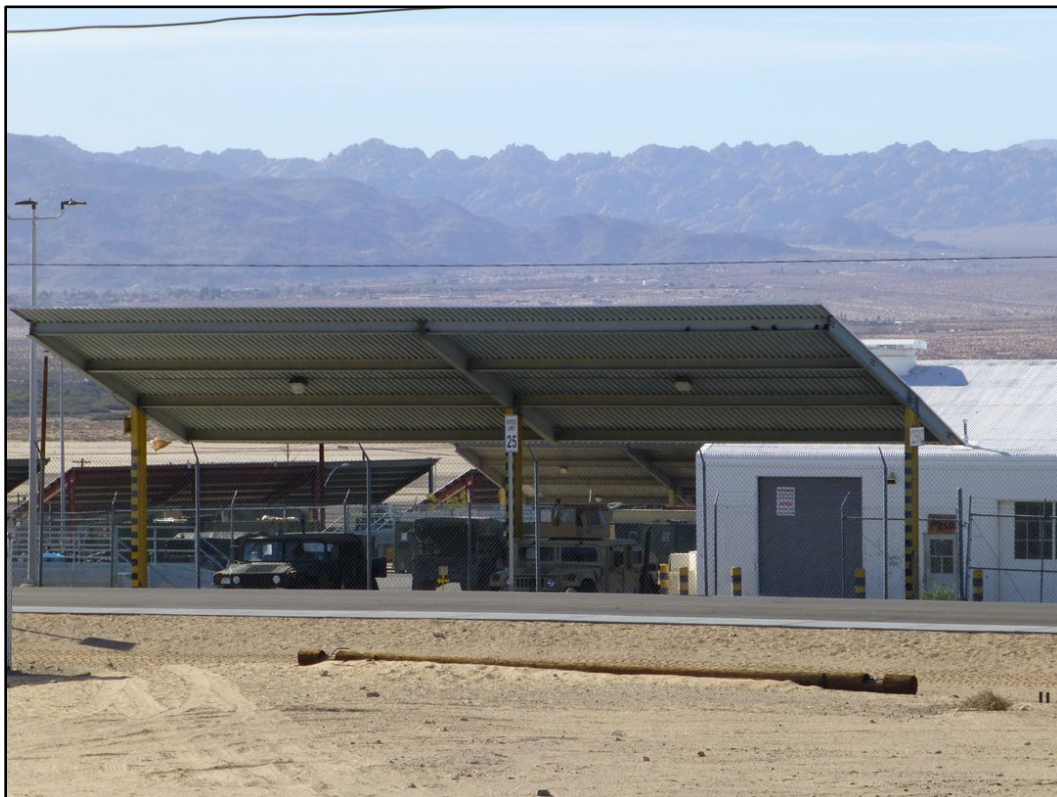
Figure 302. Building 1278Y1 at MCAGCC Twentynine Palms (ERDC-CERL 2016).
