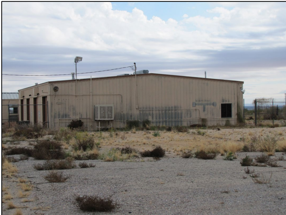
Figure 234. Building 1713 at WSMR (WSMR 2016).
