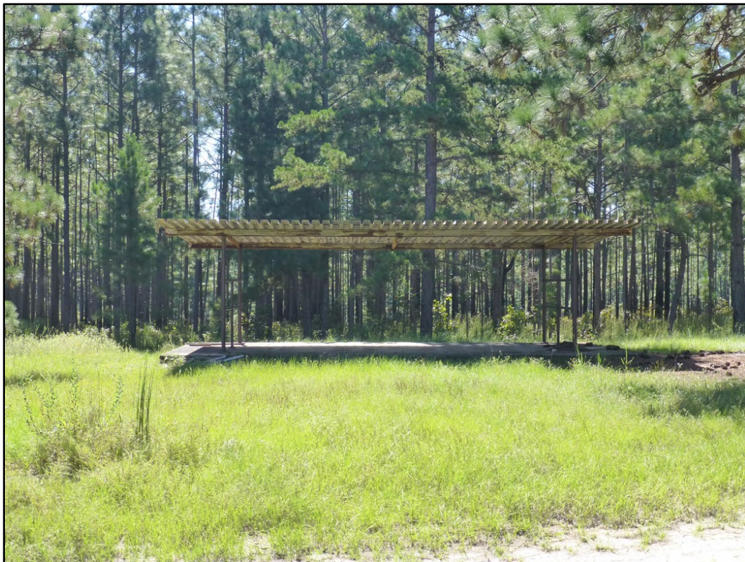
Figure 289. No Number at Fort Polk (ERDC-CERL 2016).
