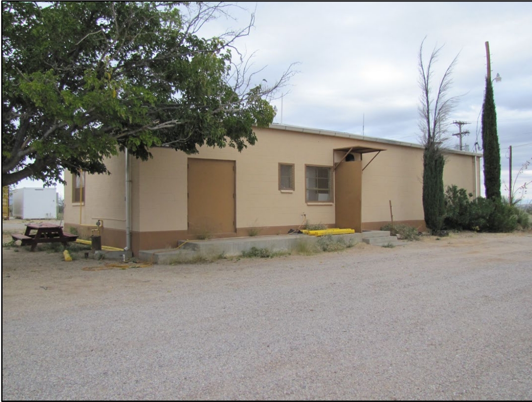
Figure 388. Building 312 at WSMR (ERDC-CERL 2016).
