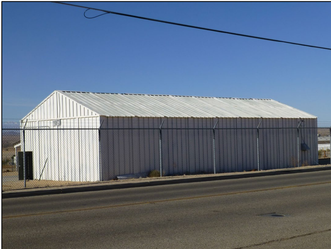
Figure 294. Building 1108T2 at MCAGCC Twentynine Palms (ERDC-CERL 2016).
