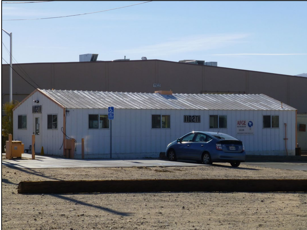
Figure 290. Building 1102T1 at MCAGCC Twentynine Palms (ERDC-CERL 2016).
