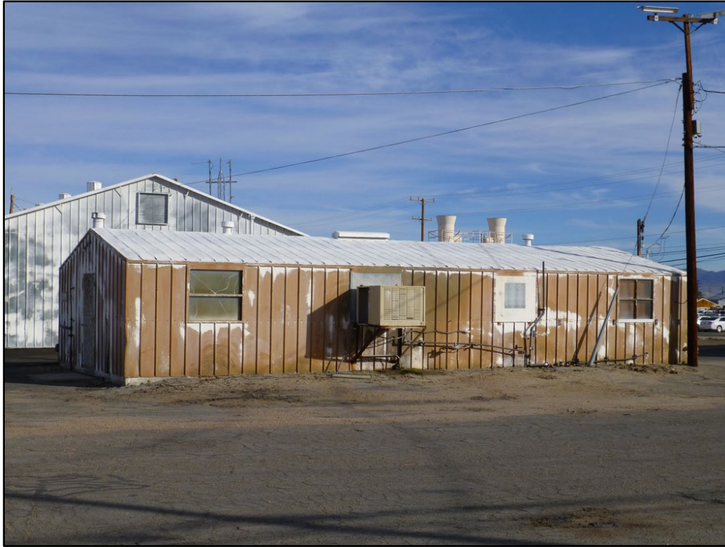
Figure 343. Building 01096 at NAWS China Lake (ERDC-CERL 2016).
