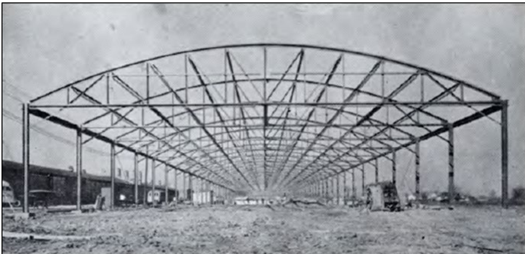
Figure 80. The steel frame of a Mesker prefabricated building with bowstring truss roof supports, 1948 (Geo. L. Mesker Steel Corporation, "Catalog E," Evansville, IN: Geo. L. Mesker Steel Corporation, 1948).
