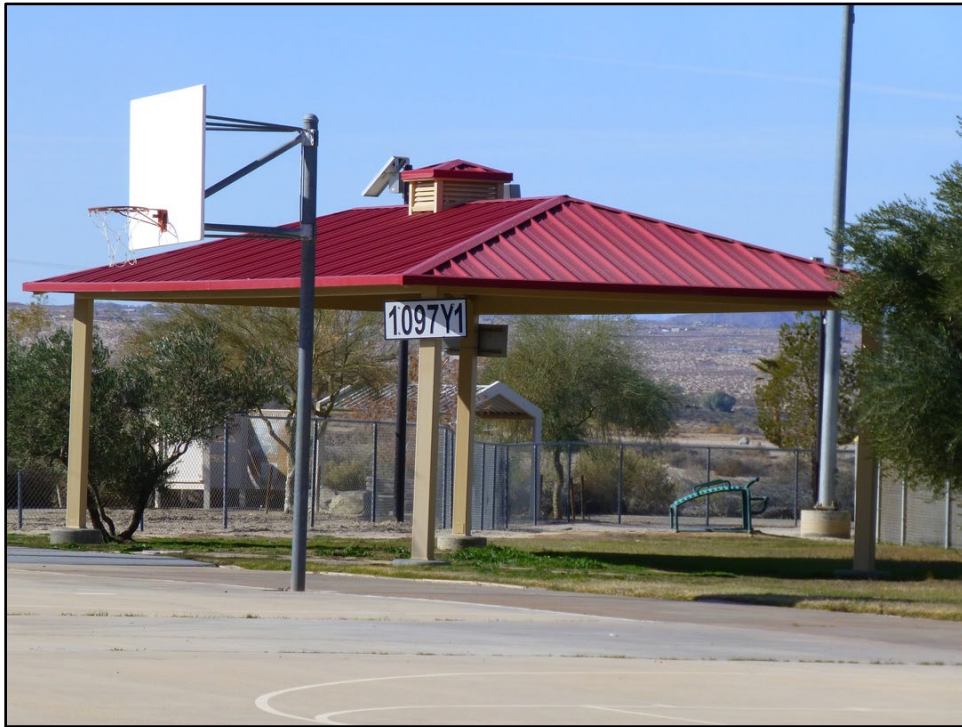
Figure 220. Building 1097Y1 at MCAGCC Twentynine Palms (ERDC-CERL 2016).
