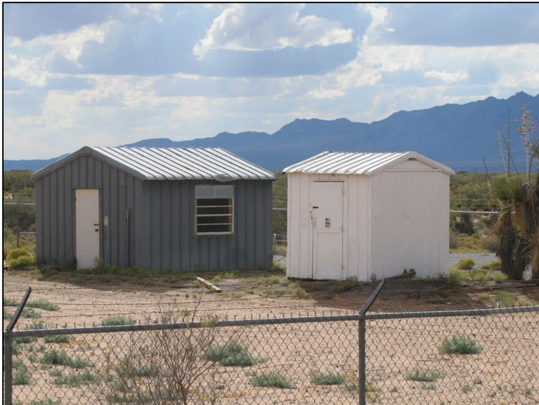
Figure 435. No Numbers at WSMR (ERDC-CERL 2016).
