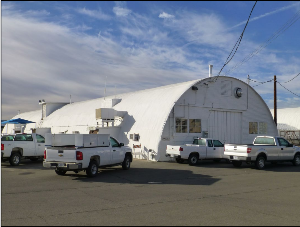
Figure 341. Building 00992 at NAWS China Lake (ERDC-CERL 2016).
