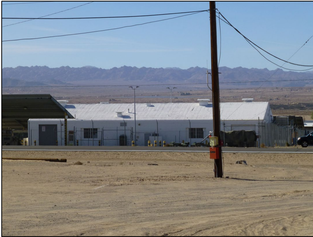
Figure 319. No Number at MCAGCC Twentynine Palms (ERDC-CERL 2016).
