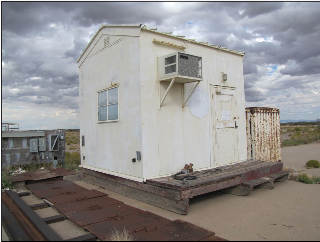
Figure 440. No Number at WSMR (ERDC-CERL 2016).
