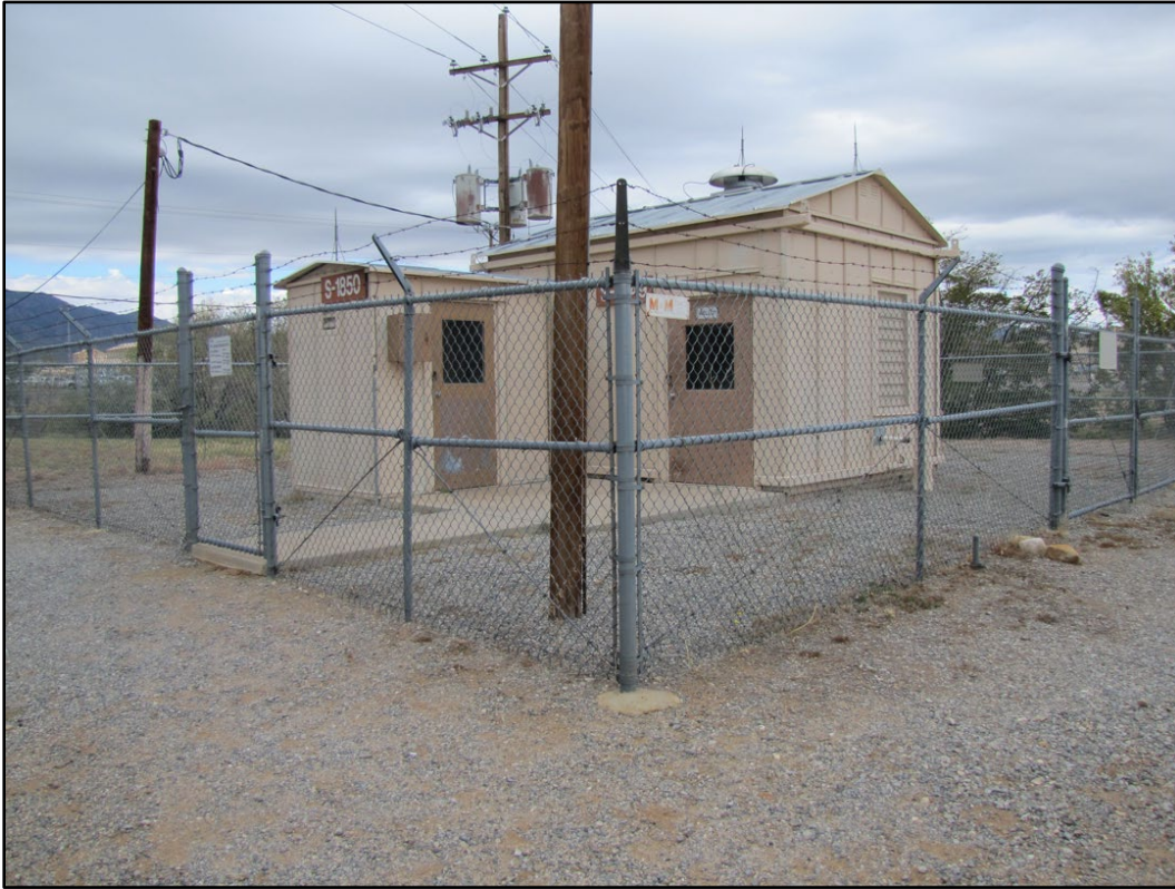
Figure 396. Buildings 1849 and 1850 at WSMR (ERDC-CERL 2016).
