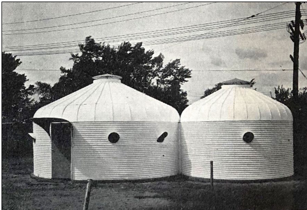
Figure 26. An exterior view of two Dymaxion Deployable Units connected to make a housing unit, 1944 ("Prefabricated Emergency Housing and Structures for the Armed Forces," Prefabricated Homes 1-5 (1944): 16-17).
