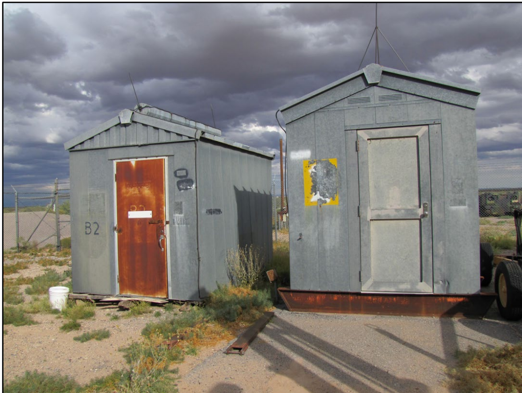
Figure 443. No Numbers at WSMR (ERDC-CERL 2016).
