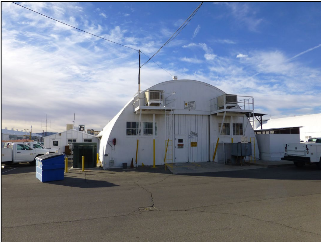
Figure 376. Building 1198 at NAWS China Lake (ERDC-CERL 2016).
