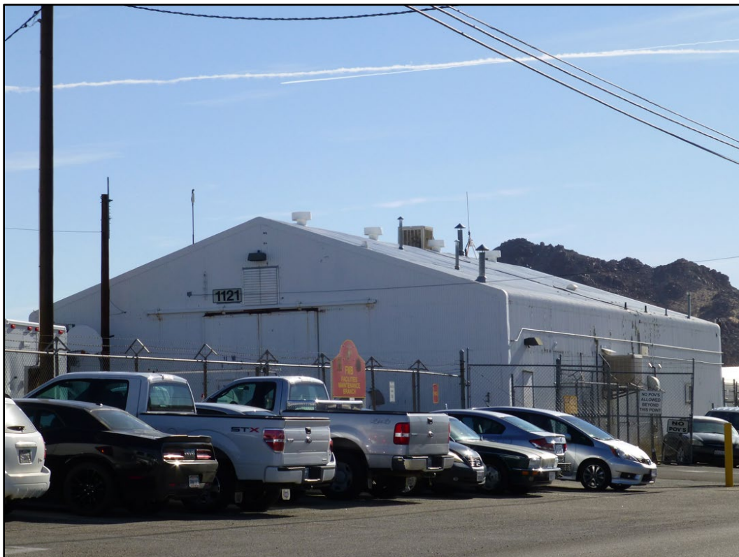
Figure 298. Building 1121 at MCAGCC Twentynine Palms (ERDC-CERL 2016).
