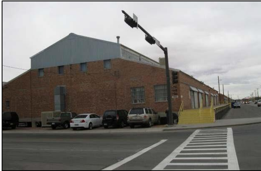
Figure 69. Bldg. 1103, general purpose warehouse.
