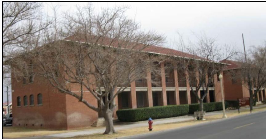
Figure 68. Bldg. 115, Fort Bliss.
