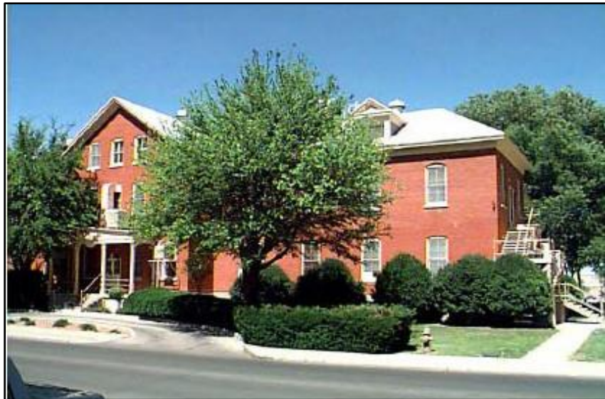
Figure 67. Bldg. 1, Fort Bliss.
