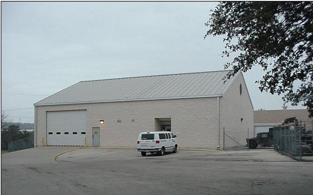
Figure 17. Existing Building 12 (built c. 1942) with CMU walls and metal roof located near APE, 2017 (Texas Military Department).
