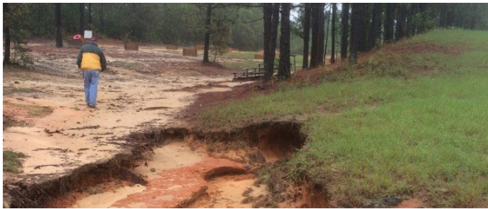
Flooding in the training area at Fort Jackson, SC. Source: US Army Photo
