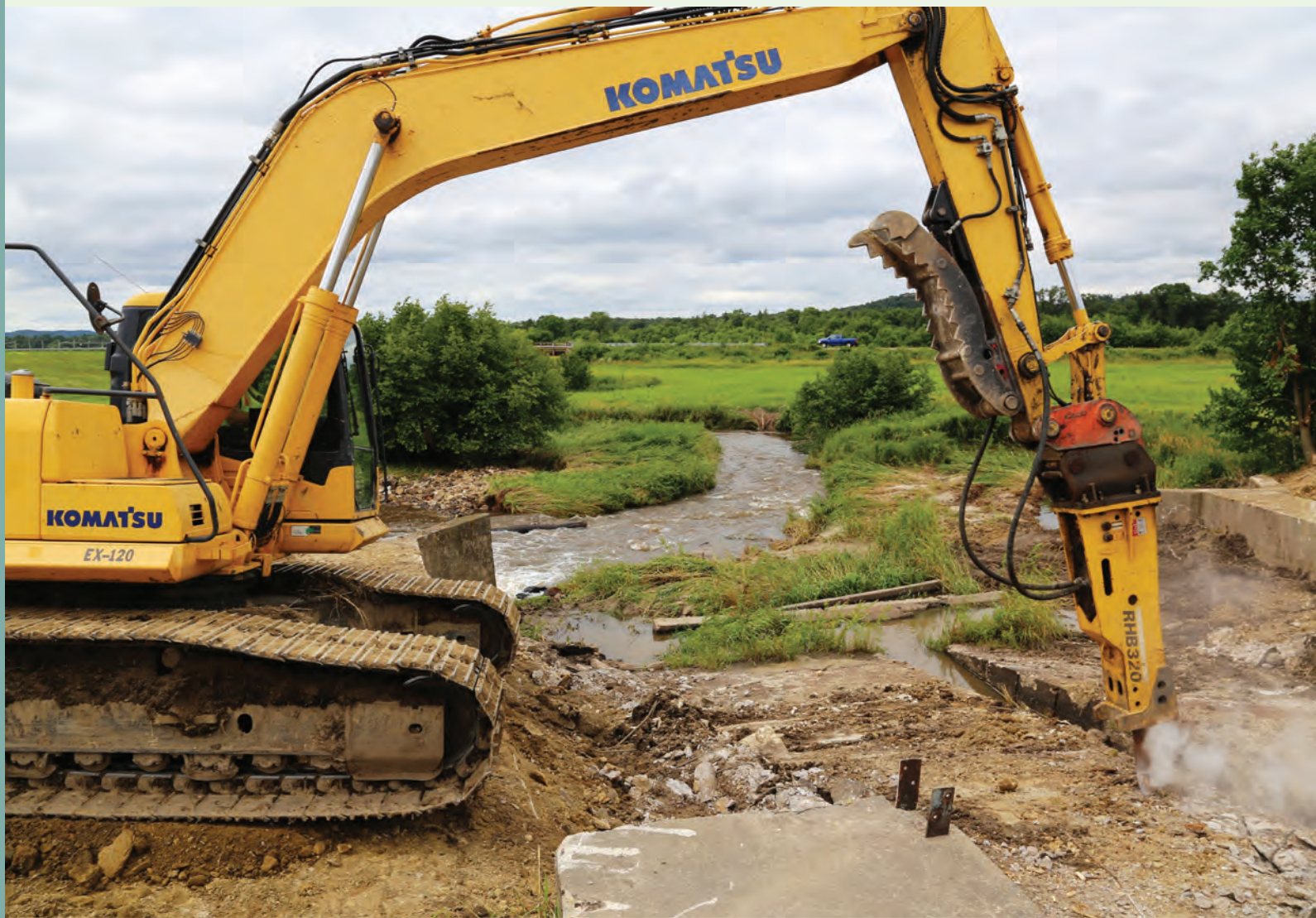
Removing an old dam to enhance and reconnect fish habitat was a shared priority of Fort McCoy, Wisconsin Department of Natural Resources, and U.S. Fish and Wildlife Service. Photo: Scott T. Sturkol/Army.
