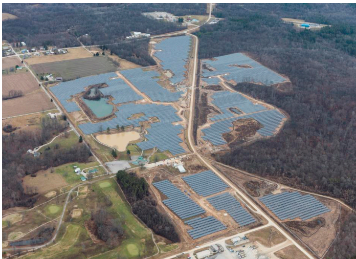
Solar array at Naval Air Station Crane. Source: DoD PIF
