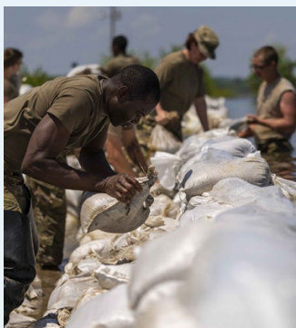
Army National Guardsmen lay sandbags at a flooding site in East Cape Girardeau, IL.
