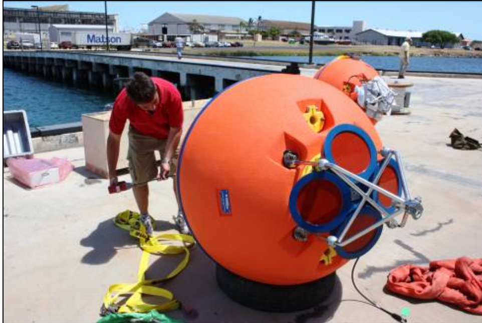
Figure 10. National Data Buoy Center (NDBC) Engineer, Bret Taft, attaching Teledyne 75kHz ADCP and cage to Flotation Technologies 49-in [124-cm] ADCP buoy, July 21, 2009. One of two used at the deepwater mooring.
