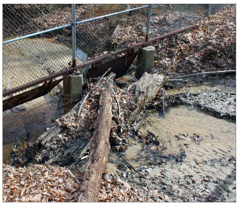
(Photos courtesy of USACE, Baltimore District) USACE, Baltimore District is assisting Joint Base Andrews in addressing potential security issues when drift and debris from local streams lodge swing gates open, providing access for people and pollution.
