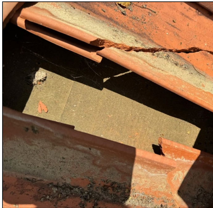
Asphalt Shingle beneath damaged Terra Cotta Clay Tile Roof, Pope Army Airfield, Fort Bragg (Corvias)
