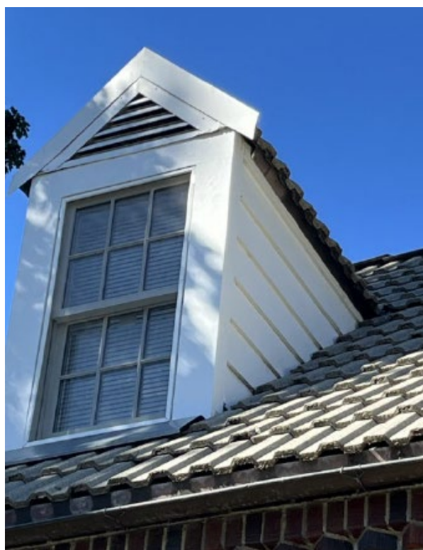
Dormer at Joint Base Lewis McChord with dry rot replaced (JBLM 2024)
