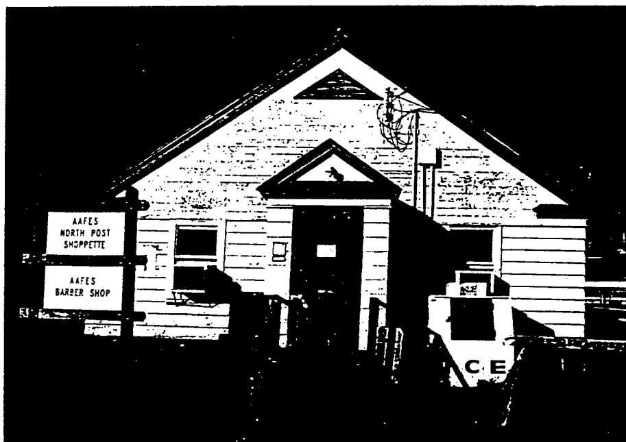
Figure 2. Arctic entry added to Nurses Quarters at Ladd Field (now Fort Wainwright) near Fairbanks, Alaska.
