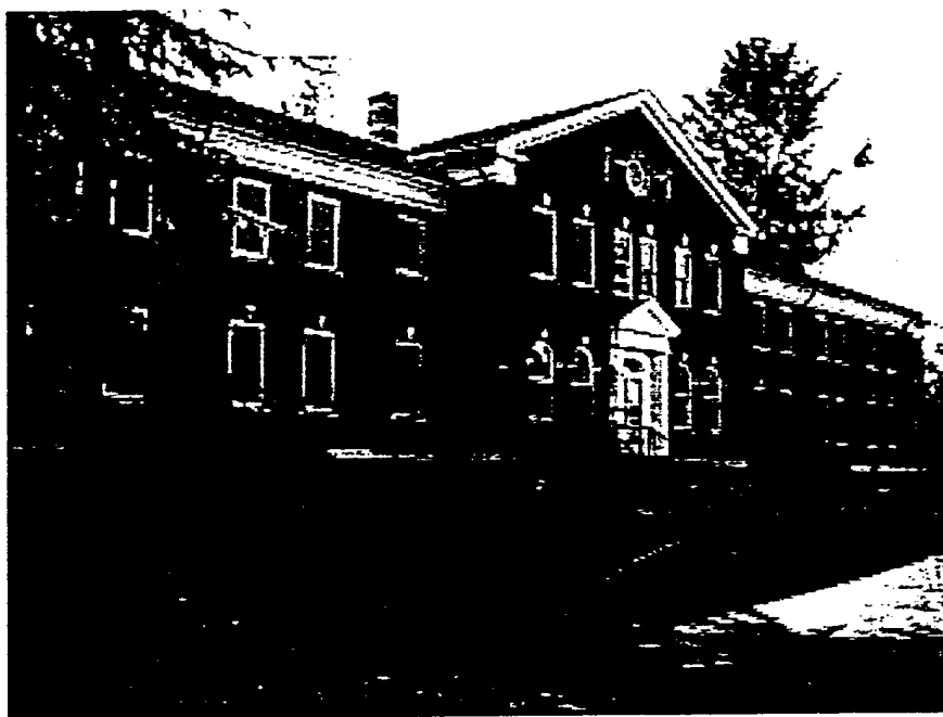
1934 Bachelor Officers Quarters at Fort Lewis, WA
