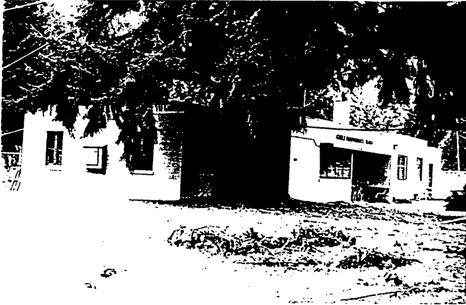
Radio Transmitter Building (Building 830, McChord Air Field, Washington) Constructed in 1939
