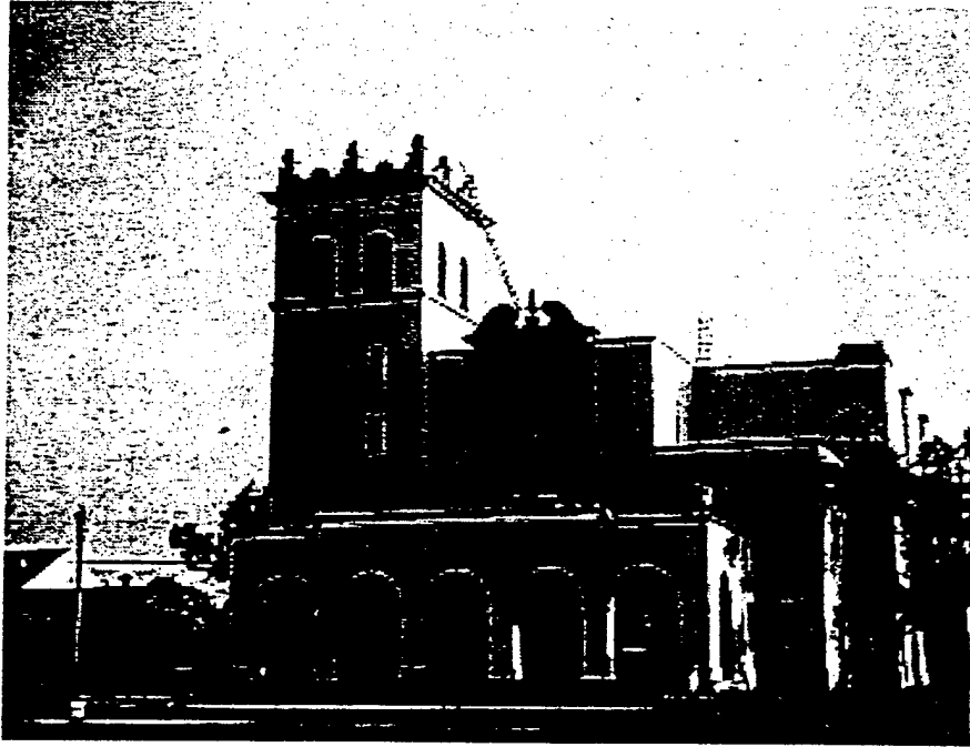
1930 s Main Theater at Fort Sam Houston, TX
