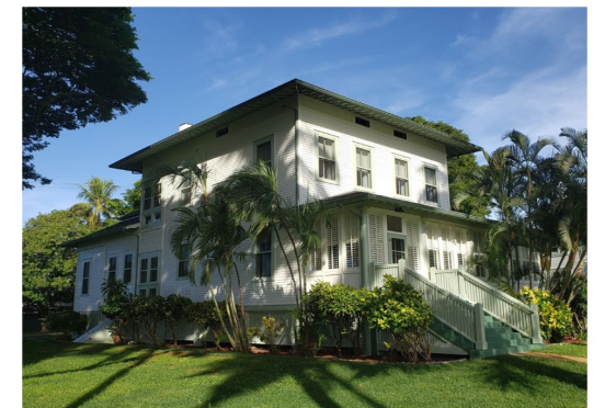
Fort Shafter, HI
