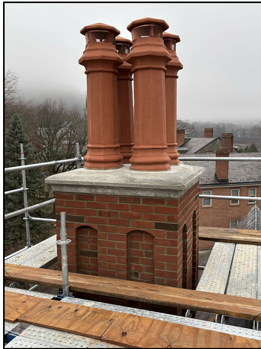
Replacement imitative substitute chimney pots on Quarters 102 (West Point 2024)
