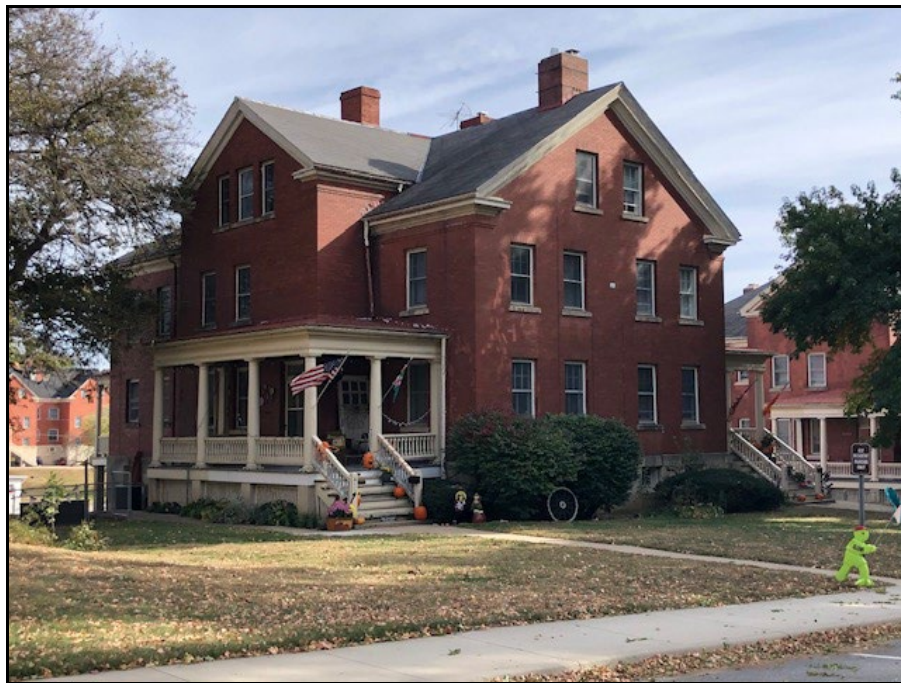
Pre-1919 Residence at Fort Leavenworth (Goodwin 2024)
