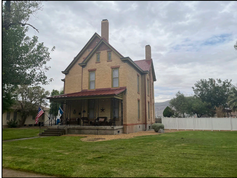
Pre-1919 Era Residence at Fort Bliss (Goodwin 2024)
