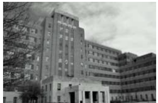
Main Hospital, Building 500
