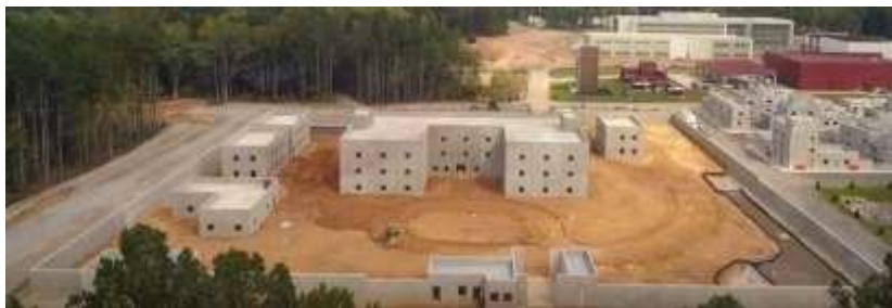
The Mock Embassy Training facility at the State Department's Foreign Area Security Training Center while under construction in 2020 on excessed Army property at Fort Pickett.
