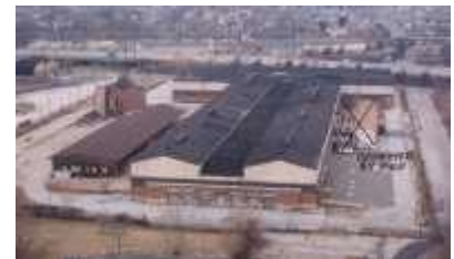
Tacony Warehouse Complex
