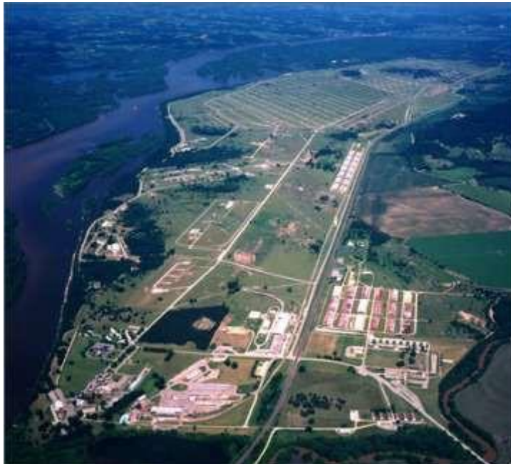
Aerial view of SVADA looking north
