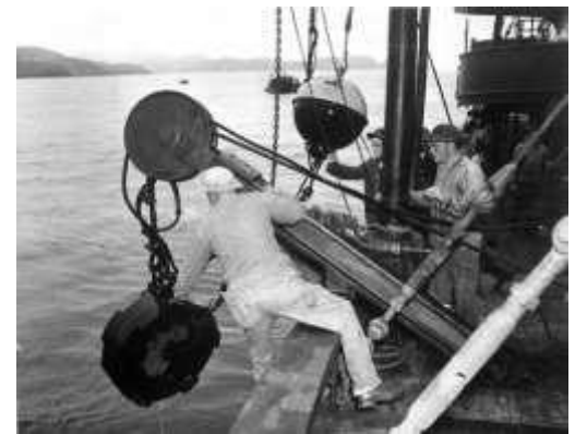
EFB soldiers laying mines in 1942
