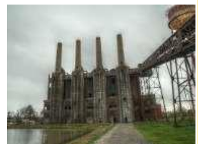
Original ALAAP Power Plant
