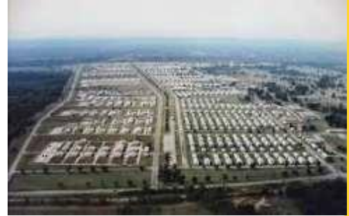
FT Chaffee cantonment area prior to closure
