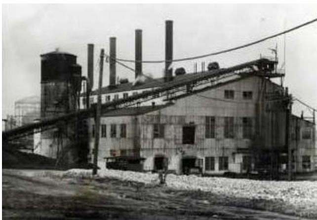
Original VOAAP Power Plant
