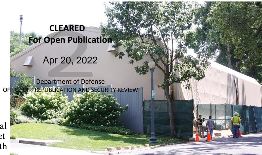
*During the height of remedial efforts, a tent covered the Glenbrook Road Remedial Action site. The tent allowed the team to work safely and efficiently while they excavated and removed hazardous materials and contaminated soil.*
