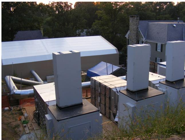
*Three large chemical agent filters are connected to the containment tent by ductwork. These filters were adapted for use at this site with sound suppression structures so that their large electric motors would not disturb the neighborhood after hours.*
