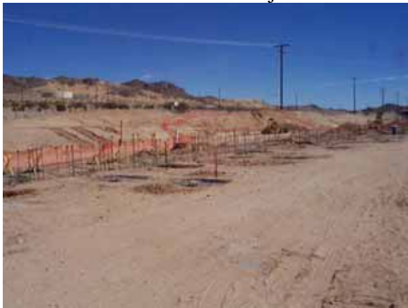
Construction Site Monitoring
