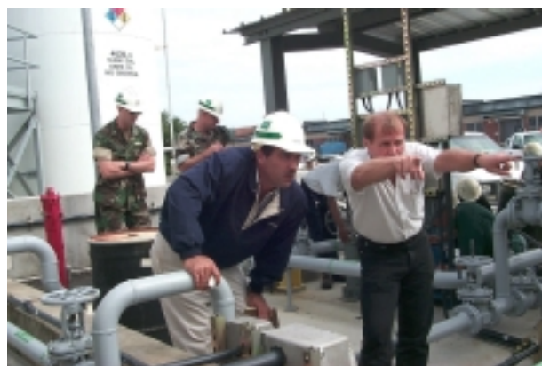
Final inspection of Blending Facility
