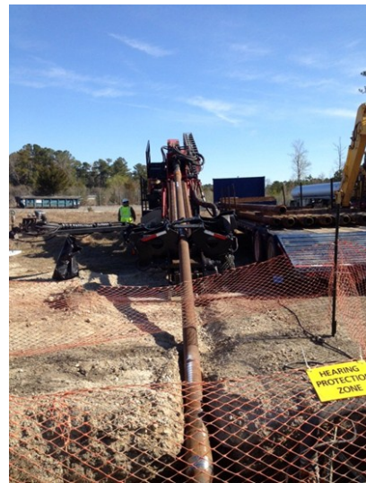
Air sparging, a passive, sustainable, and on-site remedy was selected to treat a dense liquid source area. This permanent solution can be reactivated as needed, at significantly less cost, to ensure future protectiveness.
