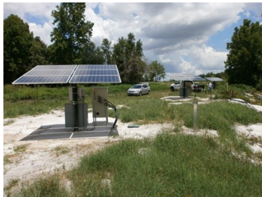
Solar-powered air sparging (removal of contaminant vapors) was selected for a pilot study to act as a sustainable solution for preventing groundwater contamination from discharging into the nearby creek.
