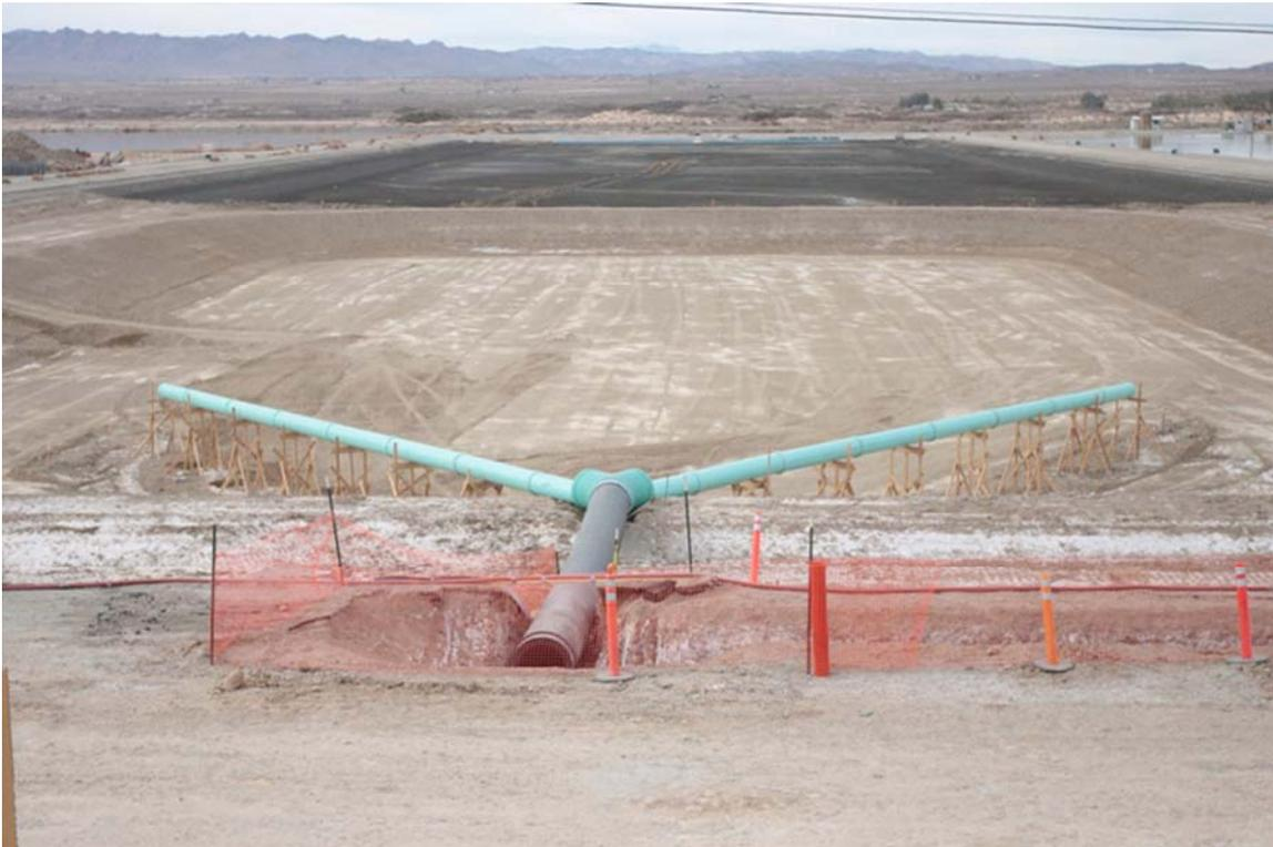
Construction site of the future Mainside Wastewater Treatment Facility at MCAGCC. This facility will utilize a biological treatment and be the first facility in the Marine Corps treating and reusing wastewater for irrigation.
