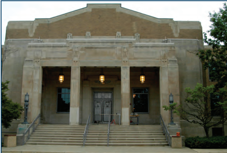
Exterior view of Building 12's main entrance. This building is the most elaborate example of art deco design at Wright-Patterson AFB. The building was rehabilitated for BRAC realignment and became a prime example of adaptive reuse of historic structures. It won the Merit Award from the Ohio State Historic Preservation Office in 2010.
