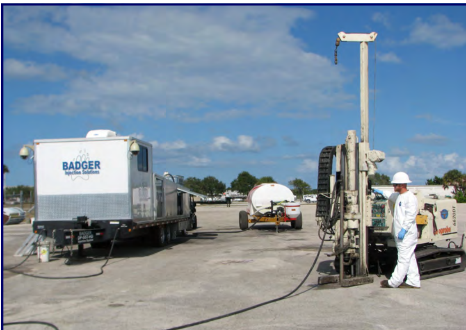
EZVI and EVO injections at Hangar K, Sept 2010.
