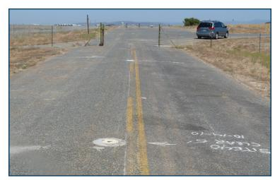
Hidden under five flush mount well caps are Emulsified Vegetable Oil injection points forming a biobarrier in a TCE contaminated plume at approximately 150 feet below ground surface. By 2013 the biobarrier has proven to be effective in cutting off the groundwater plume and preventing further migration into the runway security zone. A picket line of biobarrier injection wells can cut a contaminated groundwater plume in half shortening its life.
