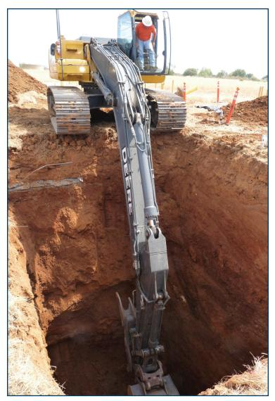
Bioreactor excavation on ERP Site 13 landfill featured during a RAB tour before being back filled with ordinary garden mulch, gravel, vegetable oil and molasses. The bioreactor was enlarged in 2012 and connected to a well which pumped groundwater to the top of the bioreactor. Pumped groundwater percolates through the mixture and carries organic material into the surrounding groundwater.
