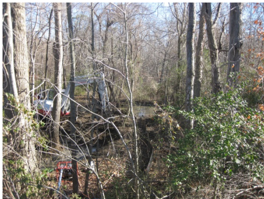
Figure 6: Precision Excavation Within Operable Unit 13
