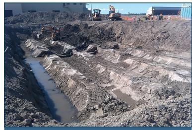
Removal projects performed at two former underground storage tank sites. These projects were strategically executed during a runway replacement project, and resulted in no mission impacts. The removal actions resulted in the removal of 12,000 tons of contaminated soil and concrete, and the treatment of 310,300 gallons of contaminated groundwater.
