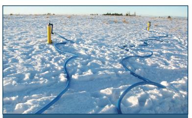
Dual-purpose remediation wells are connected to the soil vapor extraction system. Soil vapor extraction has been implemented in conjunction with in-situ chemical oxidation injections, and batch operations at the existing groundwater extraction and treatment system. The triad of remedies implemented has optimized chlorinated solvent removal and degradation at Craig Road Landfill.
