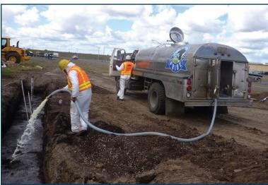
Cheese whey being applied during the construction of the sustainable bioreactor demonstration project. Fairchild AFB worked cooperatively with a local creamery to enable the reuse of cheese whey, a bi-product from creamery processes. The cheese whey served as a necessary carbon source within the construction of the solar-operated bioreactor and promotes the breakdown of contaminants in groundwater using natural processes.
