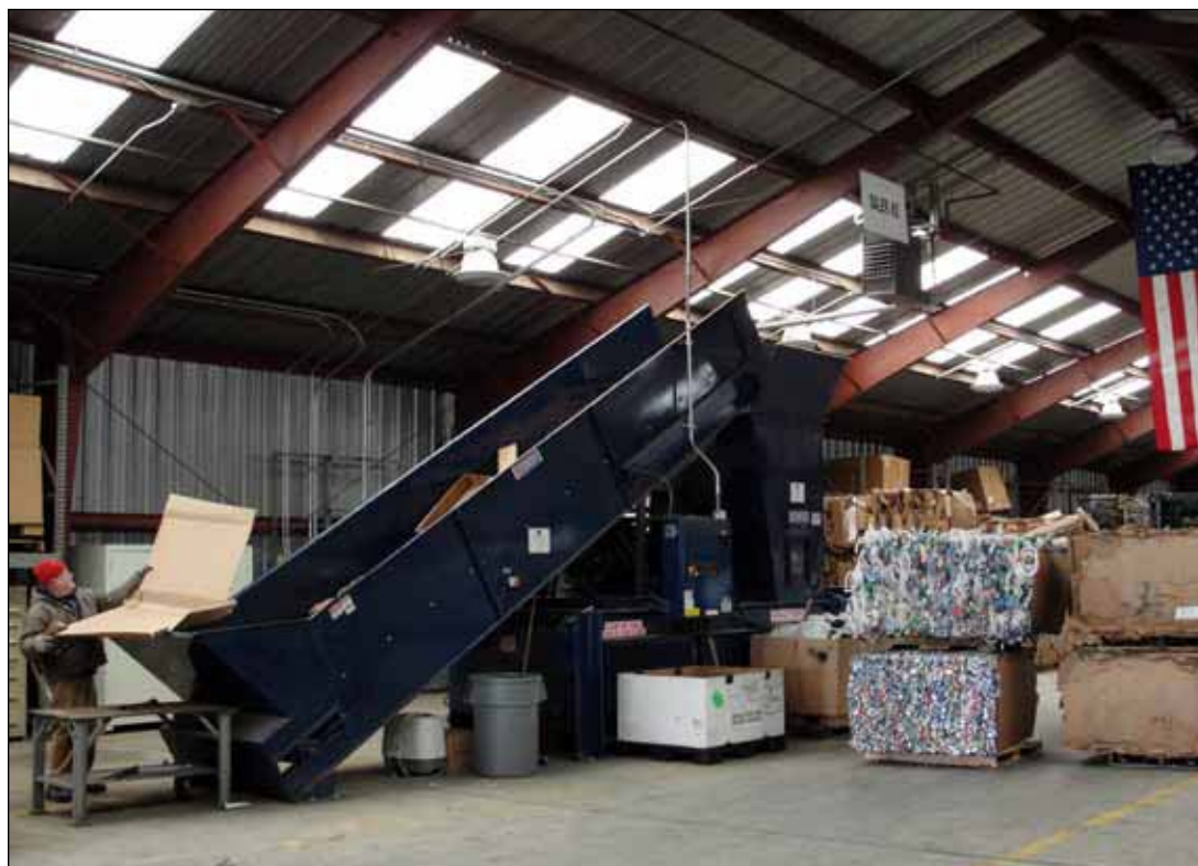
As part of LEAD's Qualified Recycling Program, employees use equipment on site to compact material.
